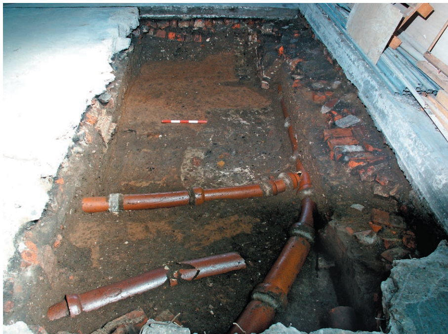
Plate 2 Trench 2 looking north after initial clean, showing natural subsoil 2032 in background, unexcavated features 2016 and 2044 in mid ground and modern drains in foreground
