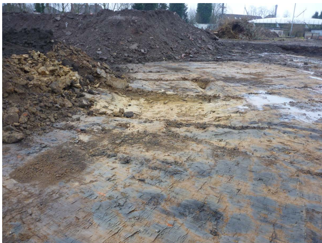
Plate 2 Eastern side of S4, showing Natural 10010 after hotspot removal
