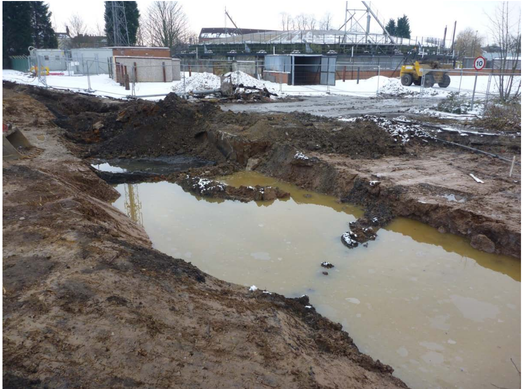
Plate 7 Excavated construction cut 11007 for tank 11006, looking south
