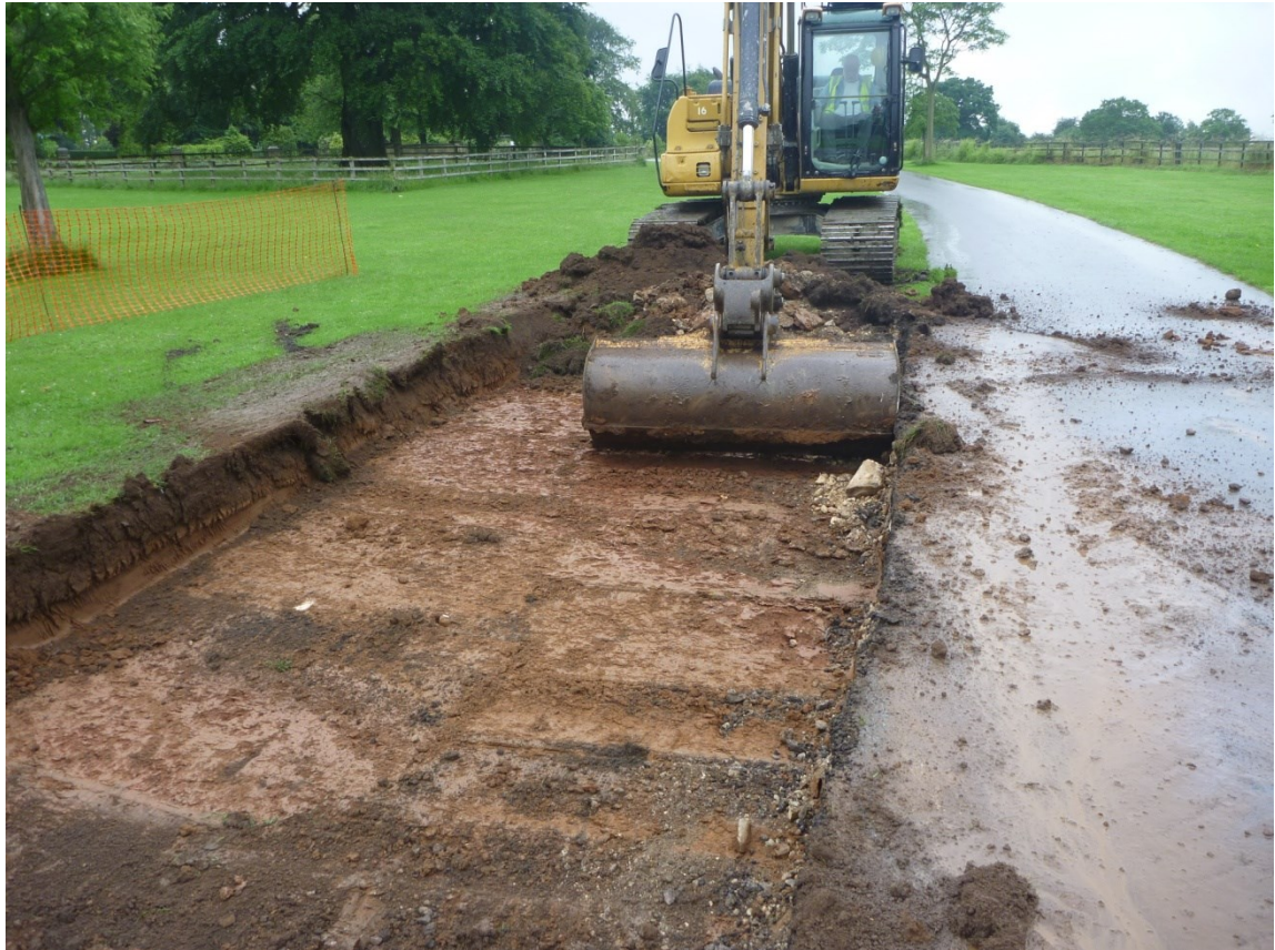
Plate 27 Machining of road widening trench in progress, looking SE
