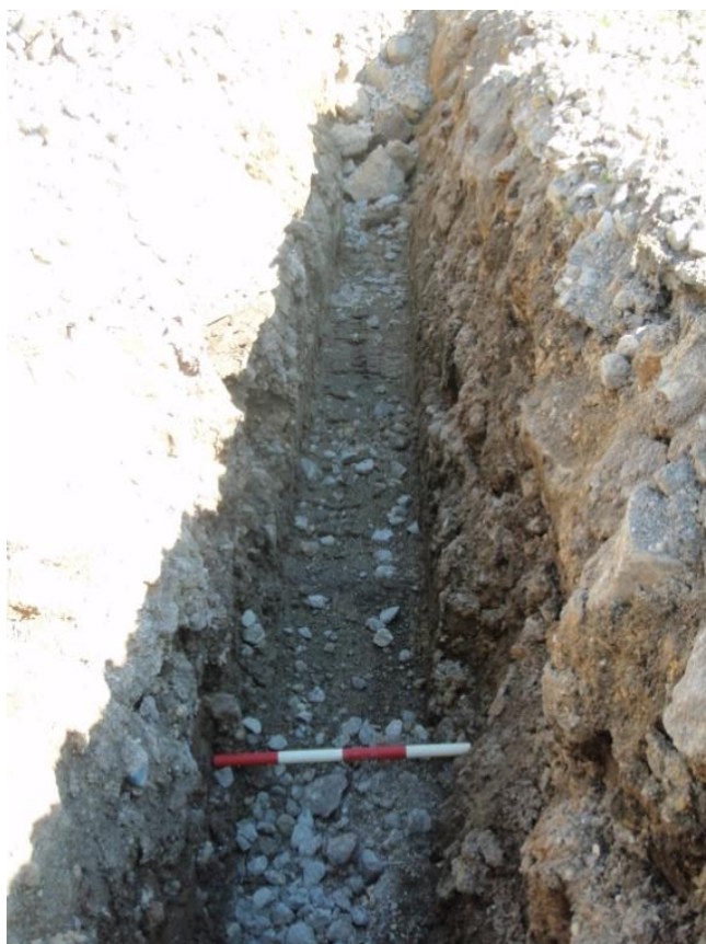
Plate 2 View along the excavated services trench facing north-north-west scale unit 0.1m.
