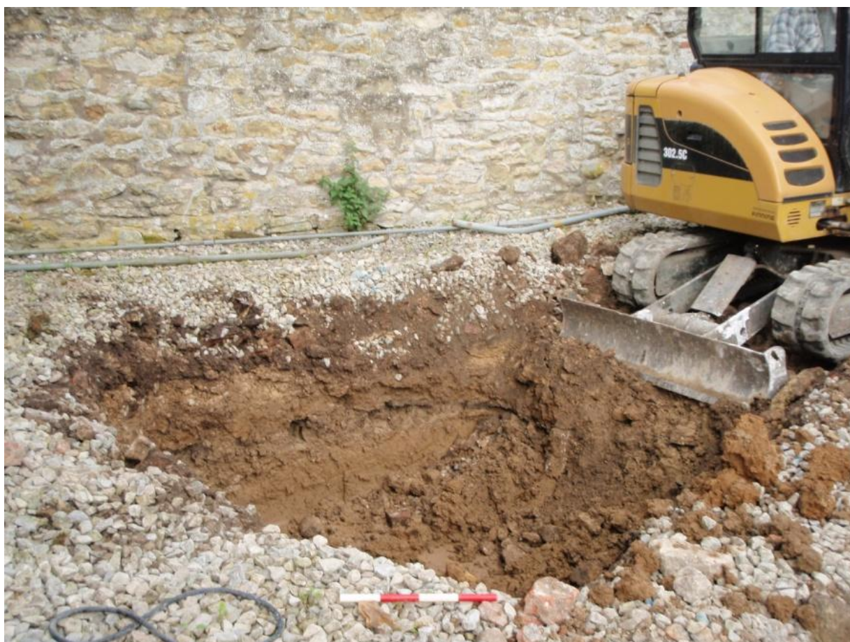
Plate 11 Excavation of the septic tank pit, facing north-west, scale unit 0.1m.
