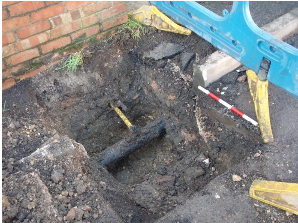
Plate 7 Trench 6 facing west, scale unit 0.1m.
