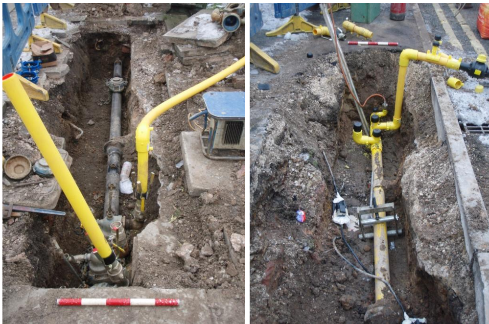
Plate 35 Trench 28 facing west and east, scale unit 0.1m.
