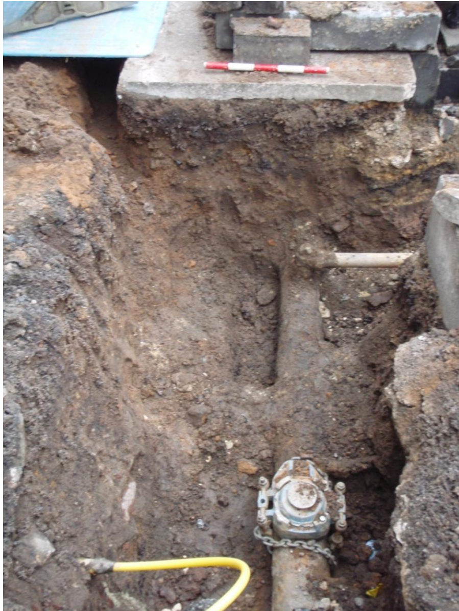
Plate 24 Trench 21 facing north-west, scale unit 0.1m.
