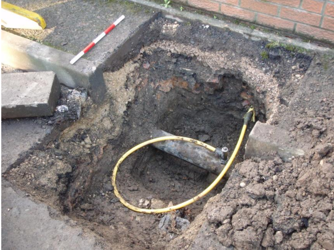
Plate 9 Trench 8 facing south-south-west, scale unit 0.1m
