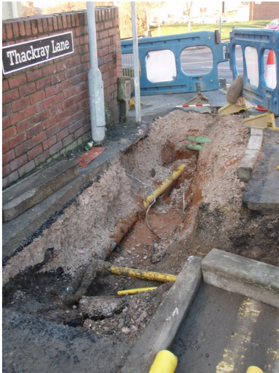
Plate 11 Trench 10 facing west, scale unit 0.1m
