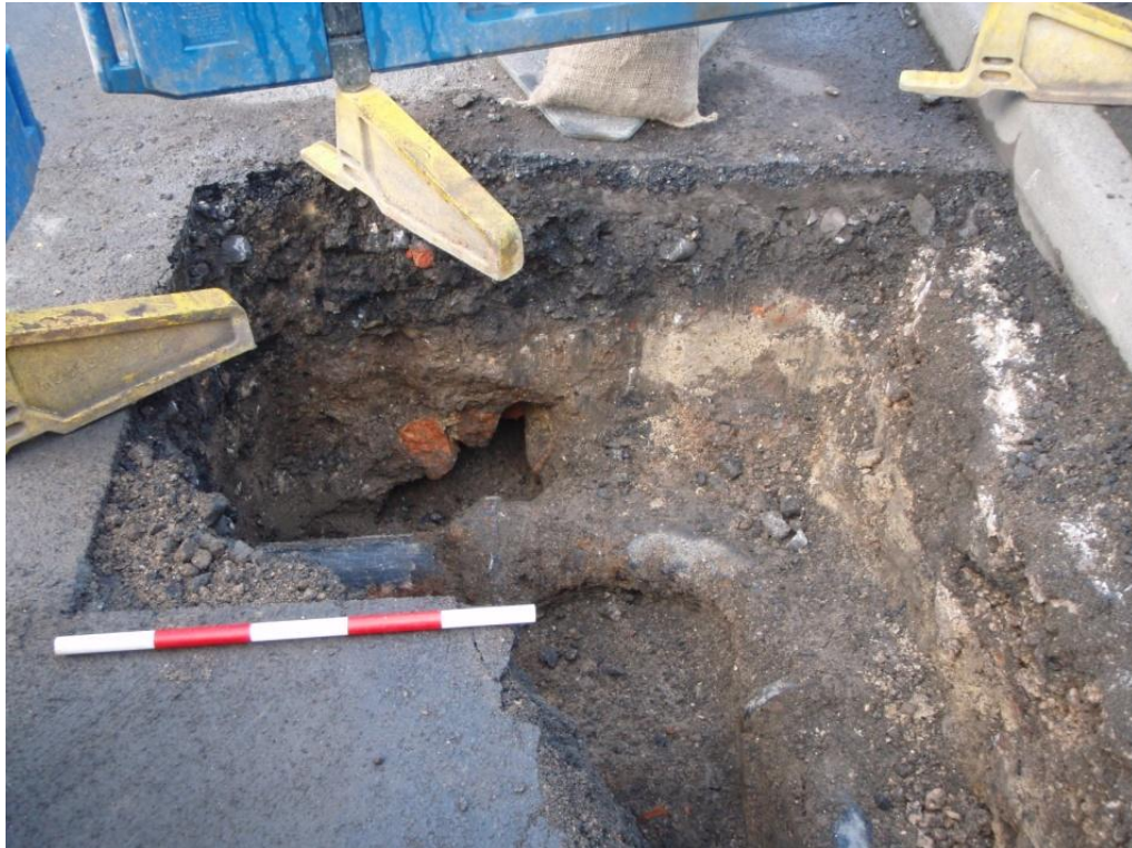
Plate 10 Trench 9 facing north-west, scale unit 0.1m
