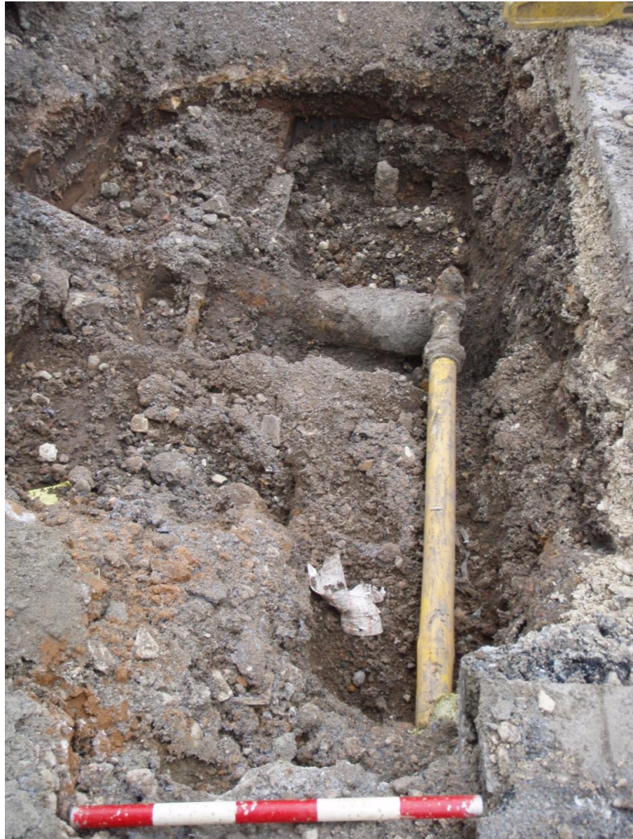
Plate 20 Trench 18 facing north-west, scale unit 0.1m.
