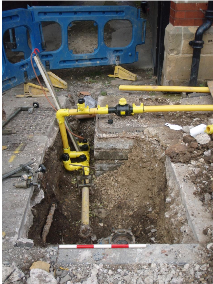
Plate 44 Trench 34, facing north-west, scale unit 0.1m.
