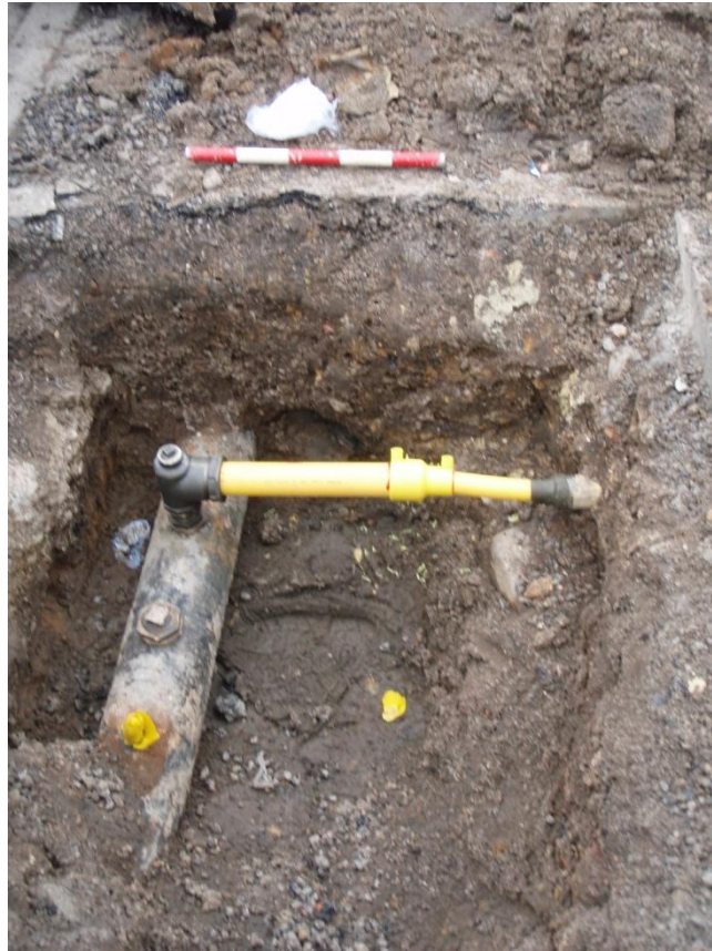
Plate 31 Trench 26 facing west, scale unit 0.1m.
