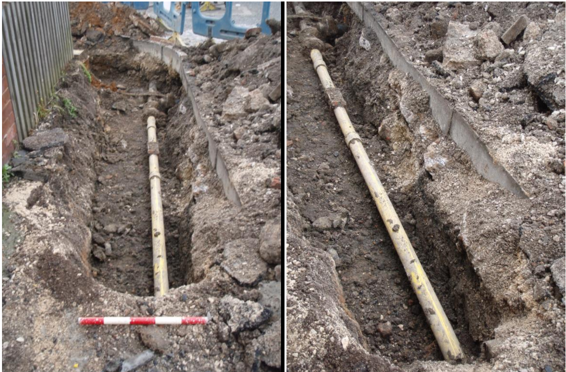
Plate 33 Trench 27 facing south and south-west, scale unit 0.1m.
