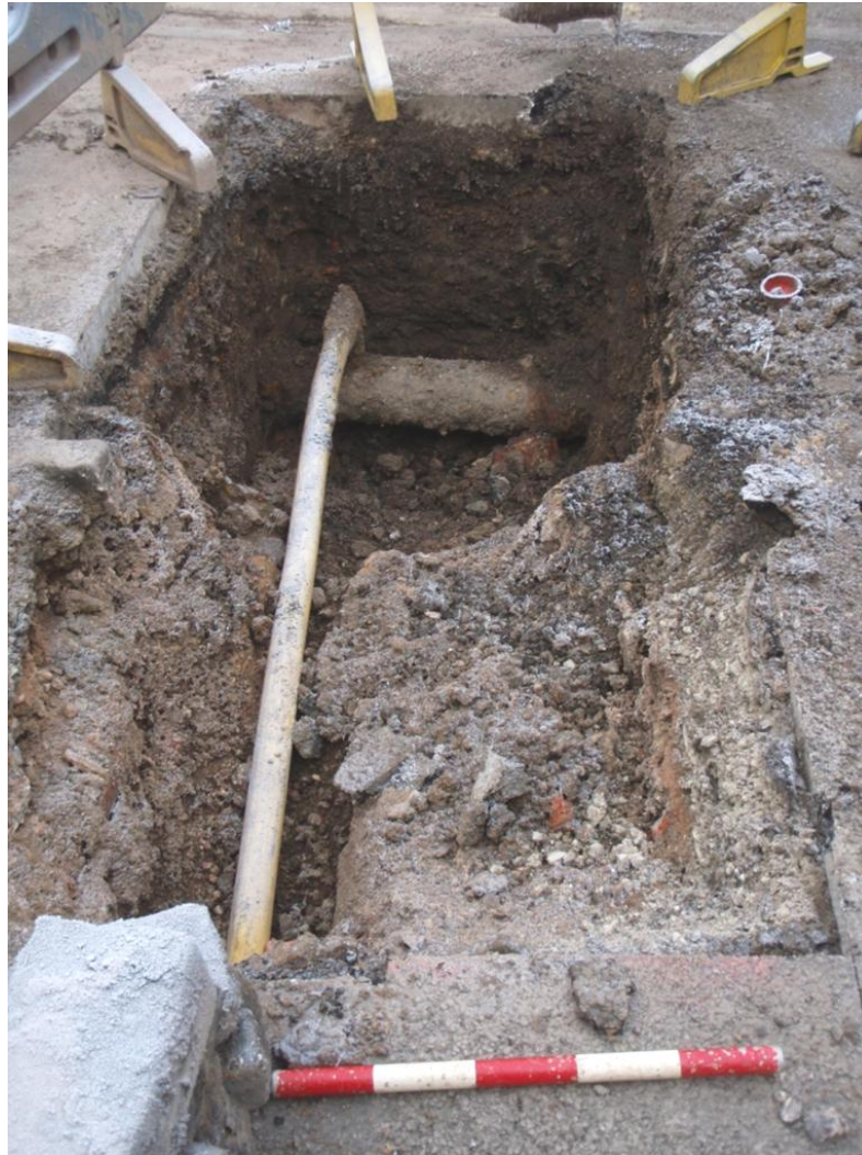
Plate 18 Trench 16 facing north-west, scale unit 0.1m.
