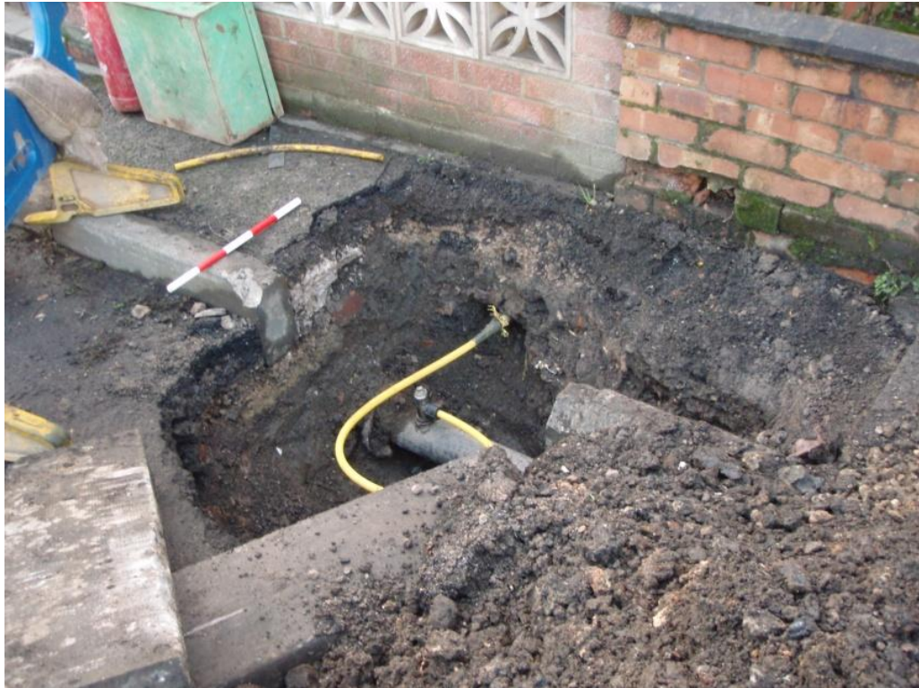
Plate 8 Trench 7 facing south-south-west, scale unit 0.1m.
