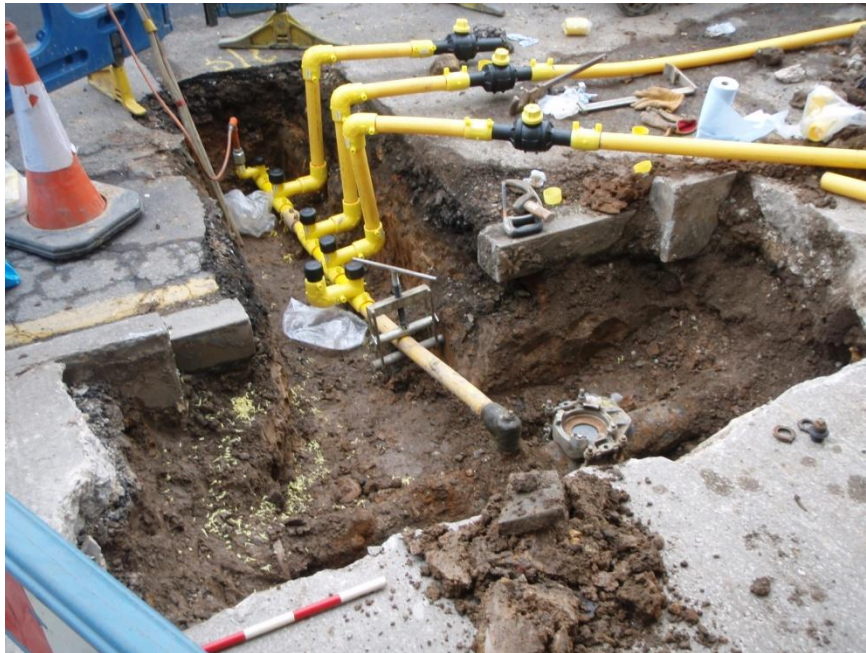
Plate 45 Trench 35, facing north-west, scale unit 0.1m.
