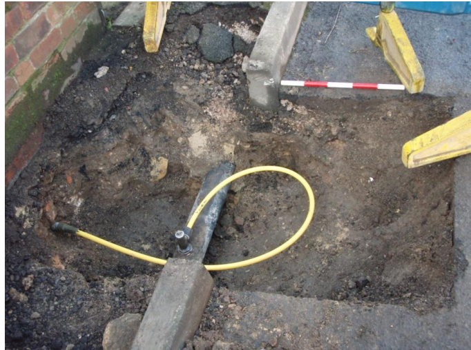
Plate 5 Trench 4 facing north-west, scale unit 0.1m.
