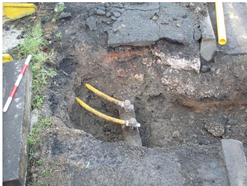
Plate 2 Trench 1 facing north-west, scale unit 0.1m.
