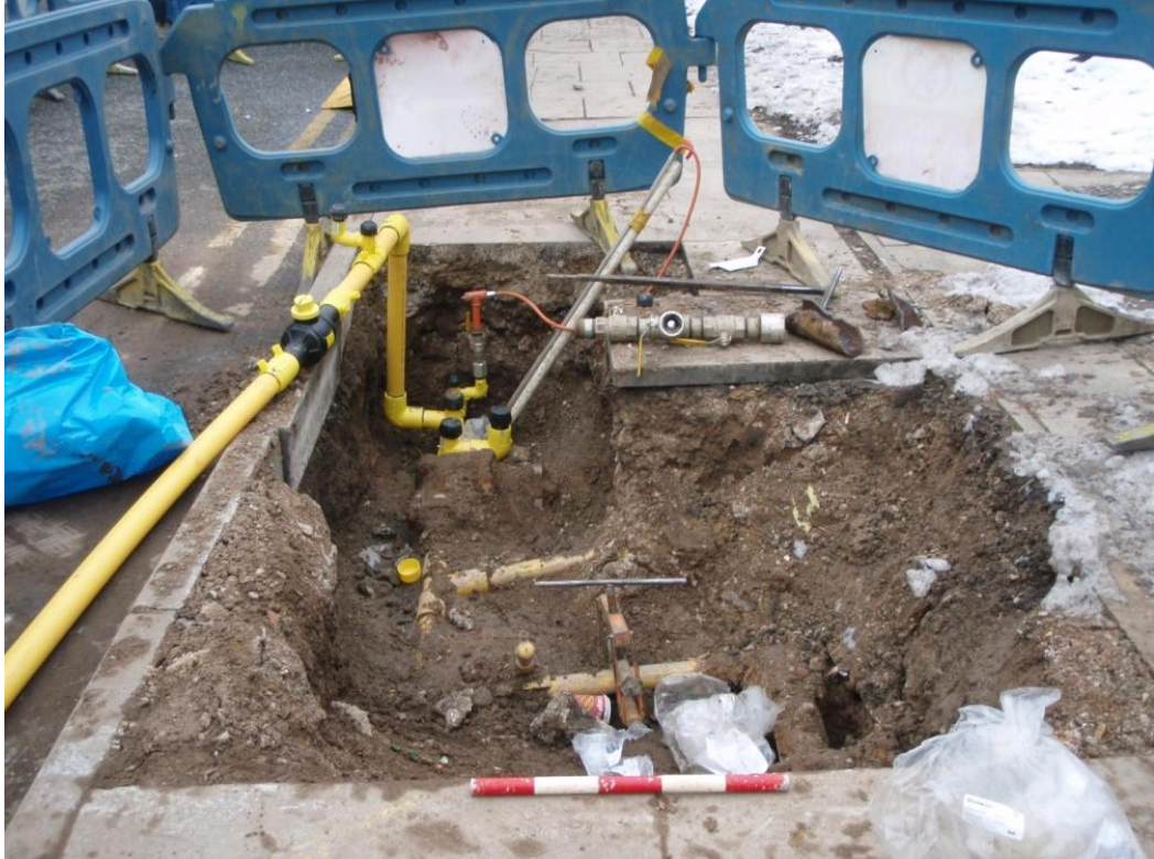
Plate 40 Trench 31 facing west, scale unit 0.1m.
