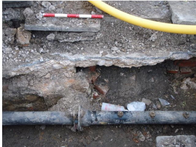
Plate 34 Eastern end of Trench 28 facing north, showing the sandstone truncated by a modern brick feature, scale unit 0.1m.
