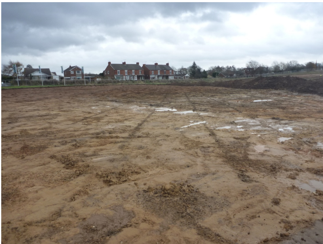
Plate 4. The north-eastern stripped area showing natural yellow clay in the foreground and natural fractured sandstone in the distance, with modern stone filled field drains showing as parallel lines, facing south-east
