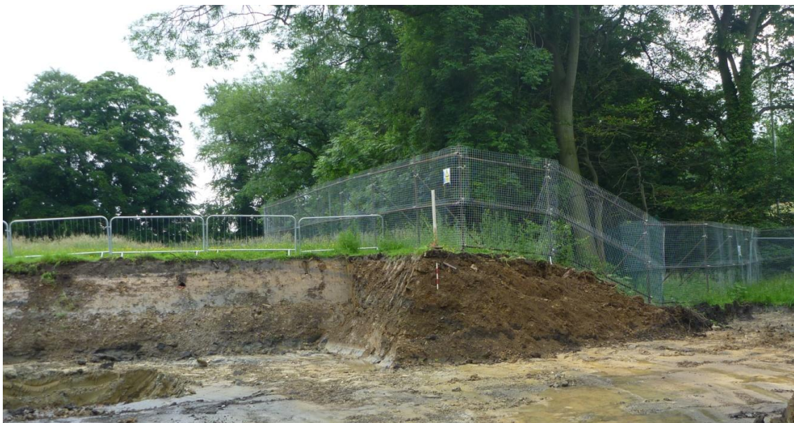
Plate 4 SE corner area of new car park as machined to formation level. A relict soil, 103, can be seen within the section and one or two tip-lines in the re-deposited material, 102, above this. Looking ESE. 0.10m scale divisions.
