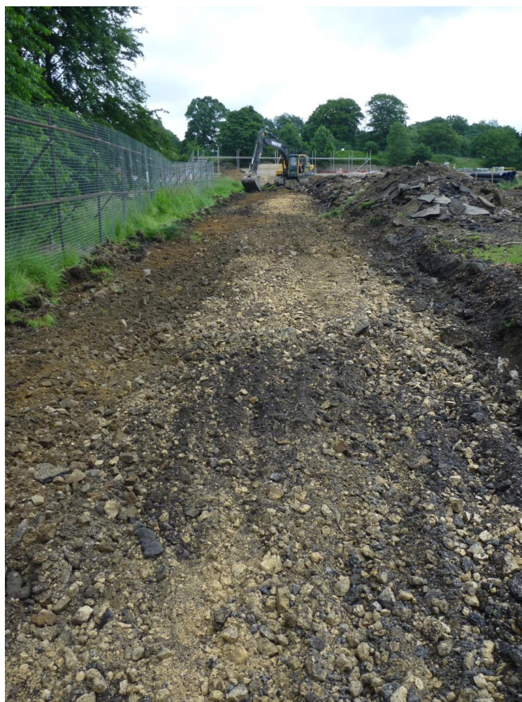
Plate 7 Stripping of the existing road adjacent to the new car park area, looking N
