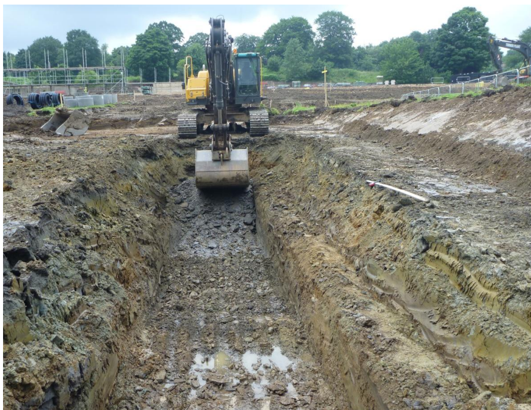
Plate 6 Excavation for the attenuation tank below the car park, looking N.
