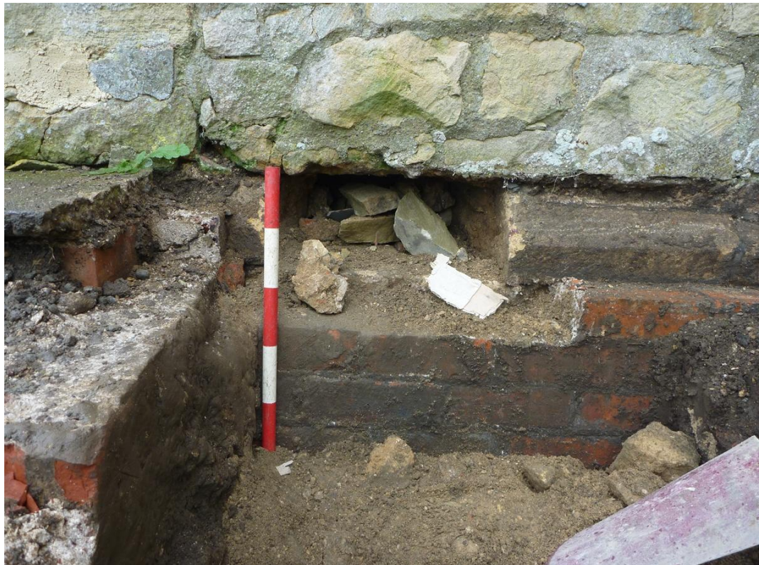
Plate 15 Aisle wall foundation after removal of plinth stone
