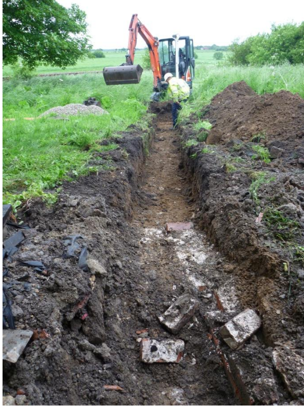
Plate 16 Foul water trench, looking WNW, showing remains of cellar 1010
