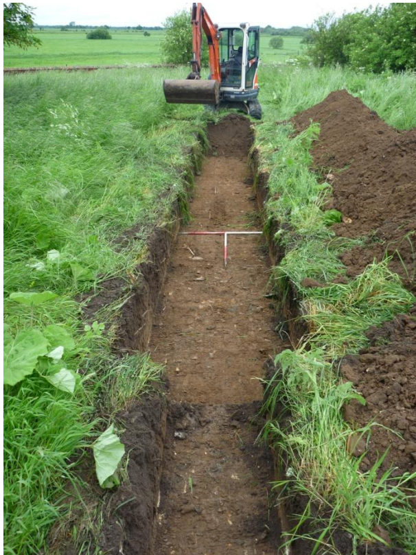
Plate 17 Soak-away trench, looking WNW
