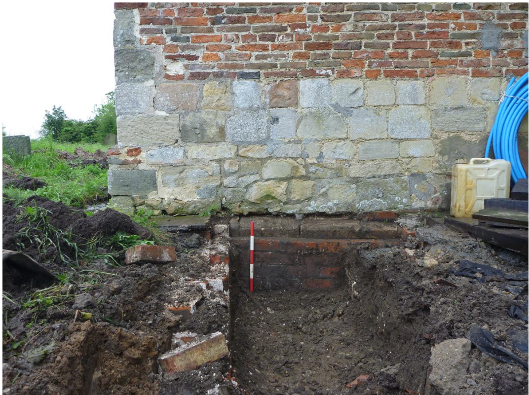
Plate 13 West facing elevation of the north aisle wall and foundation
