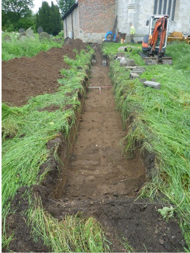
Plate 18 Soak-away trench, looking ESE
