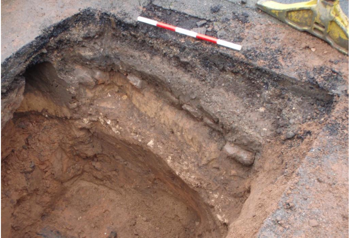
Plate 2 Metalled surface of cobbles set on a bedding of sand in Trench 25. The position of the kerbing (removed) can be seen in the void to the upper left. The stoney layer below this represents an earlier surface, with accumulation above. Looking NE
