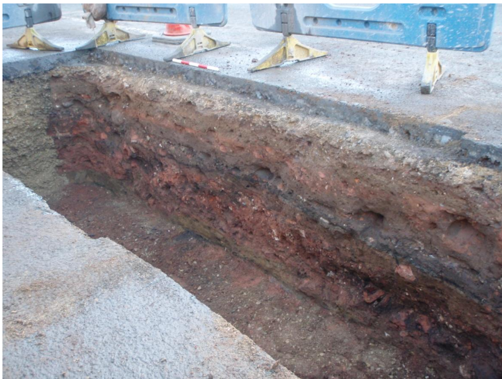
Plate 28 Mixture of rubble and soft deposits in the eastern part of Trench 56, Looking SE
