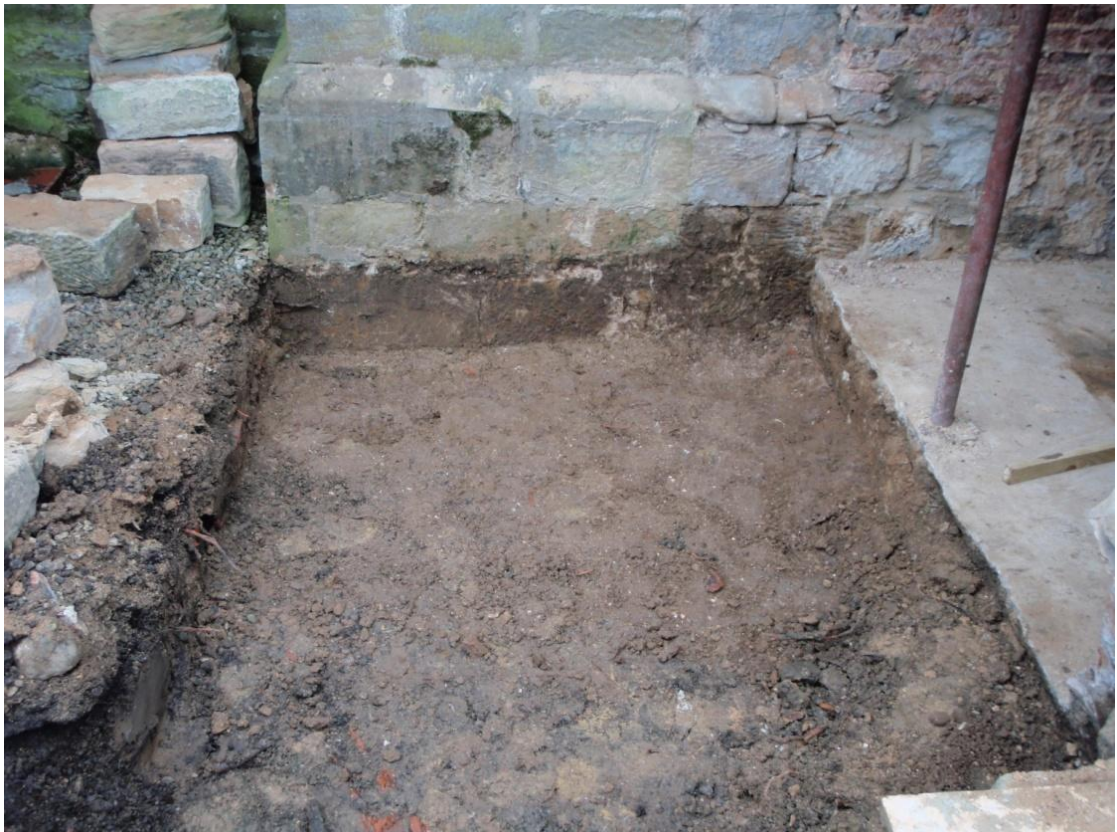
Plate 6 View of reduced area of ?natural ground in the area of extension to the store, Looking S. Note the dirtier appearance of that part in the foreground which is owed to the presence of tree roots, land drain and other disturbance.
