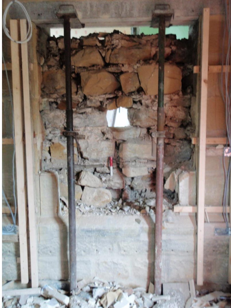
Plate 5 View of internal part of wall in area of new doorway to the library. Looking N.
