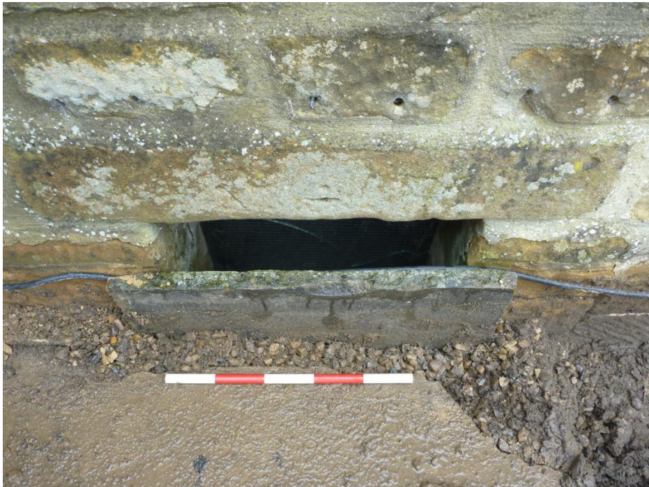
Plate 4 View of west basement window (to be blocked-up).
