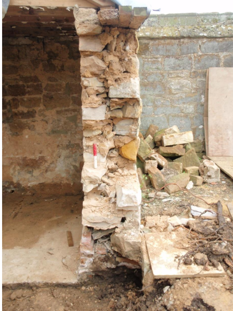
Plate 8 Cross section of store walling after removal of the east wall. Looking W.
