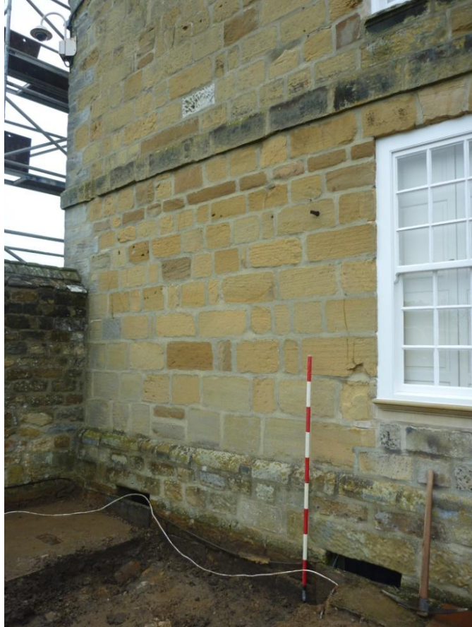
Plate 3 View of area of drawn walling, note the two basement windows.
