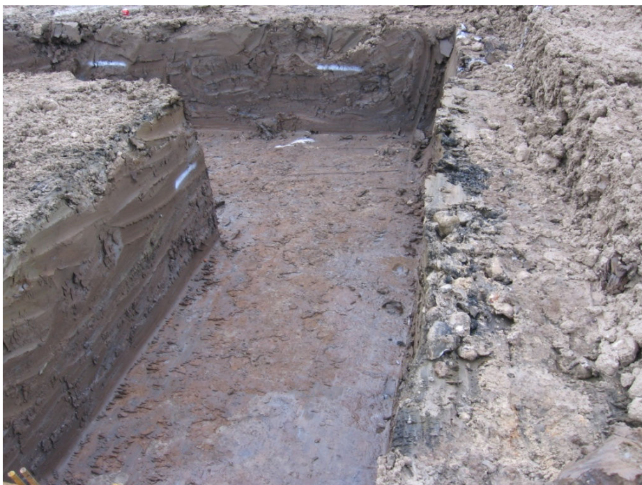
Plate 6 Foundation trenches in northern part of site showing modern materials directly over natural deposits, looking N.
