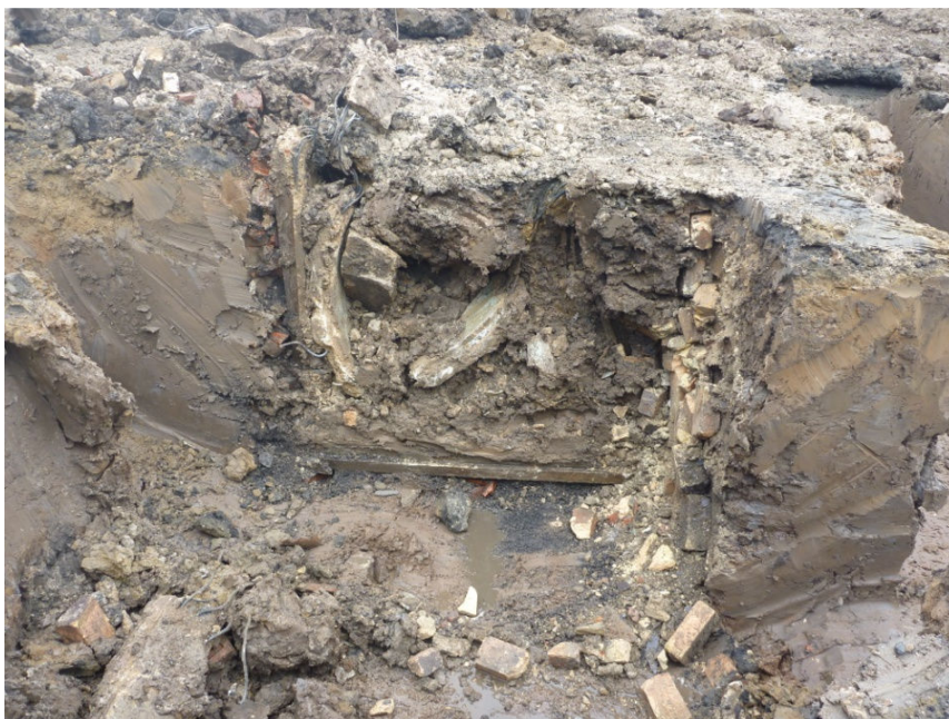
Plate 4 Walls and base of Shelter 6. Note rubble fill in narrow gap between trench cut and wall, also curved roof panels within backfill, looking N.
