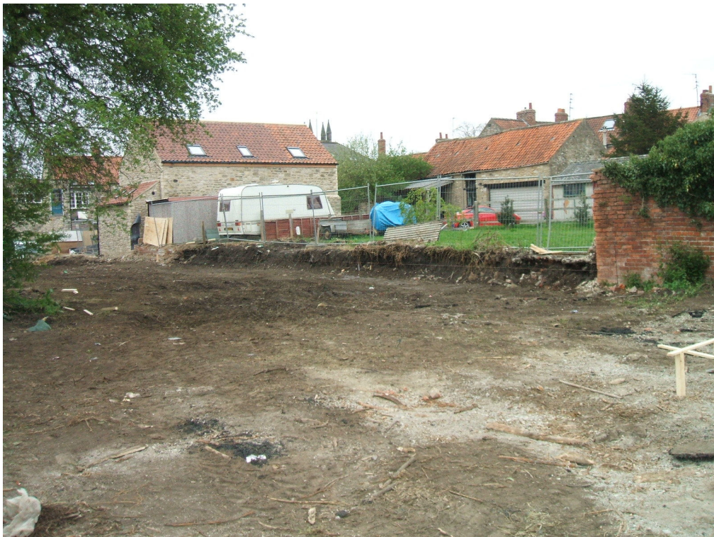
Plate 1 Site after vegetation/partial topsoil strip, looking W
