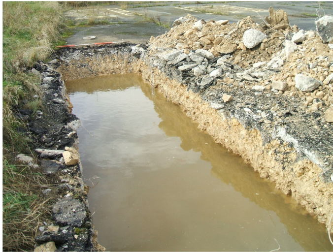
Plate 7 Groundwater in western end of Trench 7/8, looking NW
