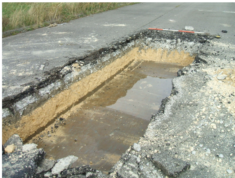
Plate 14 Trench 14, looking NE
