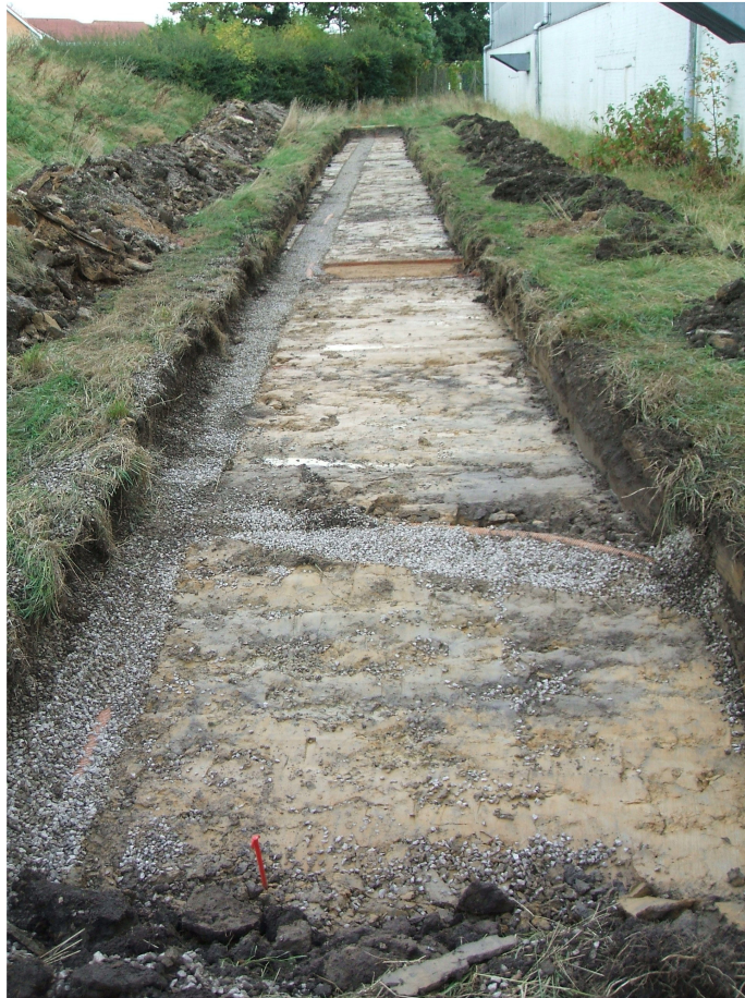
Plate 15 Trench 15, looking SE
