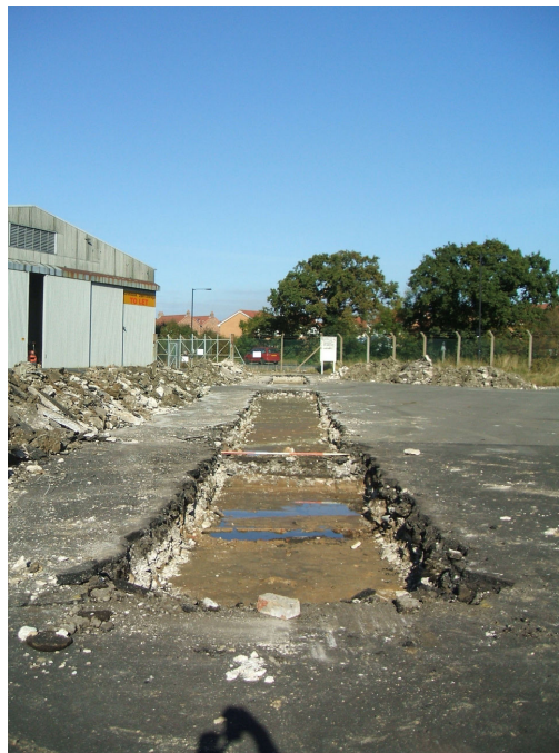
Plate 3 Trench 3, looking NNE
