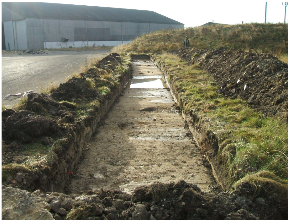
Plate 11 Trench 11, looking SE
