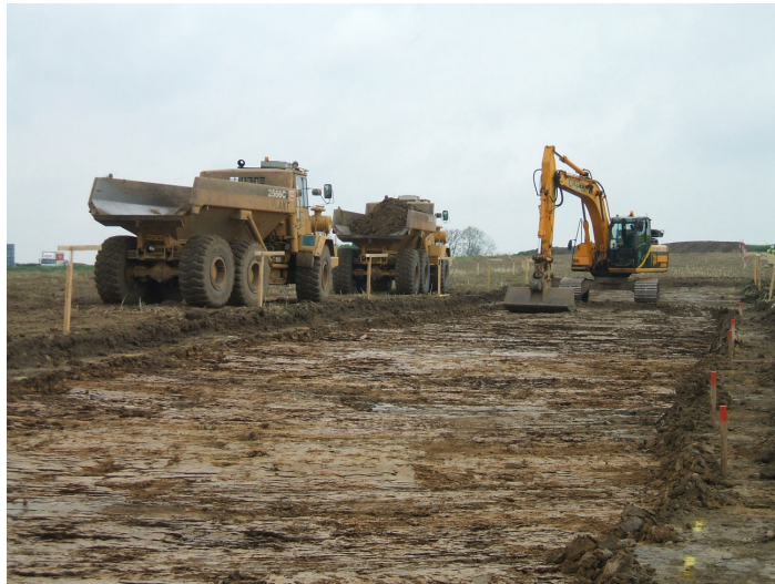
Plate 7 1stage watching brief, stripping, looking N
