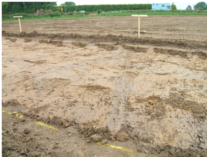
Plate 8 First stage watching brief, some of features revealed, looking W
