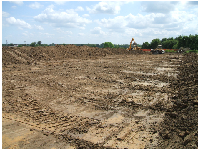
Plate 9 Second stage watching brief, process, looking S
