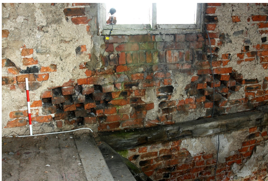
Plate 7 Blocked vents to E side of N wall below inserted window and adjacent to steps, note render to walls, looking NNE
