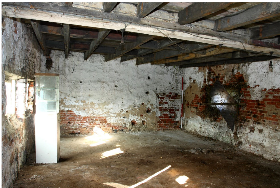
Plate 4 Barn ground floor, western space, looking WNW. Note blocked doorway near corner
