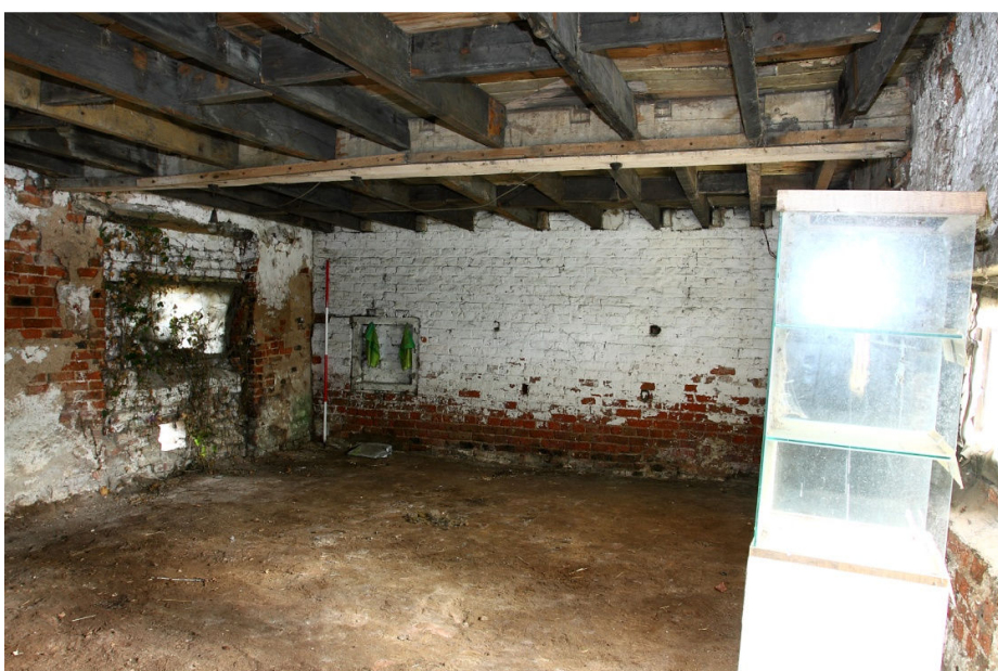
Plate 3 Barn ground floor, western space, looking ENE. Note blocked N doorway, slots in beam for coggled joists and inserted 19 th century wall with small blocked opening
