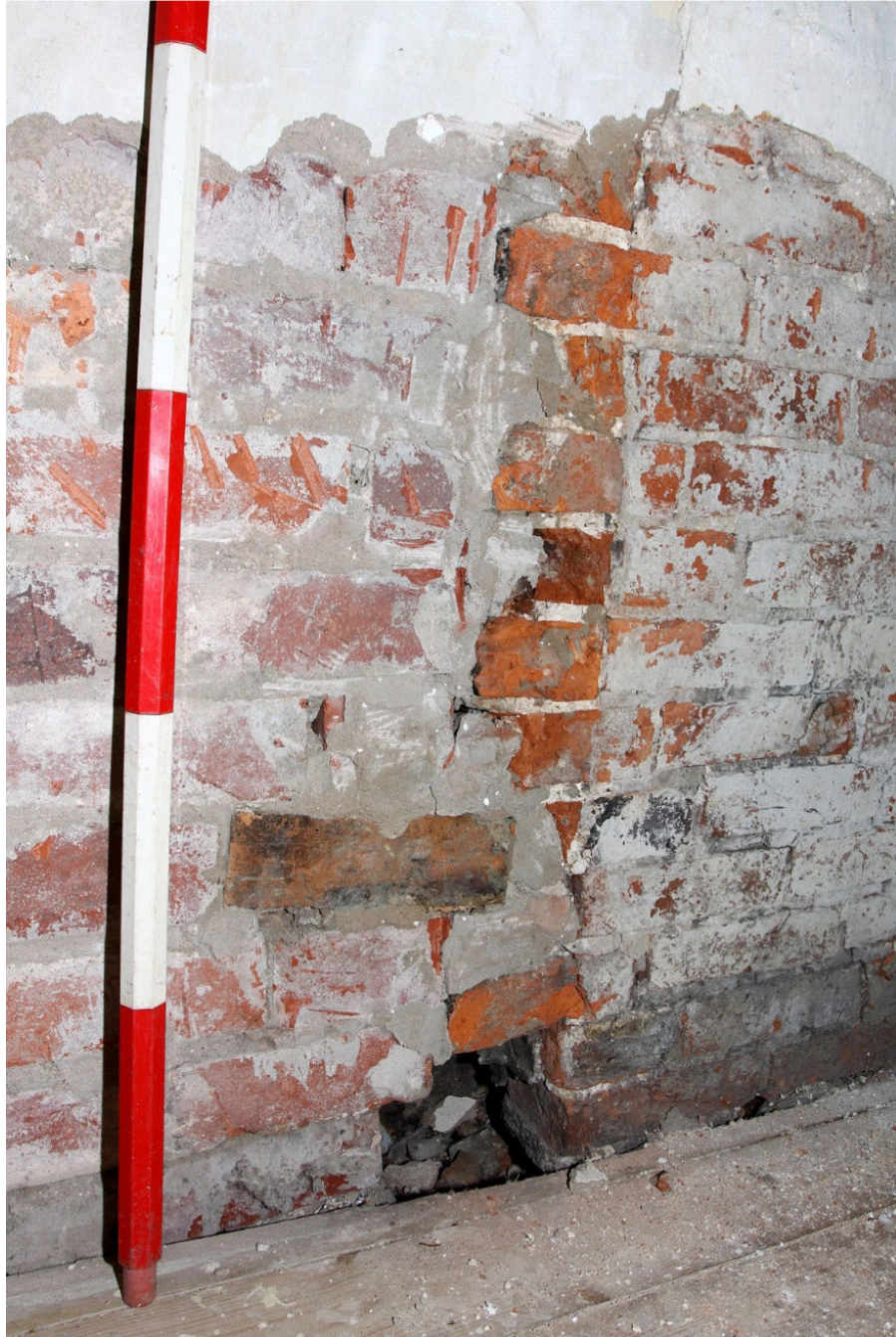
Plate 32 Blocking of former fireplace in first floor passage, looking SE
