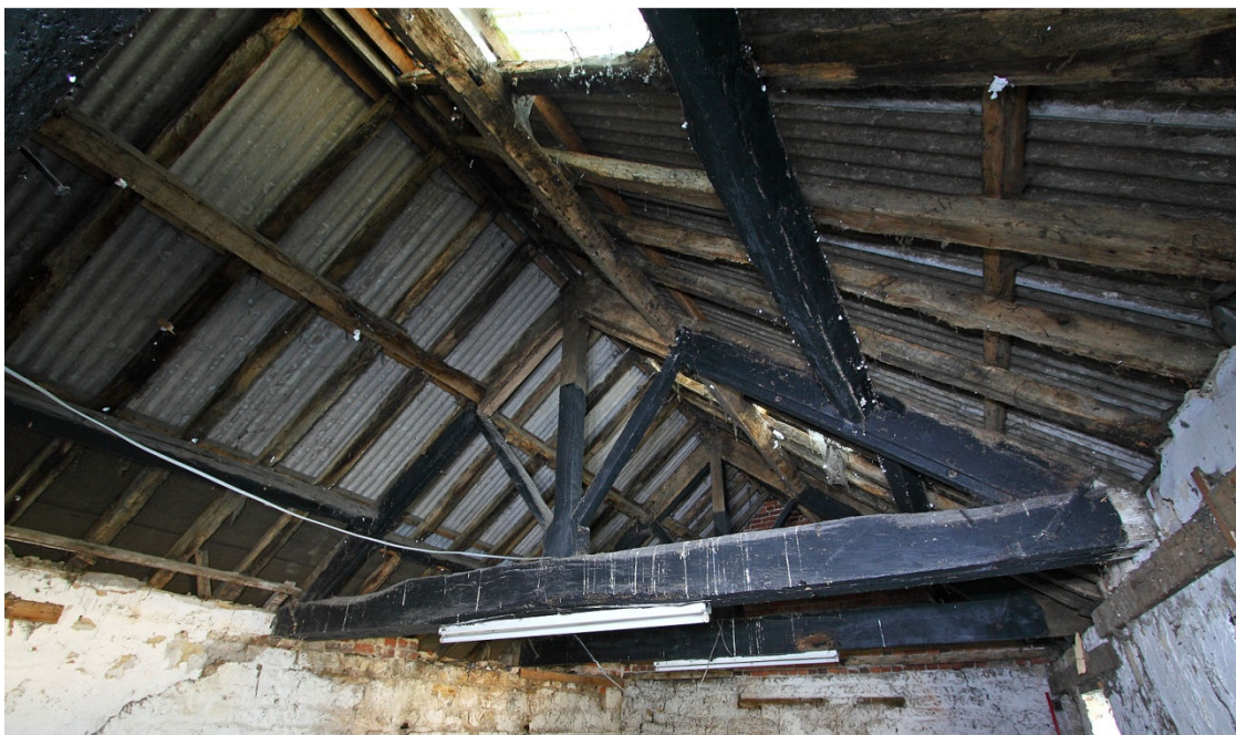
Plate 11 Painted roof truss of original building of south range, looking W
