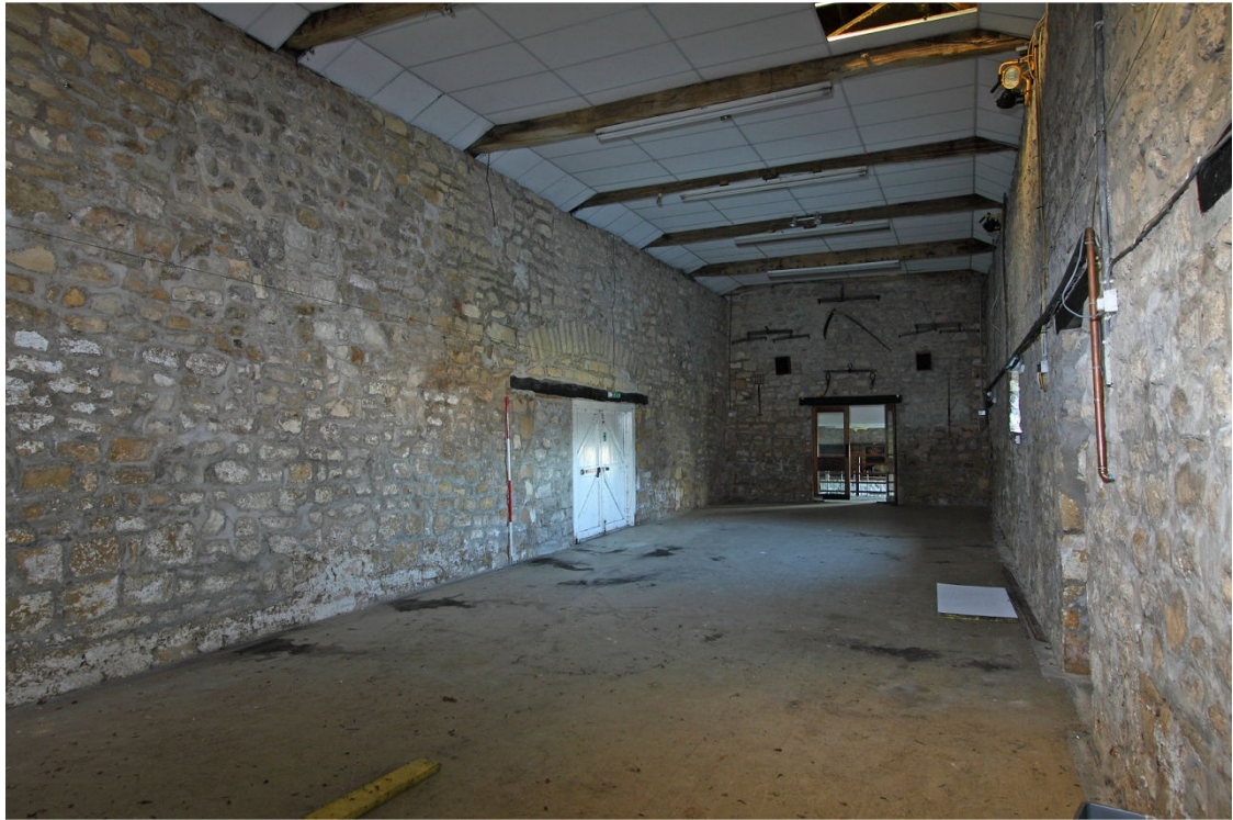
Plate 3 Interior of barn, looking N
