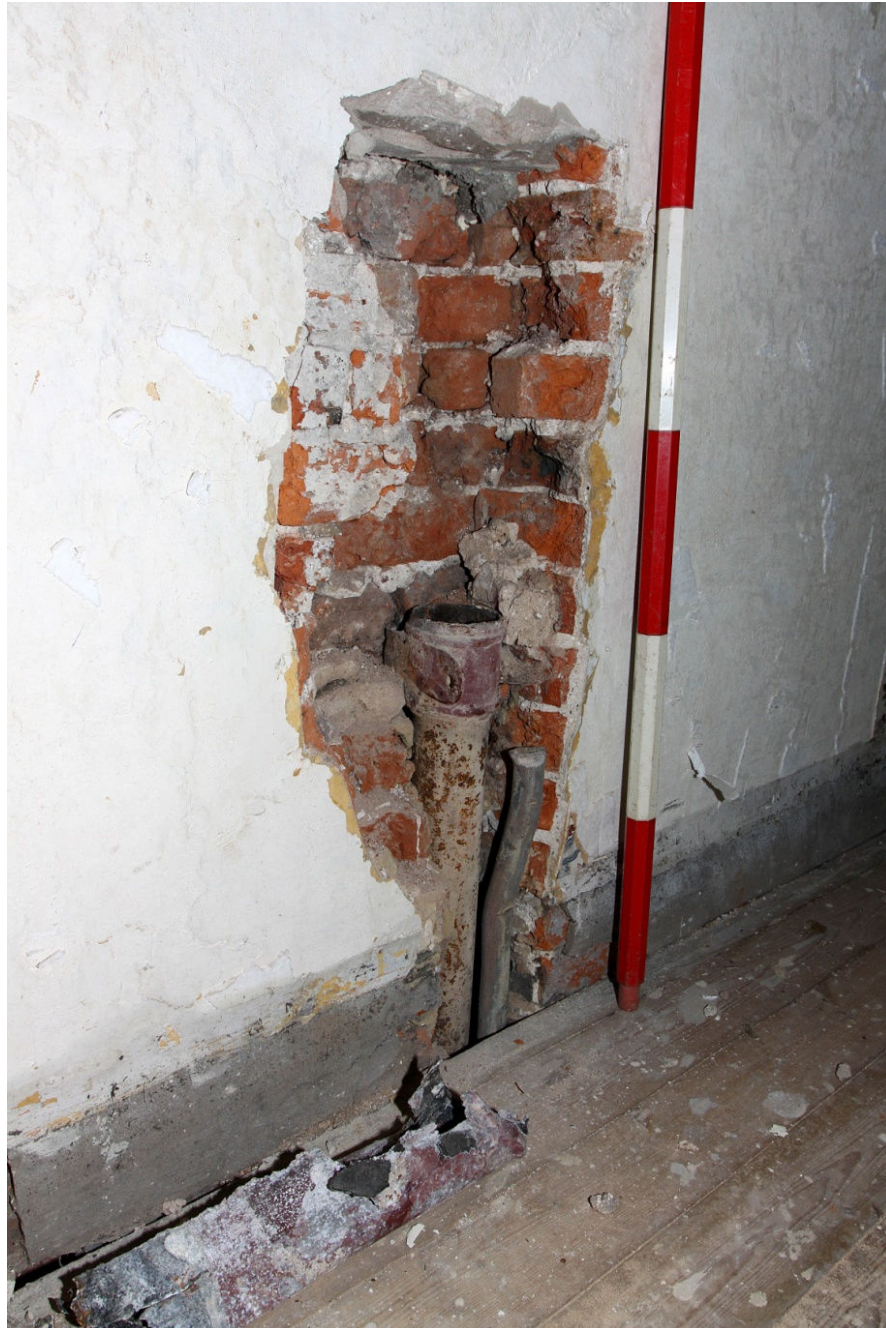
Plate 33 Pipe-work chased into wall in first floor passage, looking SE
