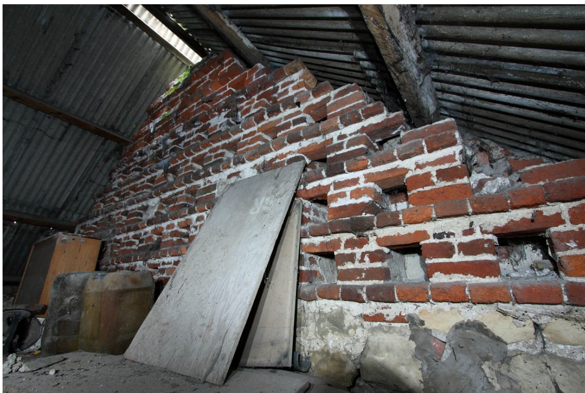
Plate 16 Nesting boxes of dovecote in west gable wall, looking SW
