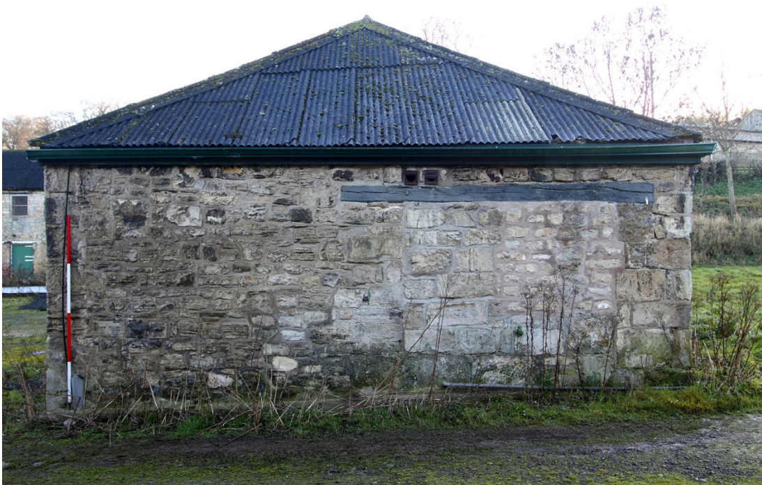
Plate 4 North end of extension to west range, looking S
