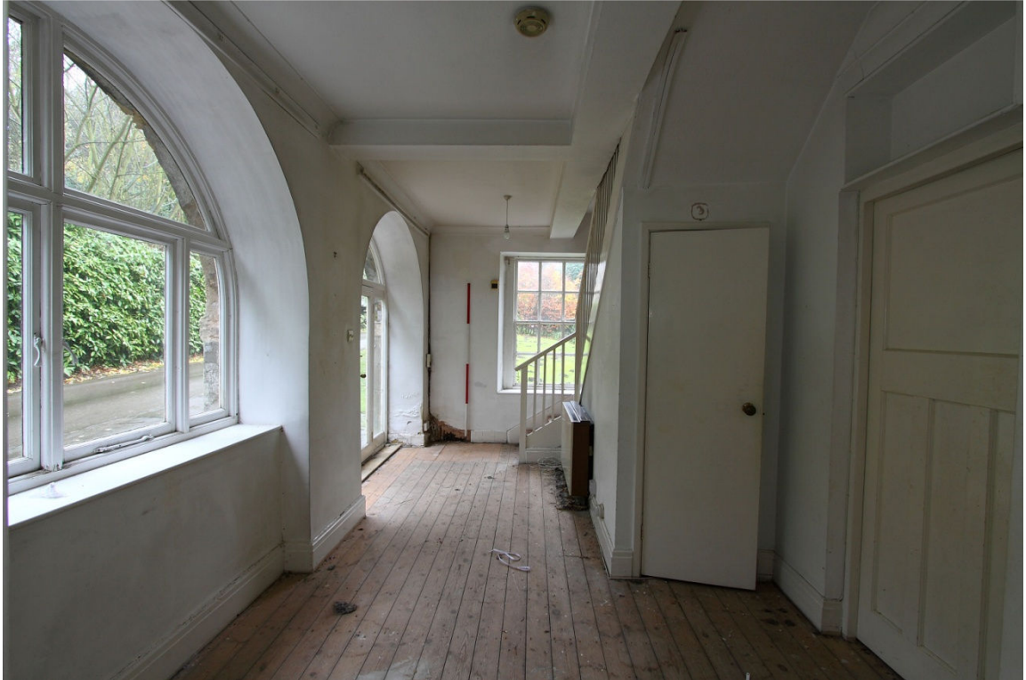
Plate 22 Brewhouse hallway, looking W
