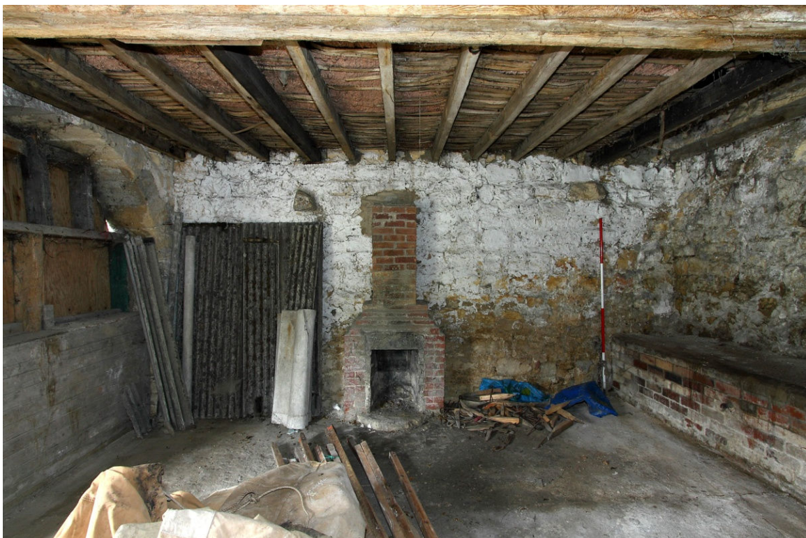
Plate 15 Interior of cart shed with inserted fireplace and plinth, looking W
