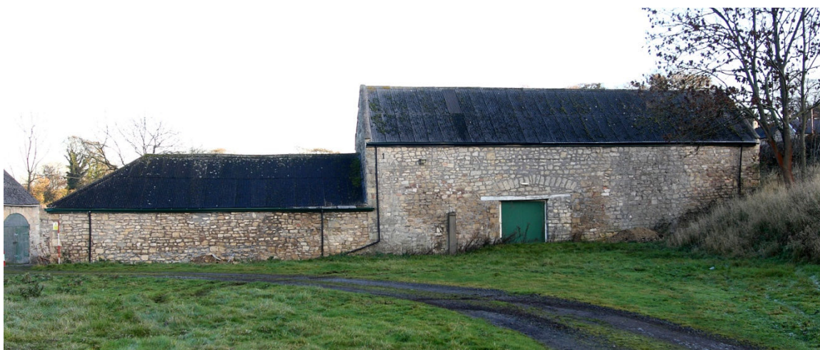
Plate 1 Barn and extension of west range, looking E
