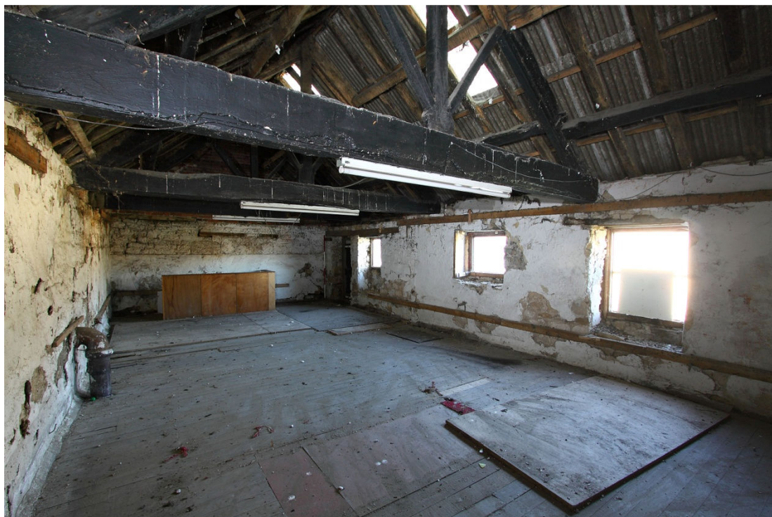
Plate 9 First floor of original building of south range, looking W
