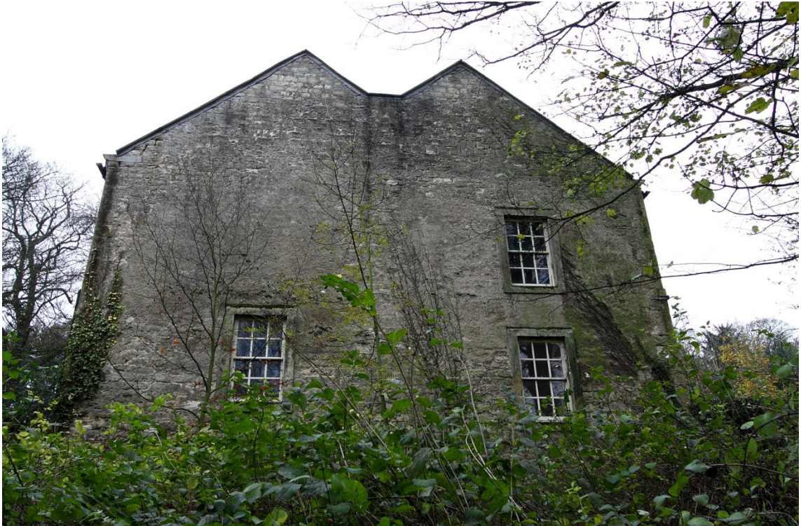
Plate 20 N elevation of Brewhouse, looking S
