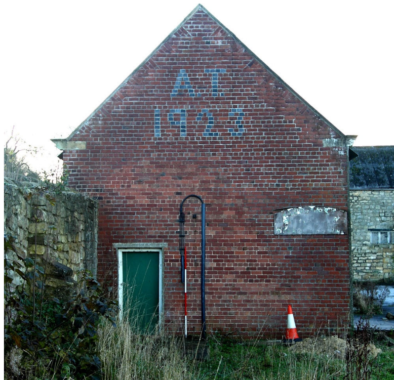
Plate 7 Rebuilt gable end of south range, note reuse of kneelers and coping, looking W
