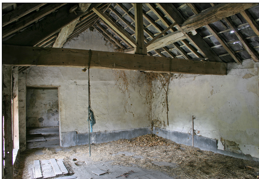
Plate 13 Building A2, central room first floor, facing west
