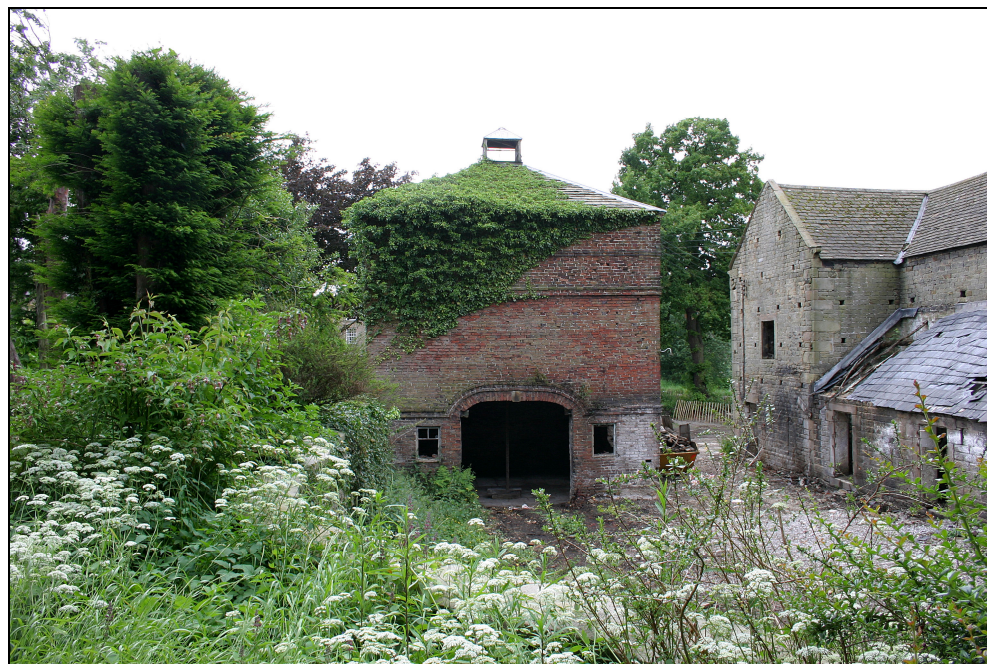
Plate 7 Building D, dovecote, east elevation
