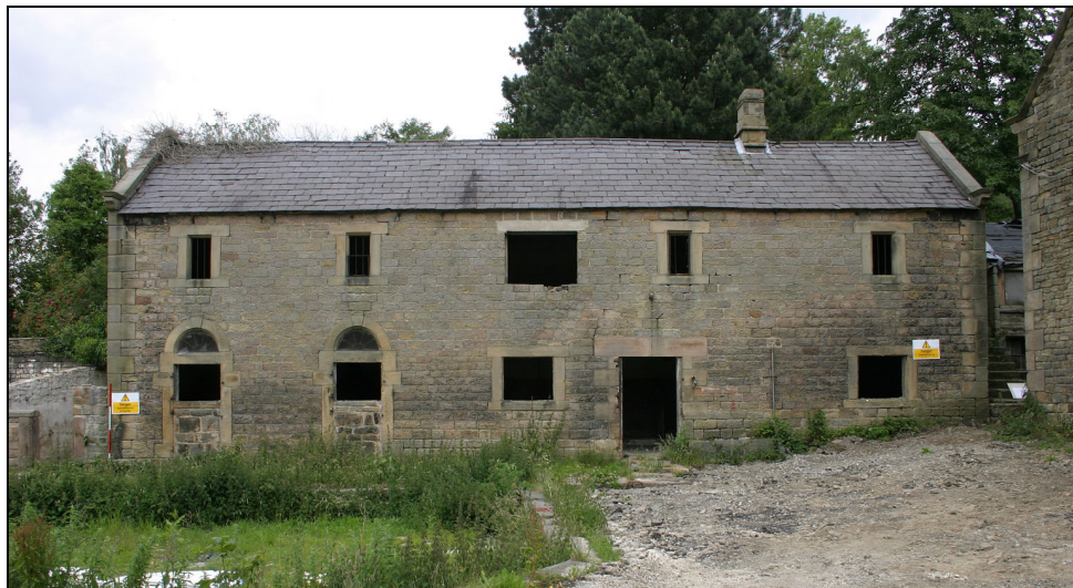
Plate 2 Building A2, stable block, south elevation
