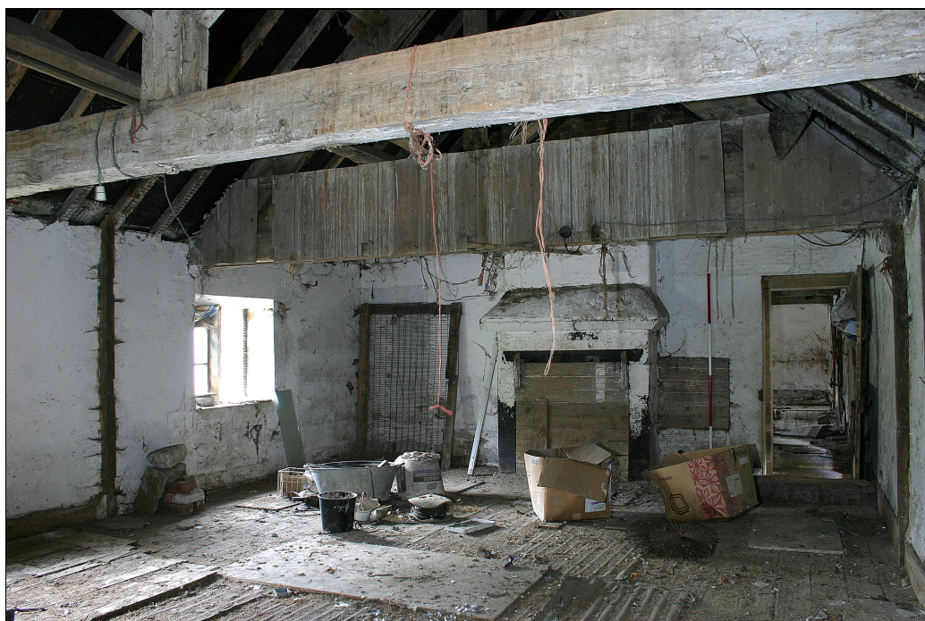
Plate 19 Building B, first floor facing west
