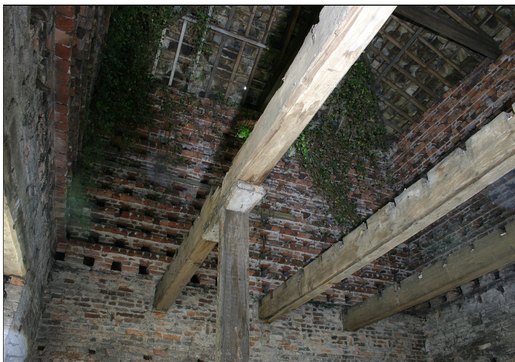
Plate 29 Building D, first floor joists and nest boxes above
