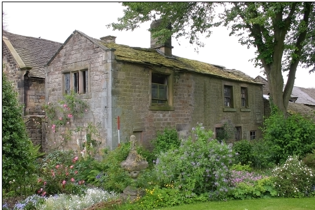
Plate 3 Building A3, wash house, north elevation
