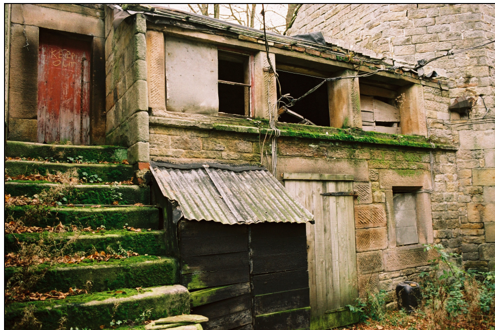
Plate 4 Building A4, hen house, south elevation Photo courtesy Rural Solutions
