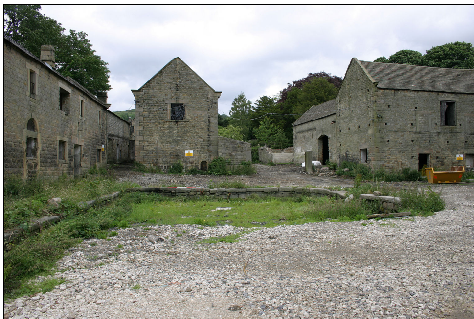
Plate 8 Buildings A,B and C, general view facing east
