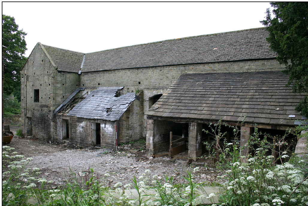
Plate 21 Building C, south elevation, with 1840's additions
