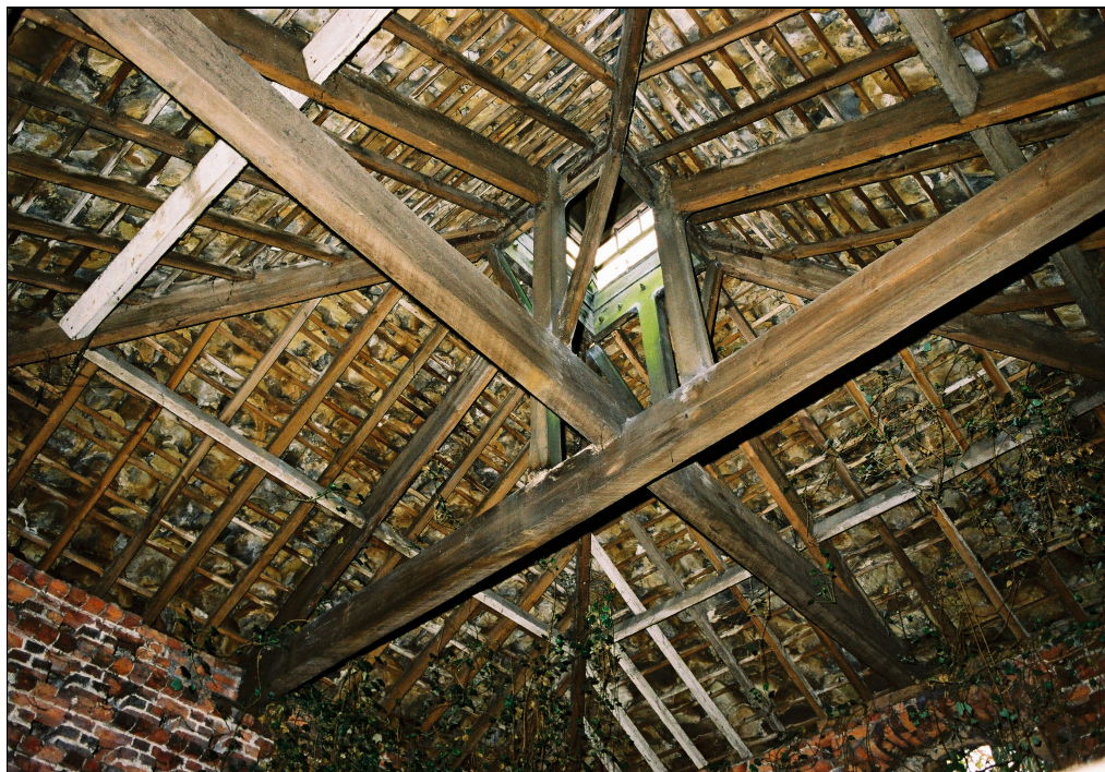
Plate 28 Building D, detail of roof structure
