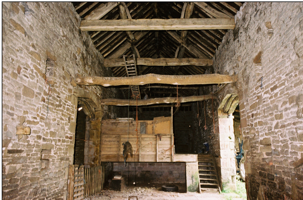
Plate 23 Building C interior, facing west Photograph courtesy Rural Solutions
