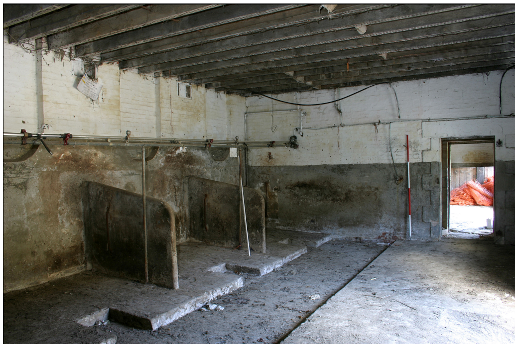
Plate 18 Building B, interior facing east
