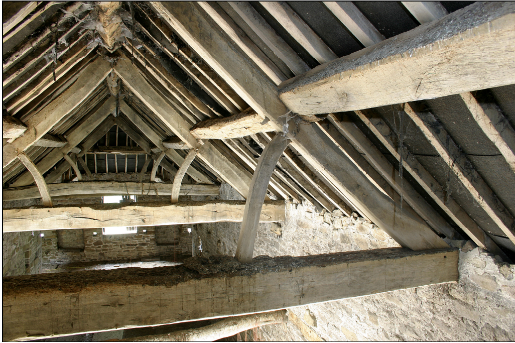
Plate 24 Building C roof structure, facing west
