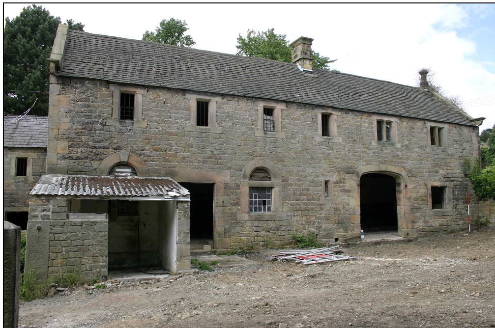
Plate 5 Building B, coach house, south elevation
