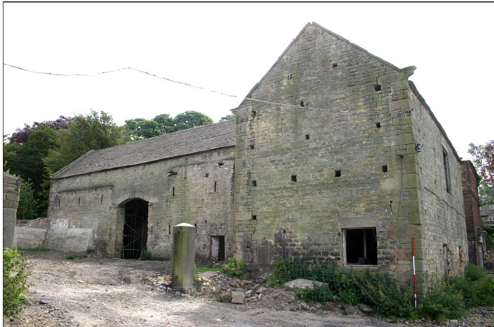
Plate 6 Building C, barn, north elevation
