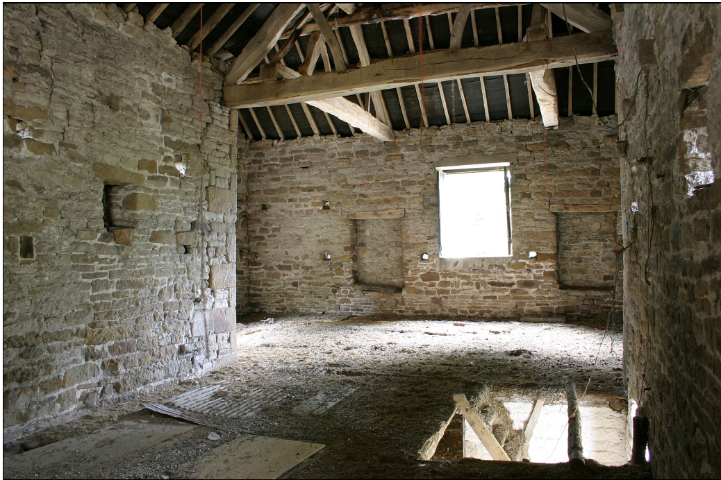
Plate 22 Building C, interior western end
