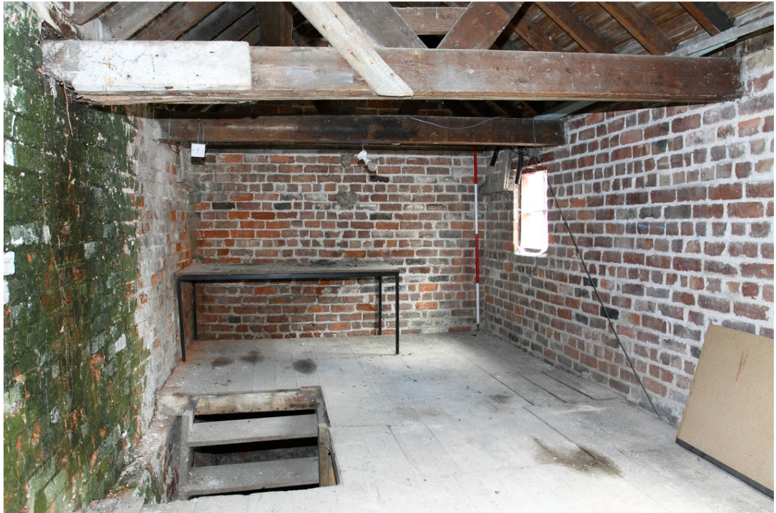
Plate 16 Building 9, first floor, looking NE
