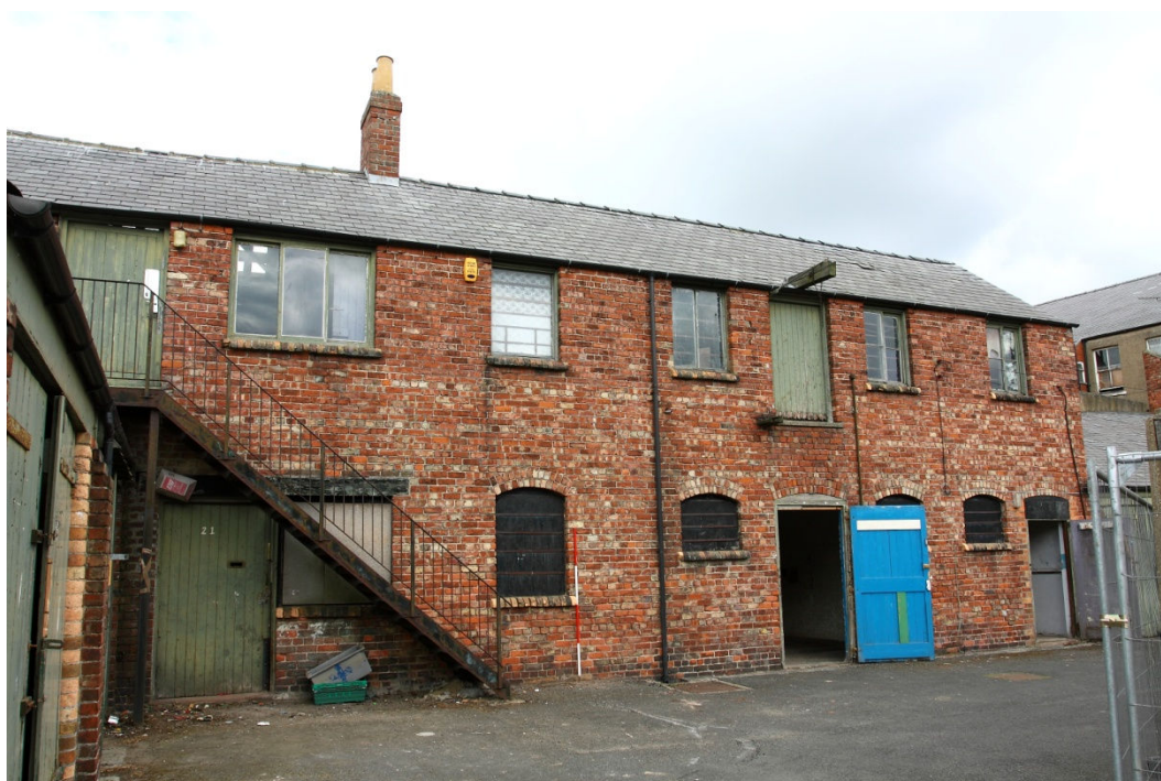
Plate 2 E elevation of two-storey part of Building 6, looking W
