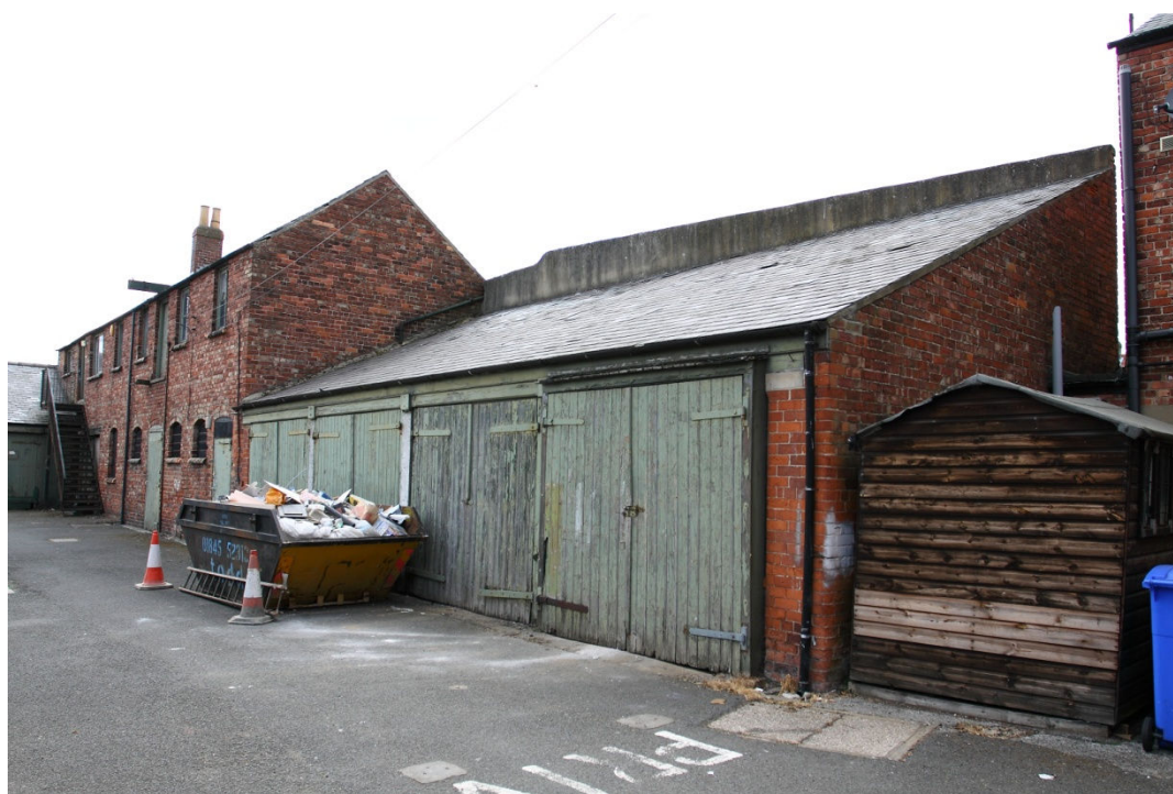
Plate 10 Façade of Spaces X,Y,Z, looking SW
