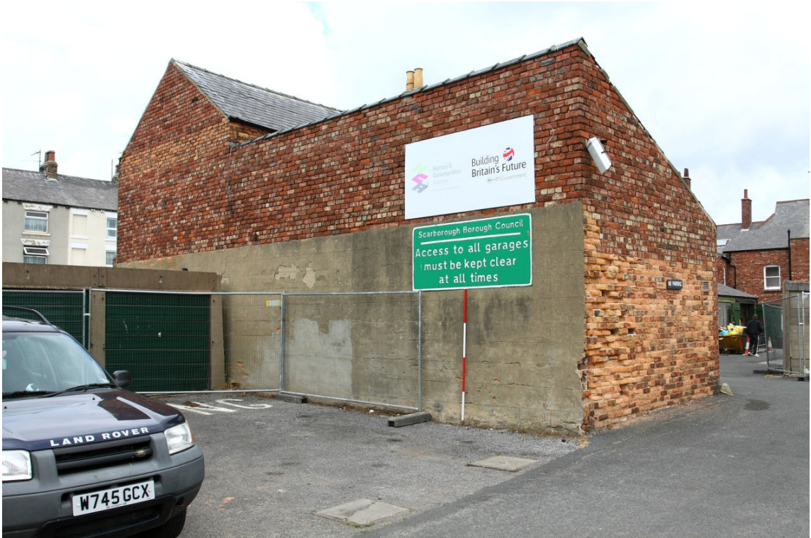
Plate 3 S elevation of Building 6, looking N
