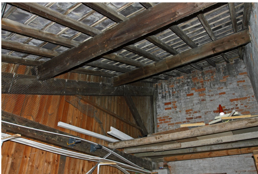
Plate 6 Roof truss of Space B, Building 6, looking SSE
