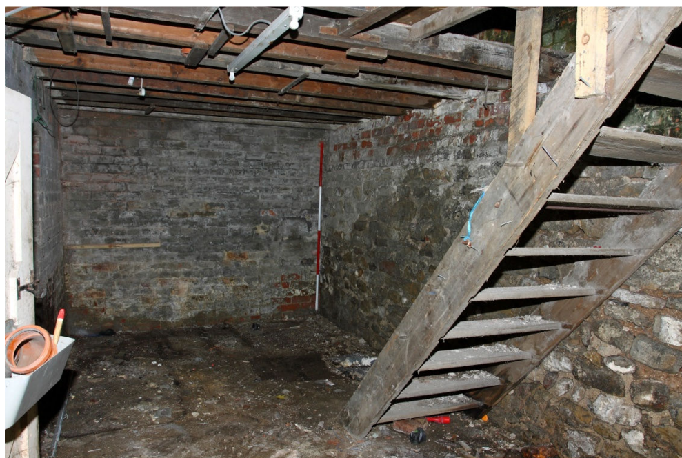
Plate 15 Building 9, ground floor, looking SW
