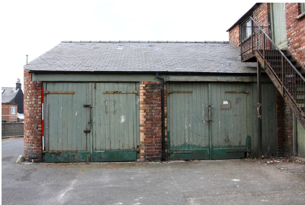
Plate 5 Exterior of Spaces A and B, Building 6, looking SW
