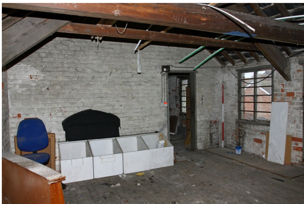
Plate 12 Space I, looking NE. Note nearest beam forms part of hoist
