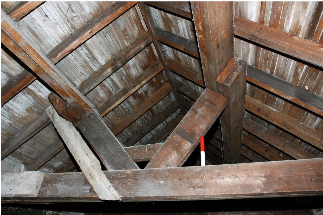
Plate 17 Building 9, detail of roof structure, looking N
