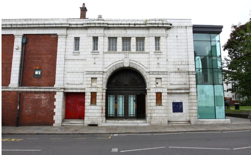
Plate 2 The ornate entrance to the foyer, looking N.W.(16jpg)
