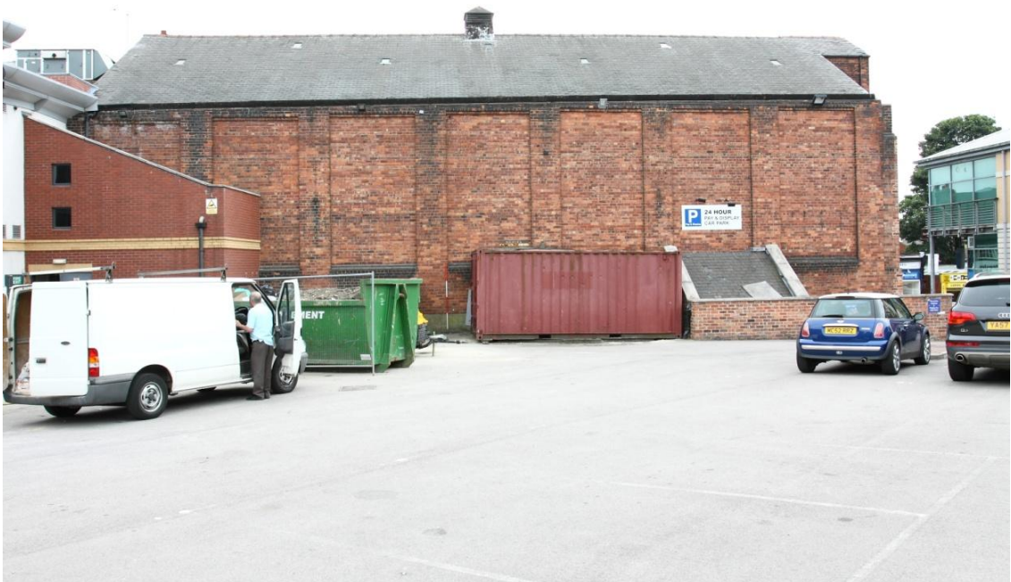
Plate 5 N.W. elevation of the cinema, looking S.E. (2jpg)
