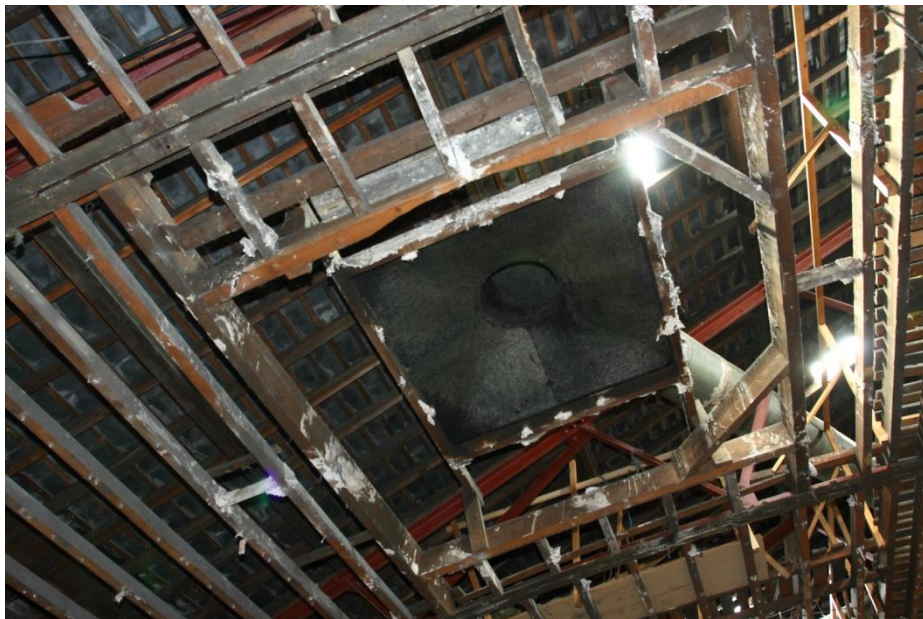
Plate 12 Roof vent, looking S.W. (37jpg)
