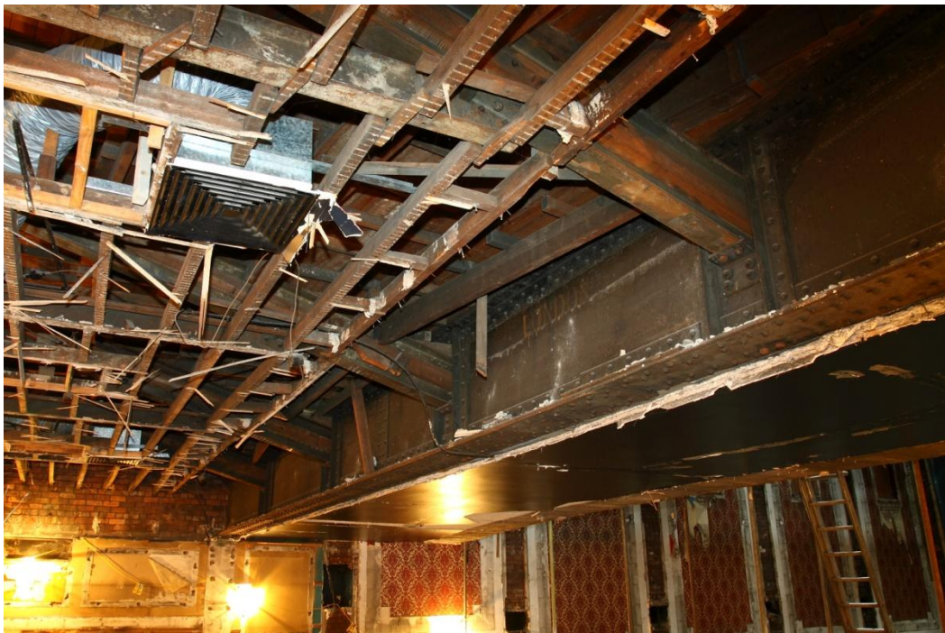
Plate 14 Structural details of the underside of the circle, looking S.S.E. (43jpg)
