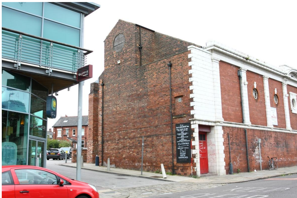
Plate 4 S.W. (end) elevation of the cinema, looking N. (5jpg)
