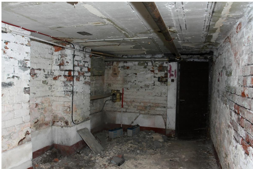
Plate 19 The N.W. chamber of the basement, looking N.W. The two brick projections to the left support the former fireplace and chimney above. (64jpg)
