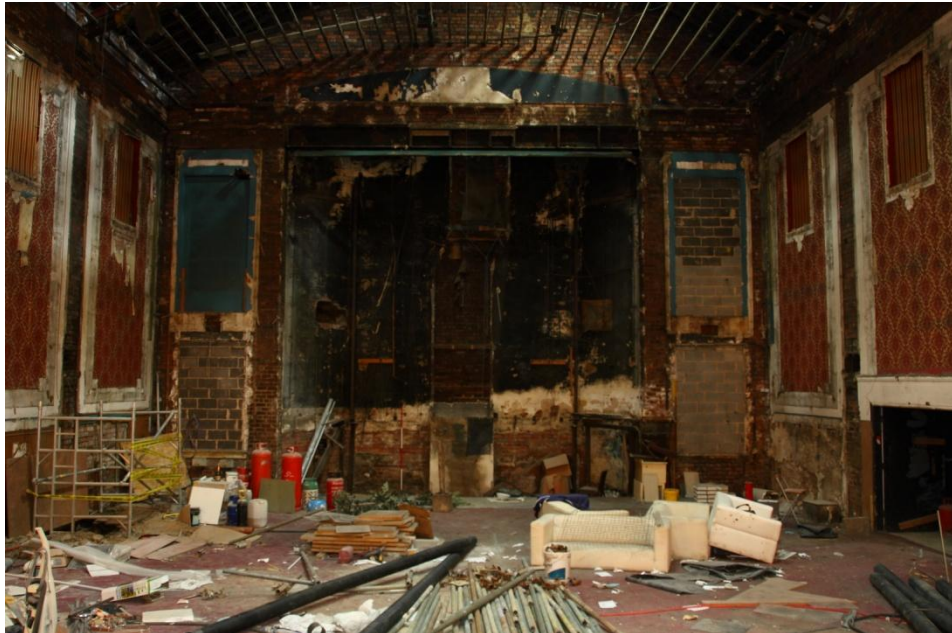
Plate 9 Screen end of the auditorium showing blocked openings to either side, looking S.W. Note chimney-like air flue in centre. (31jpg)
