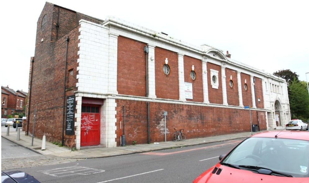
Plate 1 Overall view of the S.E. façade, looking N (8jpg)
