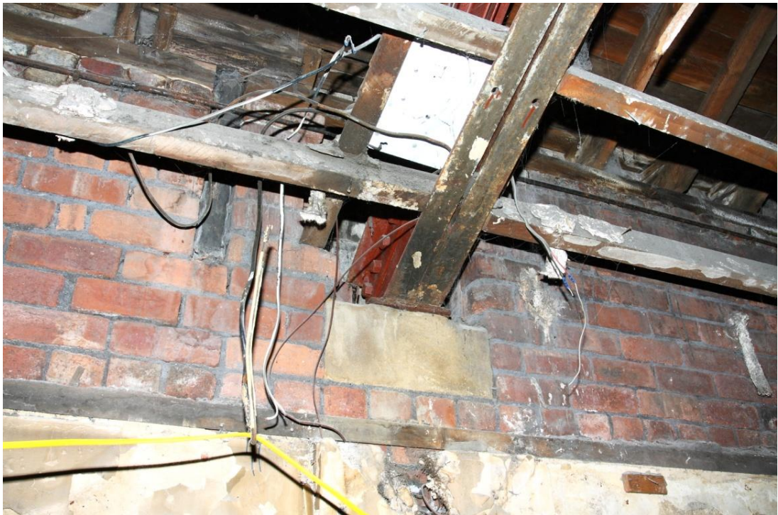
Plate 17 End of a truss sitting atop stone block, note ceiling timbers secured within 'doubled up' curved tie-beam, looking S.S.E. (39jpg)
