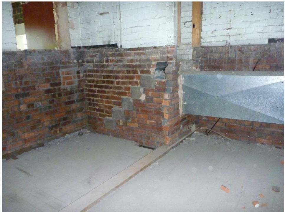
Plate 25 E. corner of the projection room, looking E. Note the truncated wall atop a girder separating the 'lantern room' (right) from the 'film room' (left). Step scars are also visible as is the door frame (top right) relating to the access to the roof space. (80jpg)
