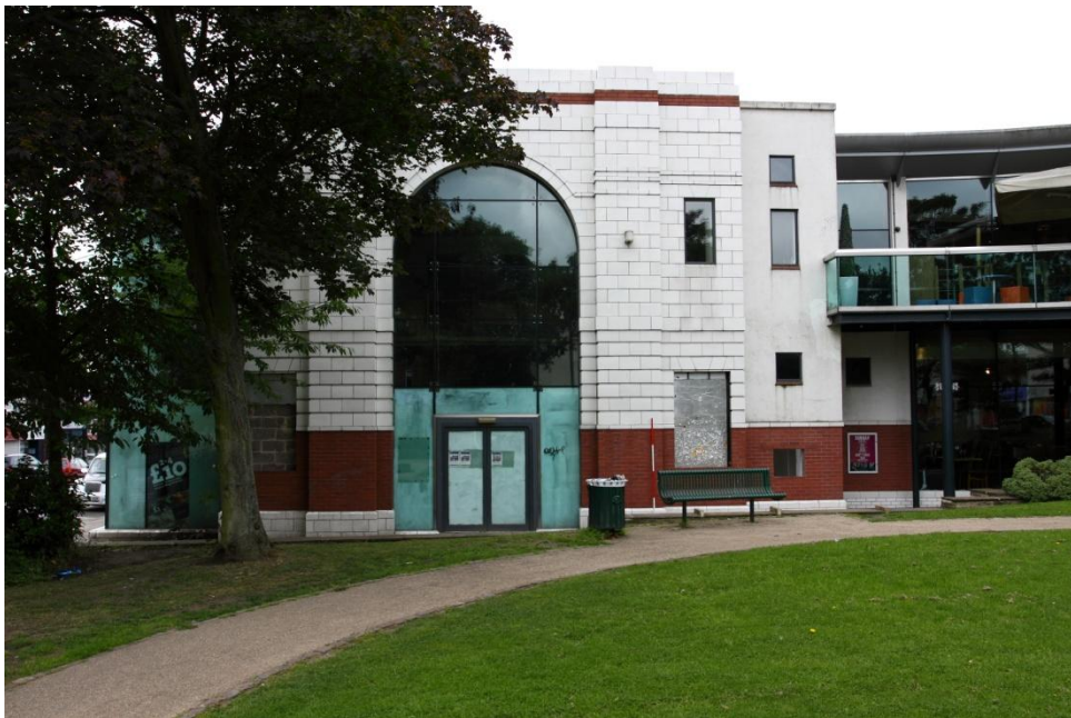
Plate 6 'Modern' N.E. elevation of the cinema, looking S.W. (14jpg)
