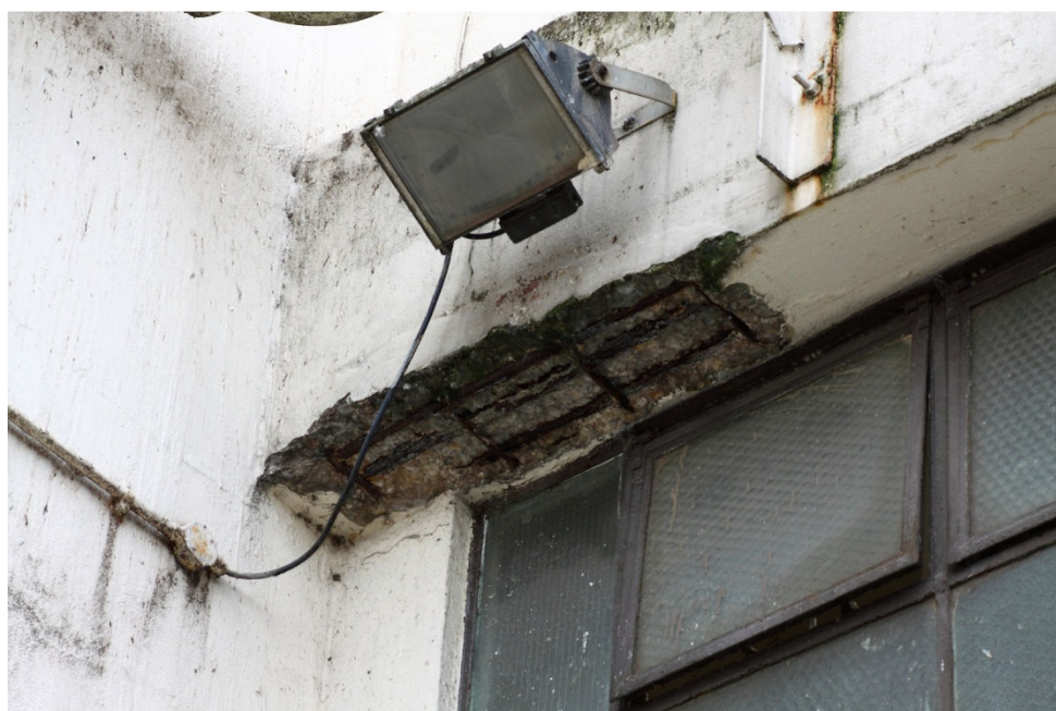
Plate 23 Detail of steel-reinforced concrete of building shell
