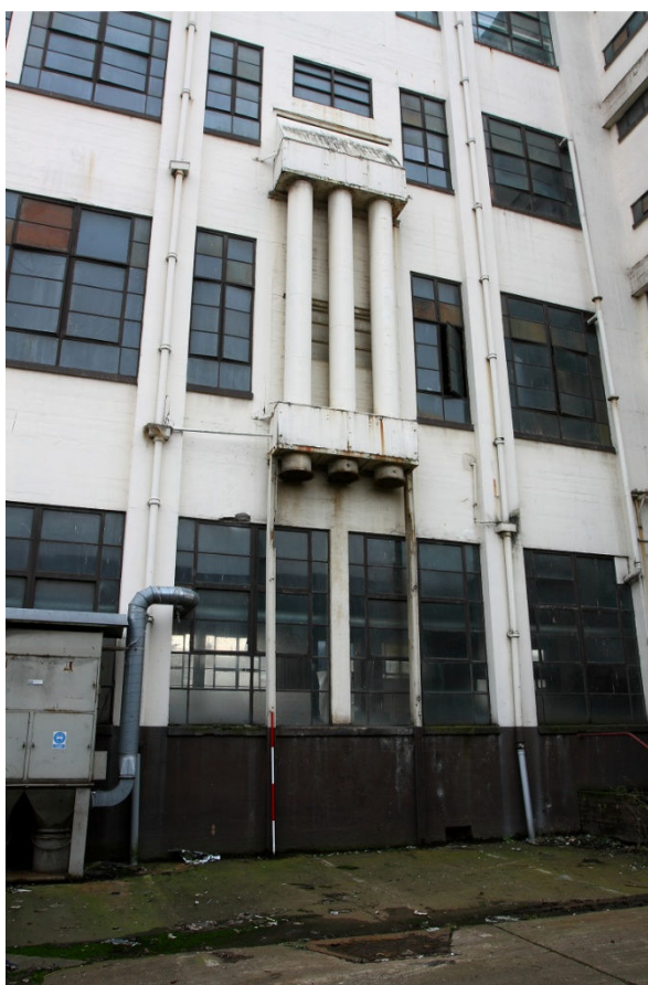
Plate 5 Waste chutes to rear elevation of building
