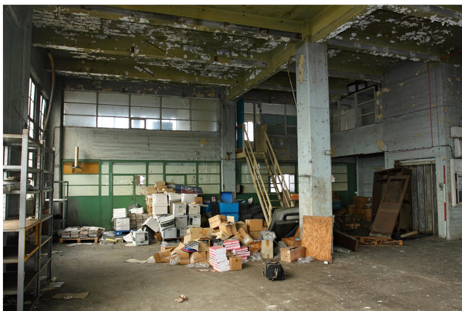
Plate 14 First floor mezzanine at NW end of building, looking NW
