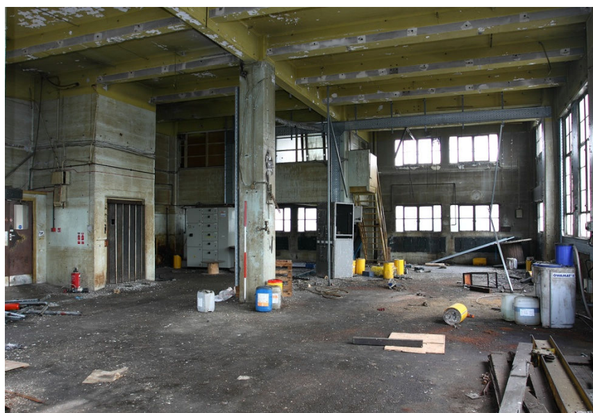
Plate 15 First floor mezzanine at SE end of building, looking ESE
