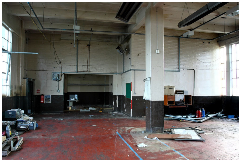
Plate 11 Later walling at SE end of ground floor, looking SE
