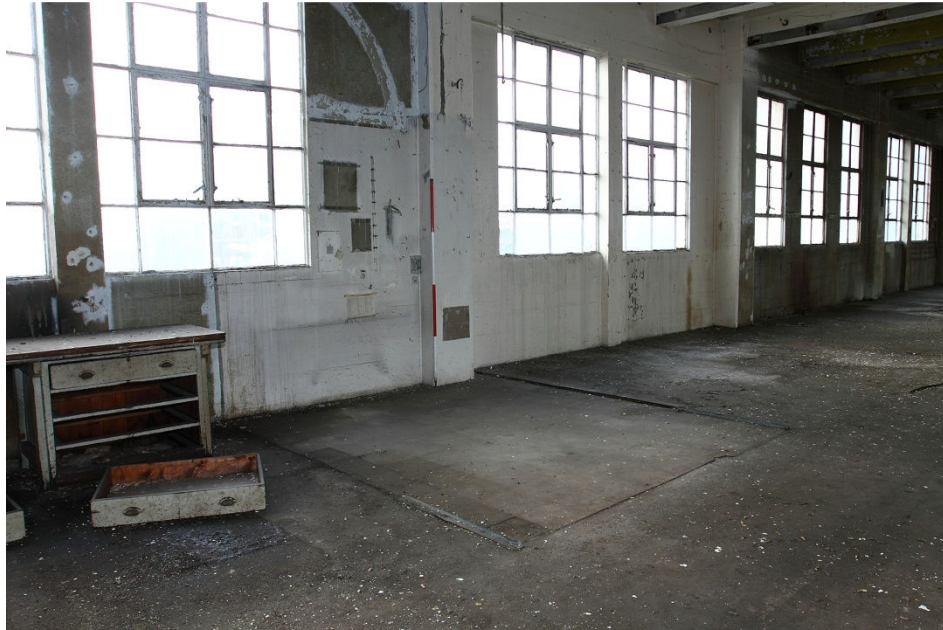
Plate 17 Second floor evidence for small enclosed space, looking W
