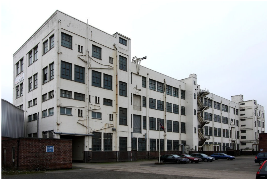
Plate 3 Rear elevation of building
