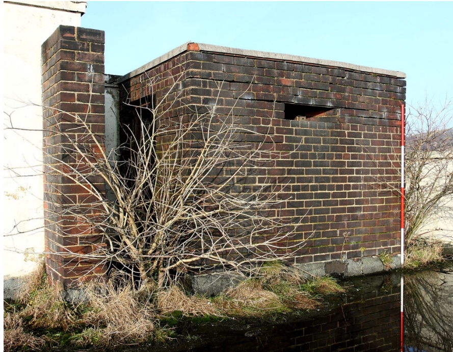
Plate 21 View of brick-built observation structure on roof, looking NNW
