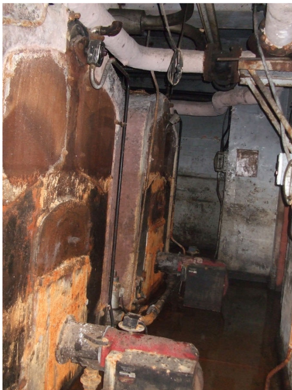
Plate 8 View of boiler room in basement
