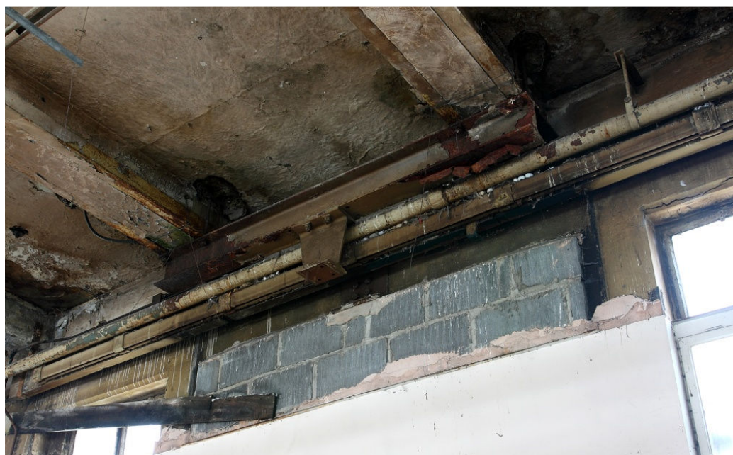
Plate 18 Third floor blocked opening with mounting for beam crane, looking N
