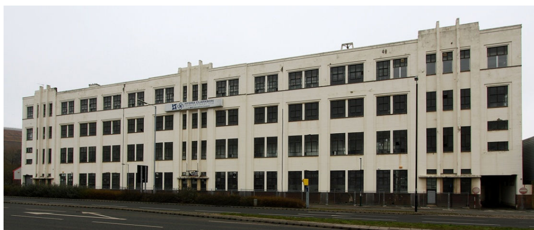
Plate 2 Front elevation of building
