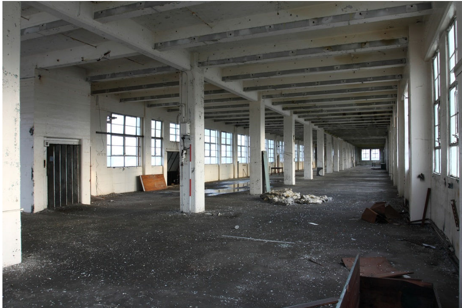
Plate 16 Second floor, looking ESE
