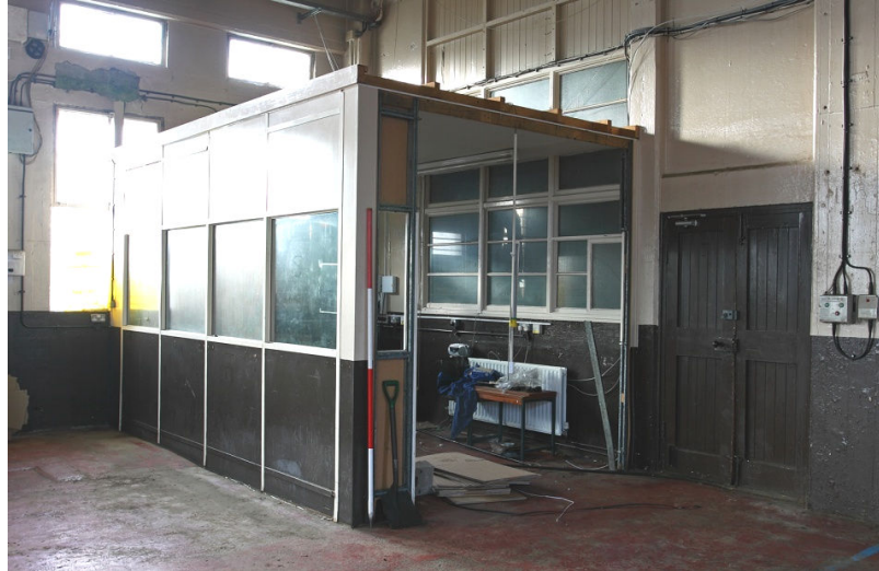
Plate 10 Office to W corner of NW end of ground floor, looking W
