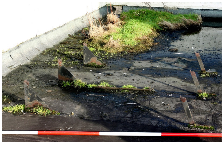
Plate 22 Mounts for signage on roof, looking NNE
