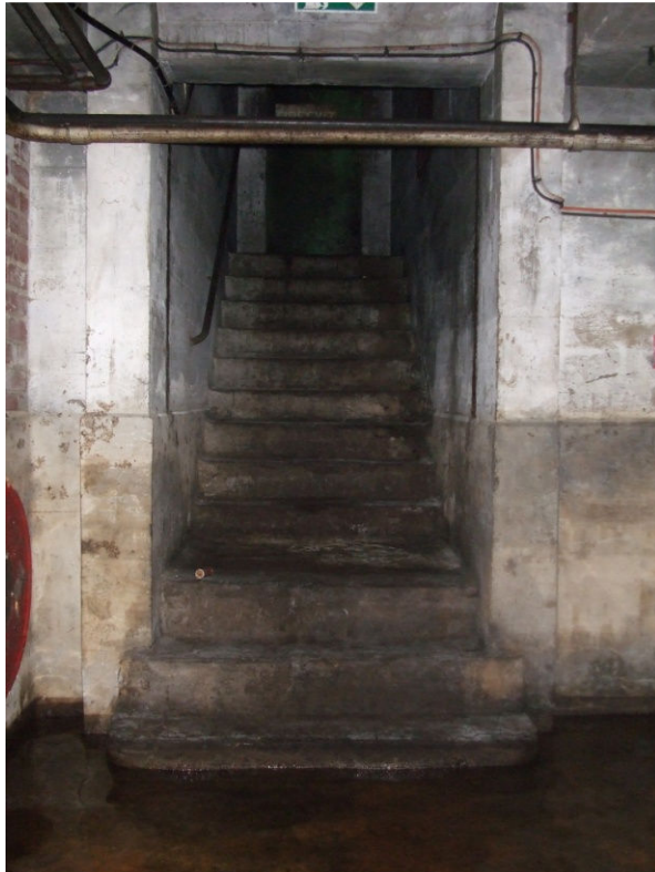
Plate 7 Access to basement via one of 'air raid' entrances
