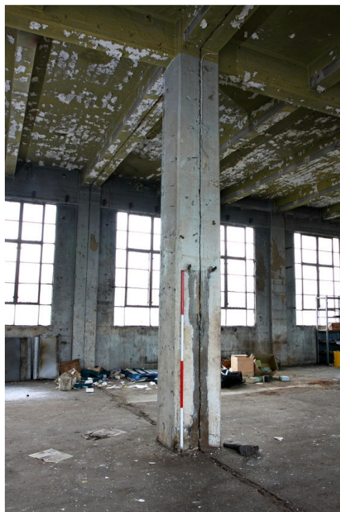
Plate 13 Structural division within building, first floor looking WSW
