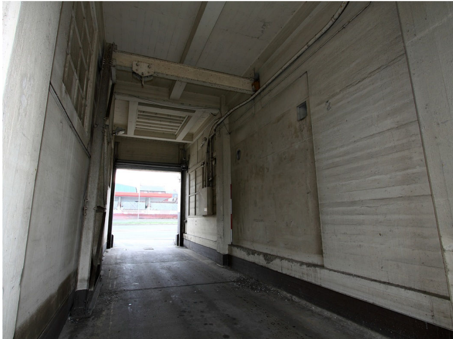
Plate 6 Passage-way to SE side of building, looking SW
