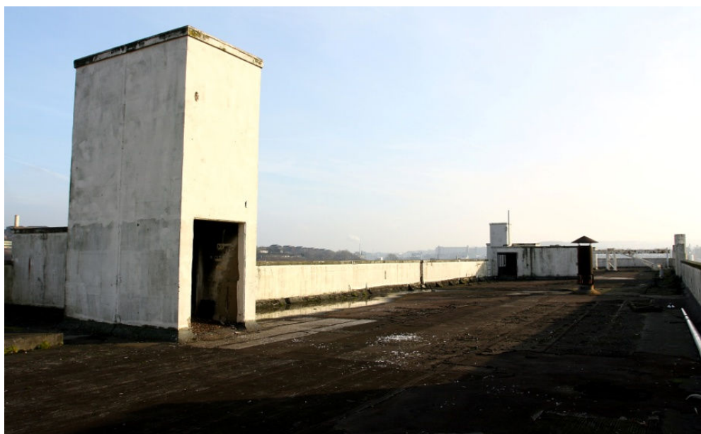
Plate 19 View of roof, NW lift shaft in foreground, looking ESE
