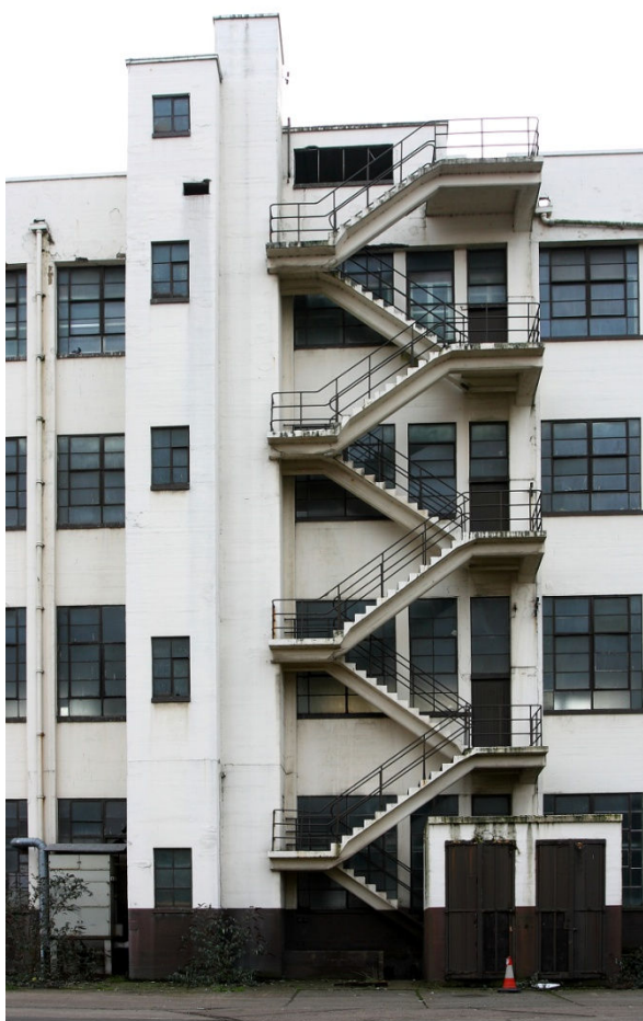
Plate 4 Fire escape to rear elevation of building
