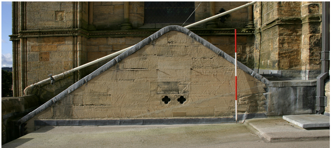
Plate 5 View of west end of south aisle roof showing roof scar of original roof-line. Scale in 0.5m units
