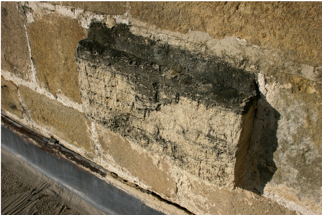
Plate 2 One of the cut-away corbels on the south face of the nave walling.
