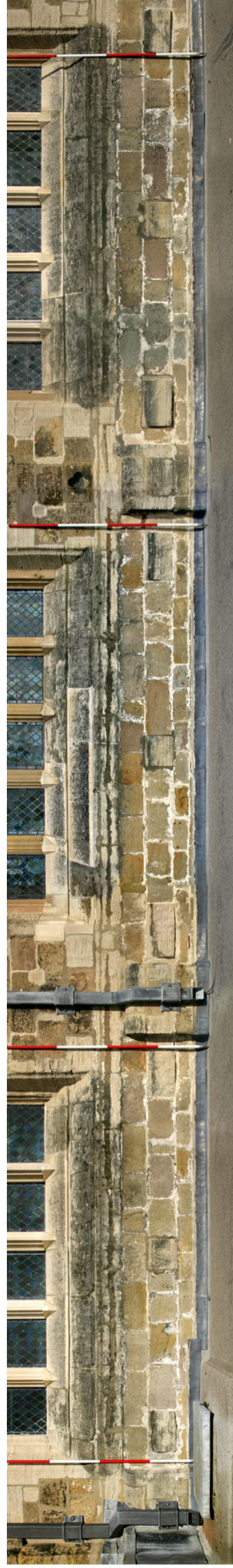
View of western part of top photograph, showing roof scar of original roof-line (immediately below window surround) and cut-away corbels (three per bay).
