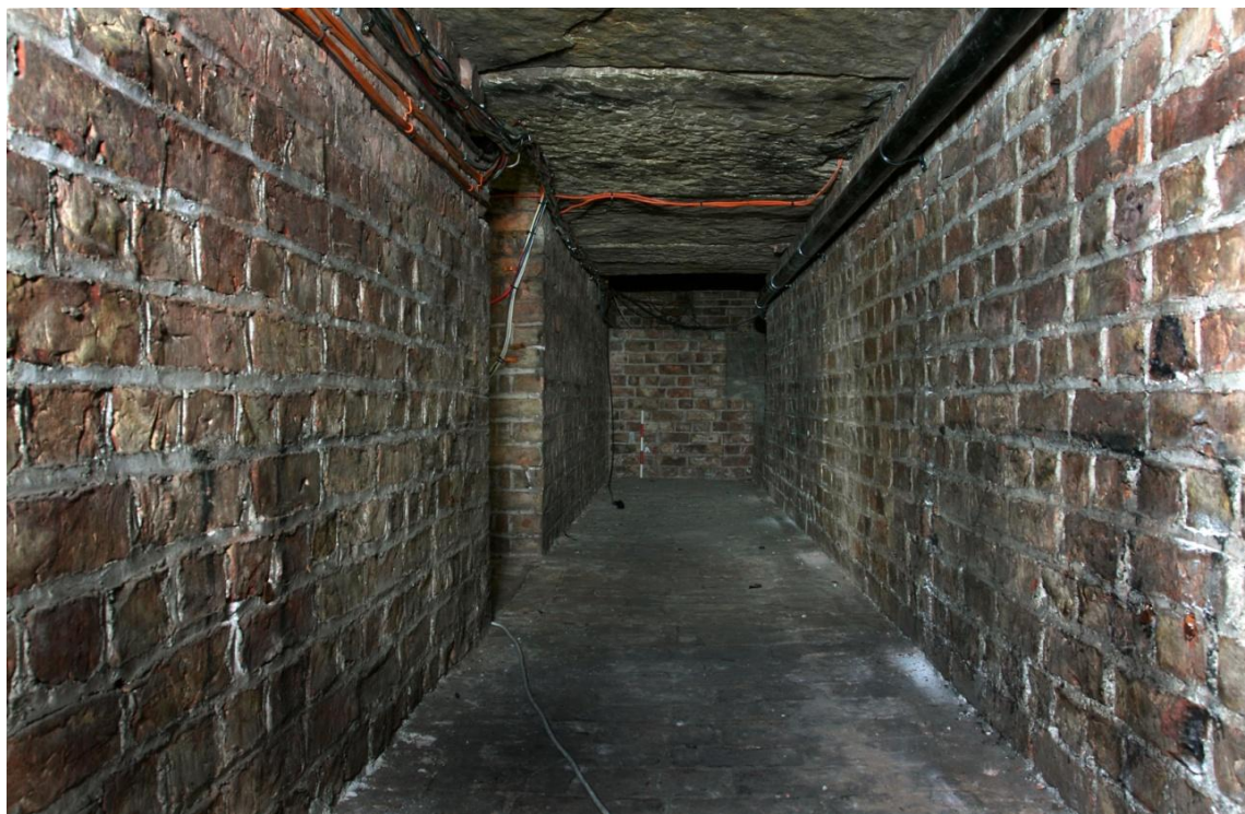
Plate 1 Arm of the 'T' shaped organ ducts, looking N
