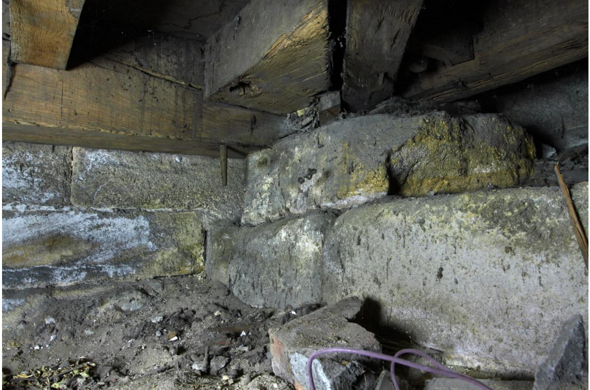
Plate 6 West side of N line of early walling (right) showing the walling of the present W end of the choir overriding the earlier work, looking WNW
