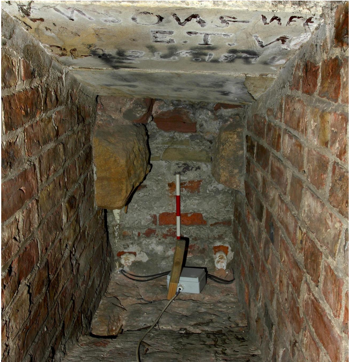
Plate 13 Rear of the crypt at W end of tunnel, looking W
