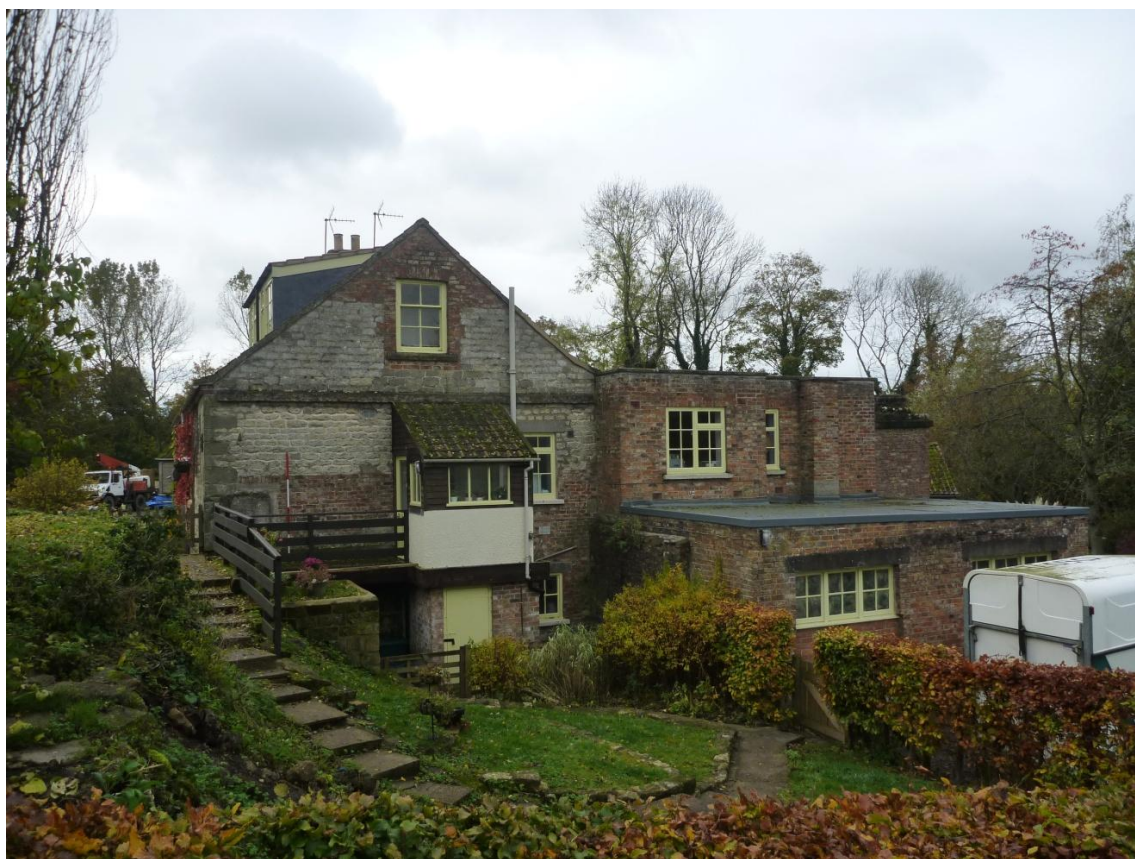
Plate 8 Side (NE) elevation of the mill. The present entrance to the former mill building is via the timber lean-to. Note the altered brick extensions now covered by flat roofs
