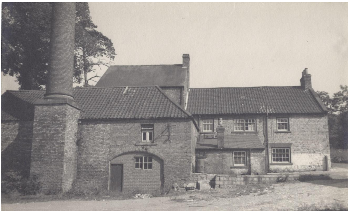
Plate 4 Rear, NW facing, elevation of Mill House and adjacent mill
