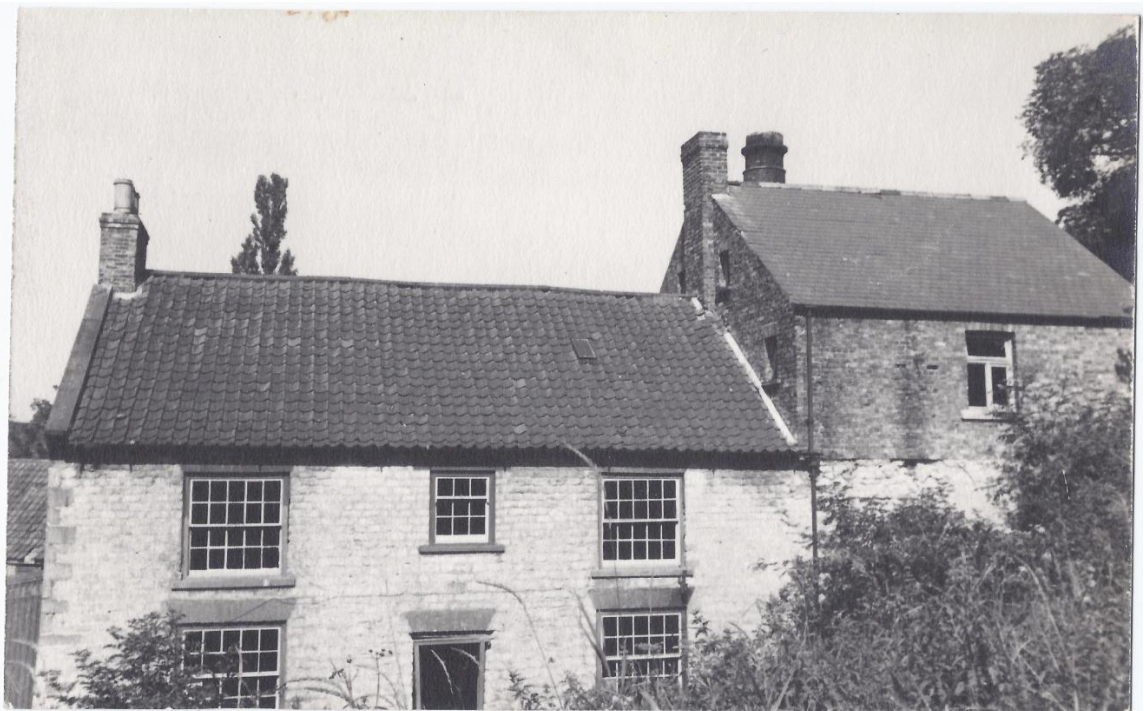
Plate 1 Front, SE facing, elevation of Mill House and adjacent mill
