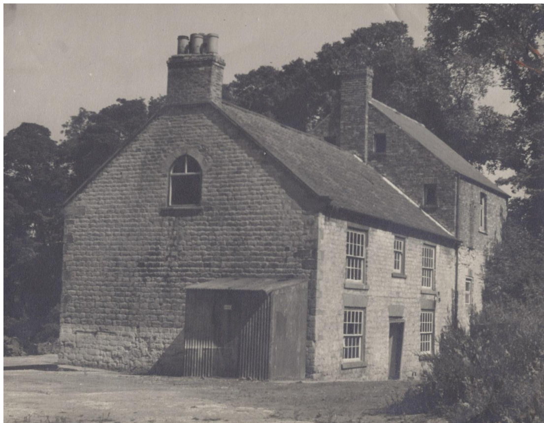
Plate 2 SE and SW facing, elevations of Mill House and adjacent mill
