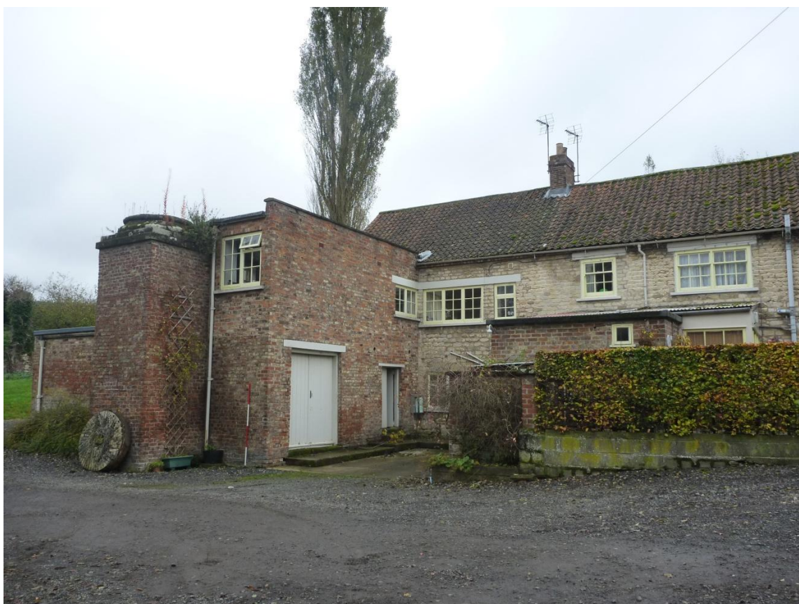
Plate 10 Rear of the mill complex. Note the truncated chimney and brick extensions.
