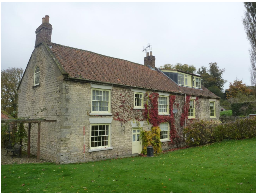
Plate 6 Front (SE) elevation of Mill House and adjacent mill
