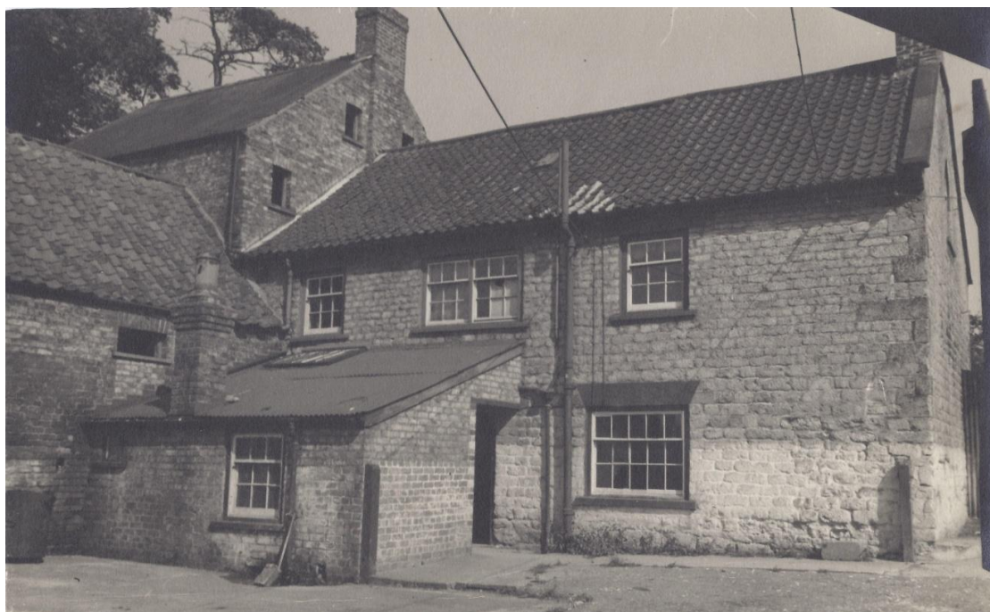
Plate 3 Rear, NW facing, elevation of Mill House and parts of NW facing sides of mill
