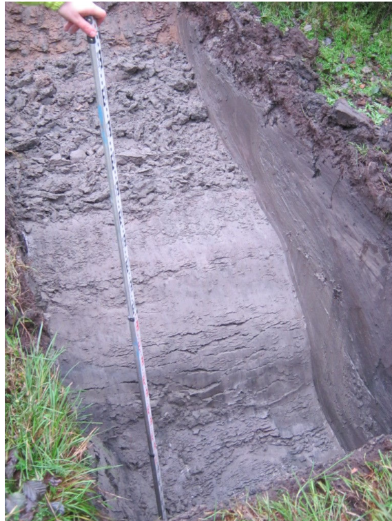
Plate 6 Trial Pit looking east
