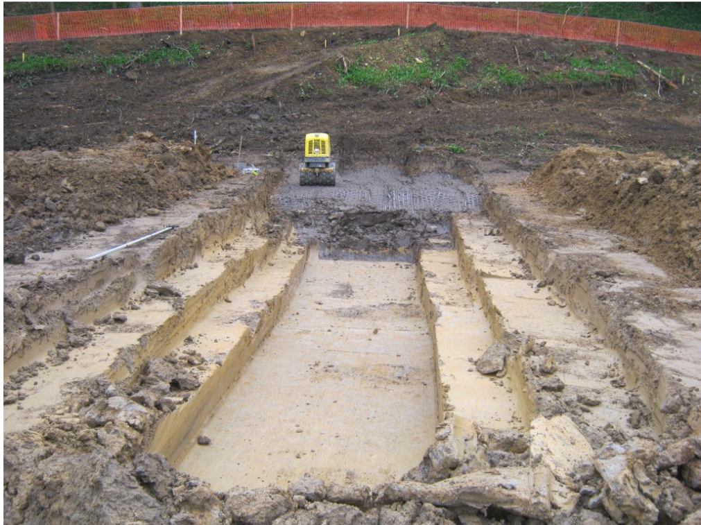
Plate 8 Watching brief natural clays & key trench profile facing south-west
