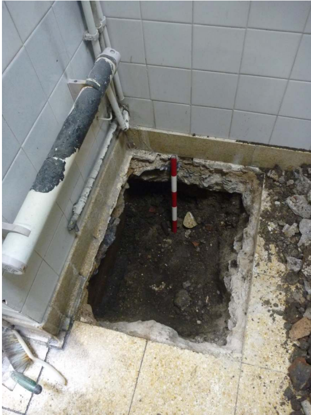
Plate 1: Post excavation shot of trial hole
