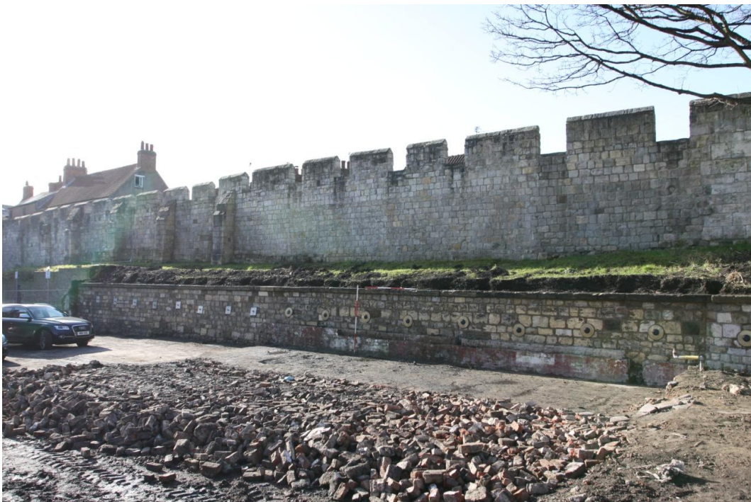
22. South facing view of the retaining wall. Scale units 0.5m
