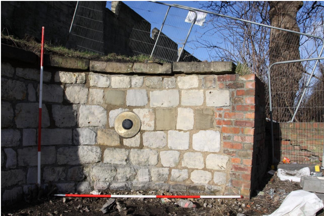
17. West facing view of the retaining wall. Scale units 0.5m
