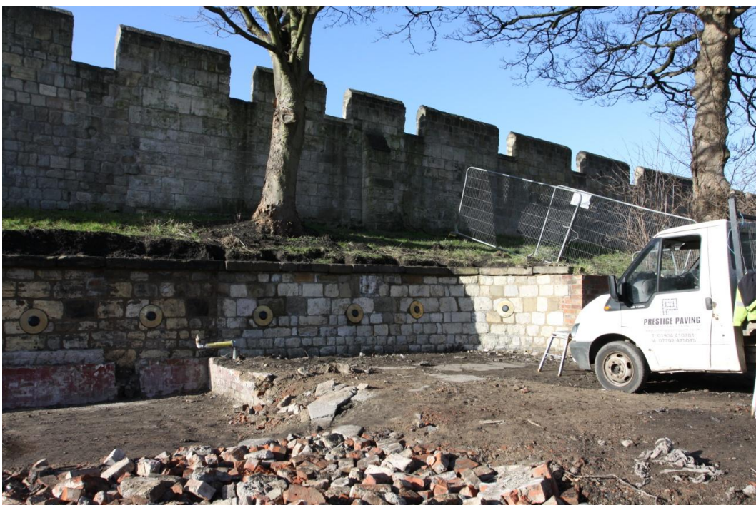
18. West facing view of the retaining wall
