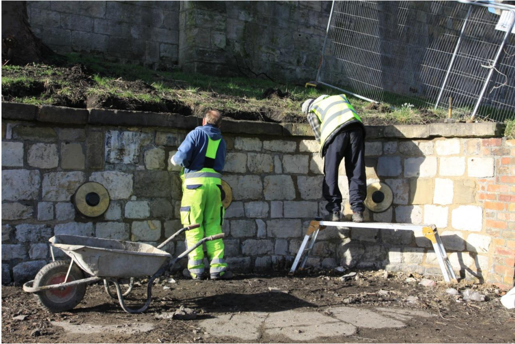
35. West facing view of the retaining wall during restoration
