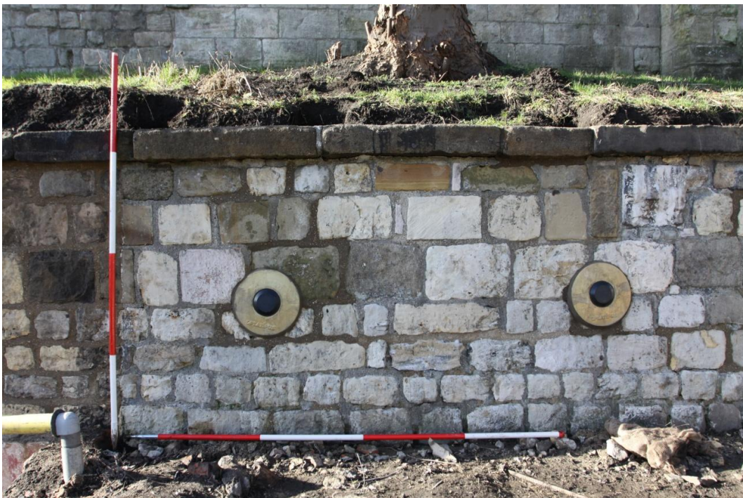
14. South-west facing view of the retaining wall. Scale units 0.5m
