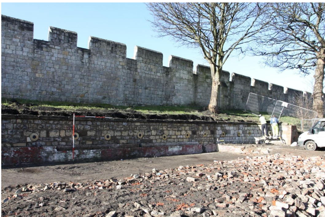
20. West facing view of the retaining wall. Scale units 0.5m
