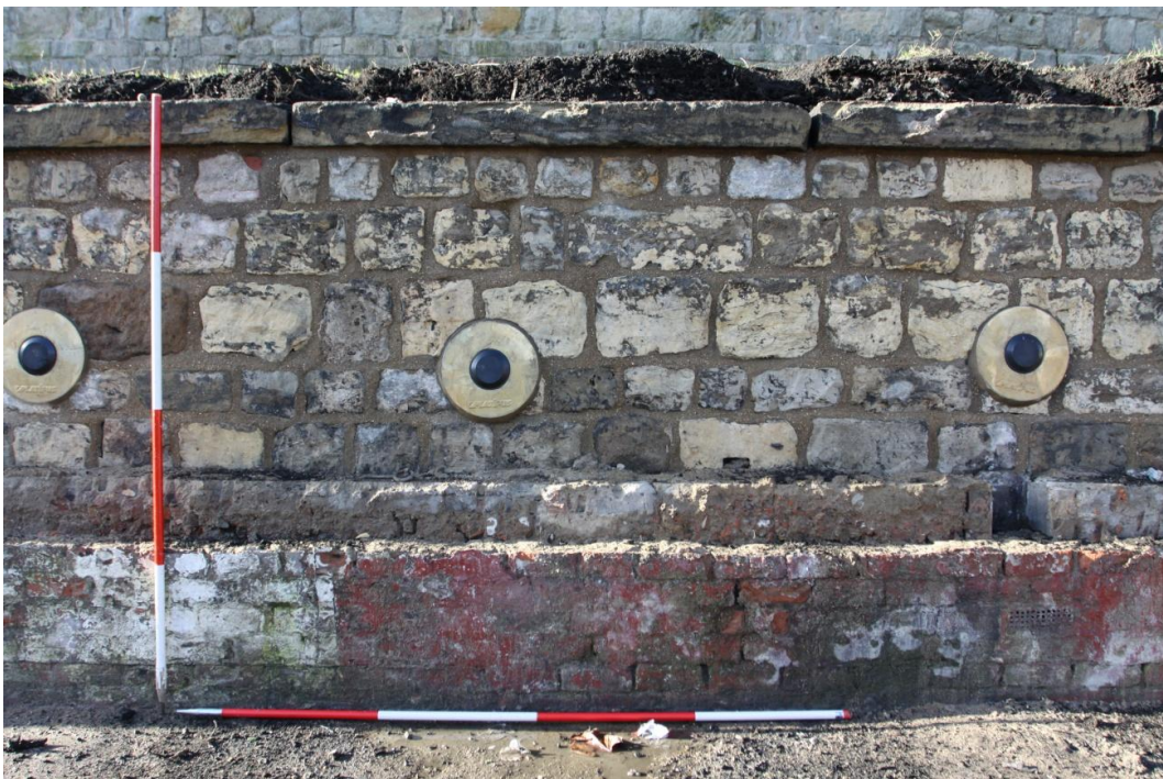
10. South-west facing view of the retaining wall. Scale units 0.5m
