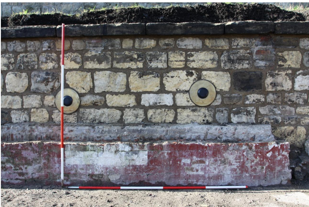
12. South-west facing view of the retaining wall. Scale units 0.5m
