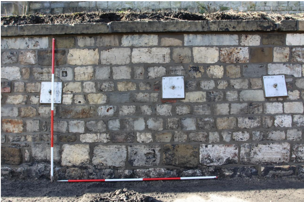
6. South-west facing view of the retaining wall. Scale units 0.5m
