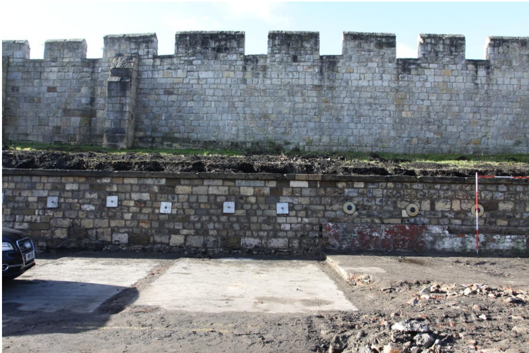
29. South-west facing view of the retaining wall. Scale units 0.5m
