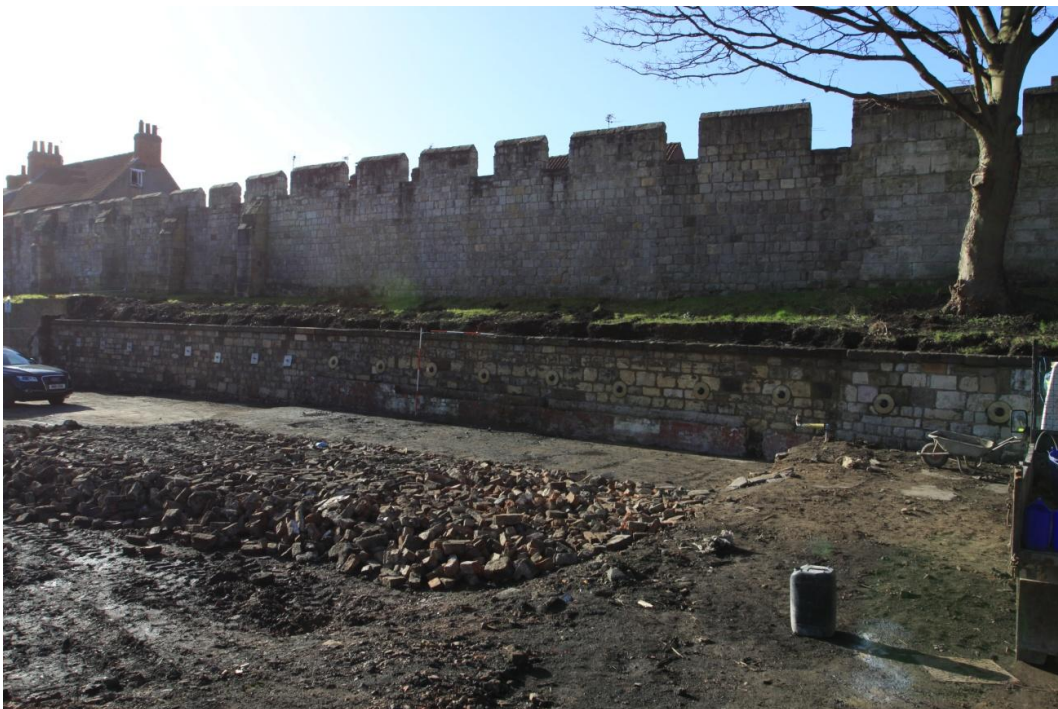
34. South facing view of the retaining wall. Scale units 0.5m
