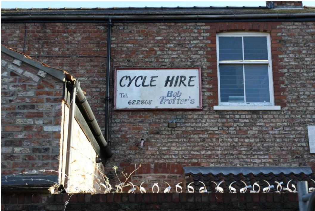
3. Detail of nearby 19th century buildings
