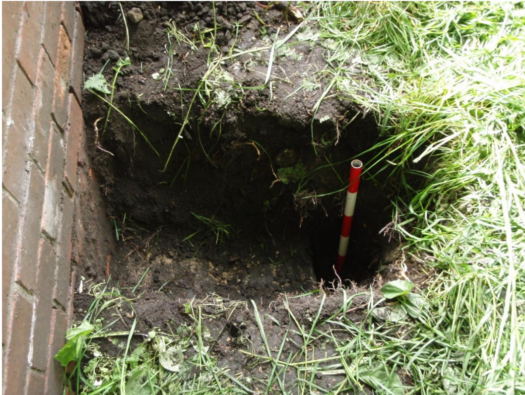
Plate 4. South-east facing view of Trial Pit 3. Scale units 0.10m
