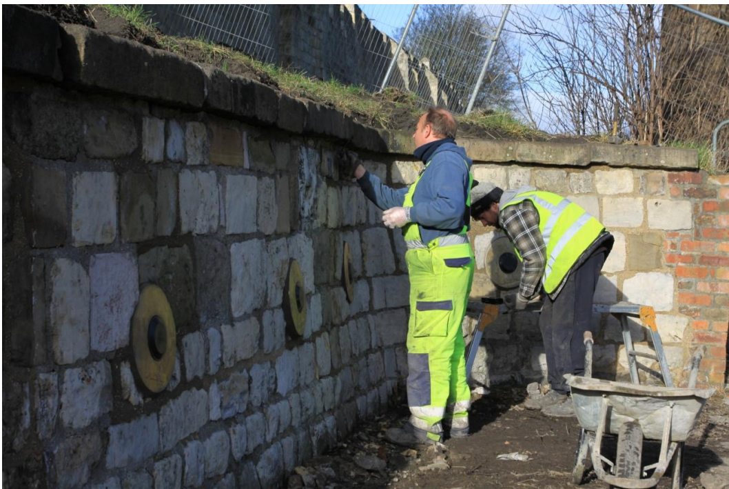
36. West facing view of the retaining wall during restoration
