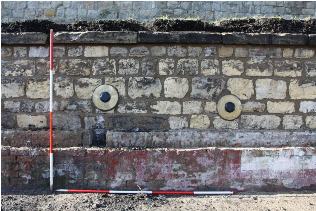
11. South-west facing view of the retaining wall. Scale units 0.5m
