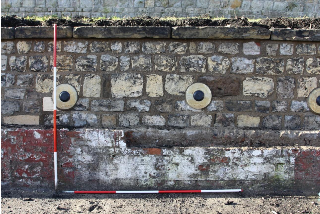
9. South-west facing view of the retaining wall. Scale units 0.5m
