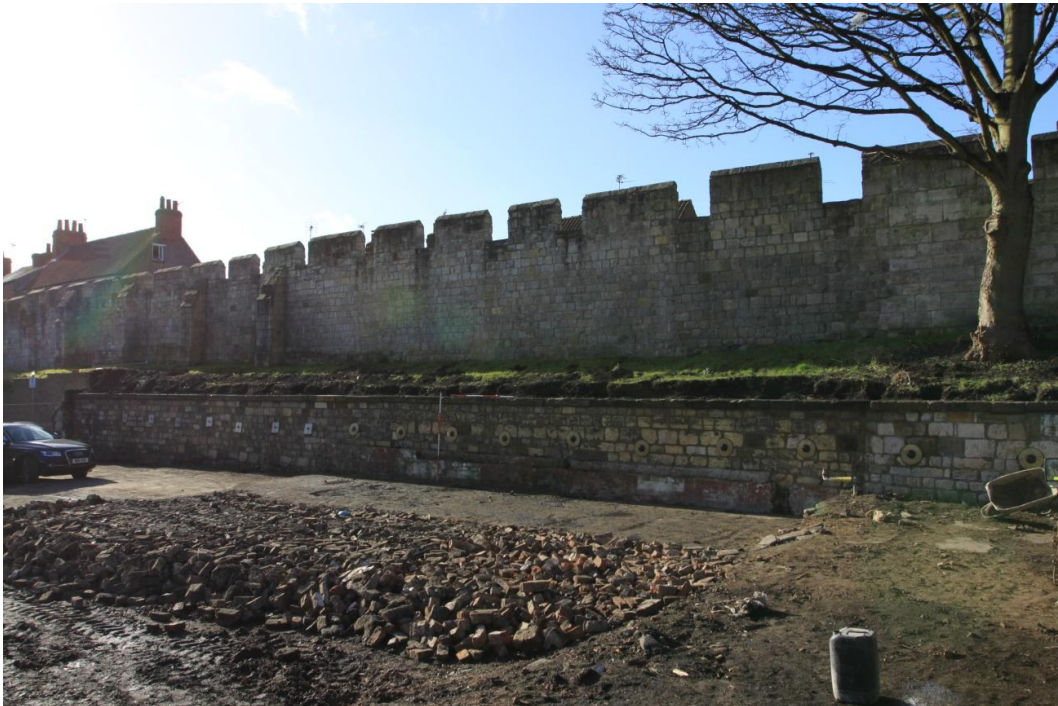
31. South facing view of the retaining wall. Scale units 0.5m
