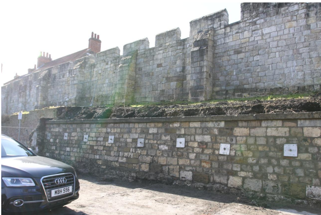
30. South facing view of the retaining wall
