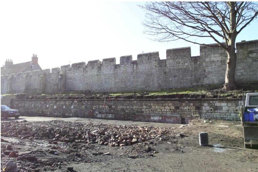
26. South facing view of the retaining wall. Scale units 0.5m
