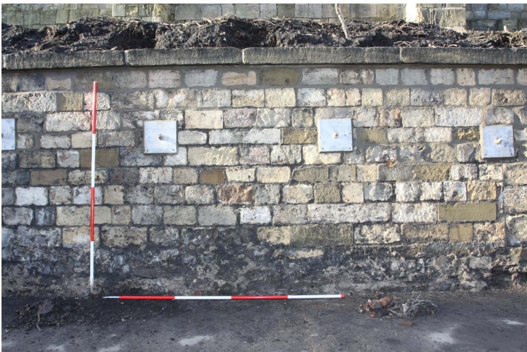
2. South-west facing view of the retaining wall. Scale units 0.5m
