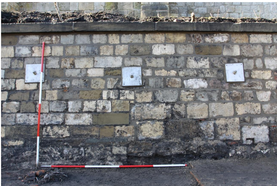
4. South-west facing view of the retaining wall. Scale units 0.5m
