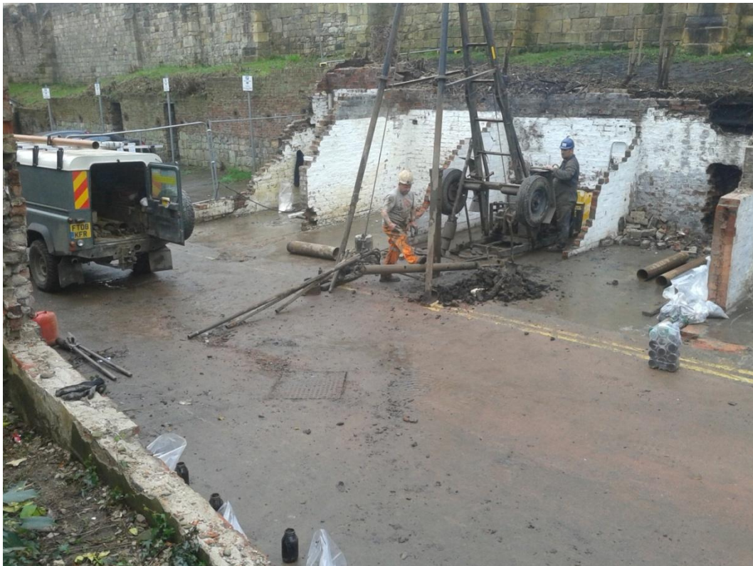
Plate 8. Borehole 1 under excavation.
