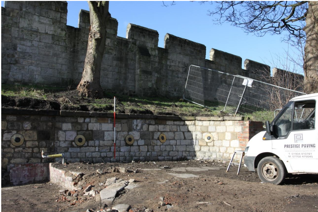
19. West facing view of the retaining wall. Scale units 0.5m
