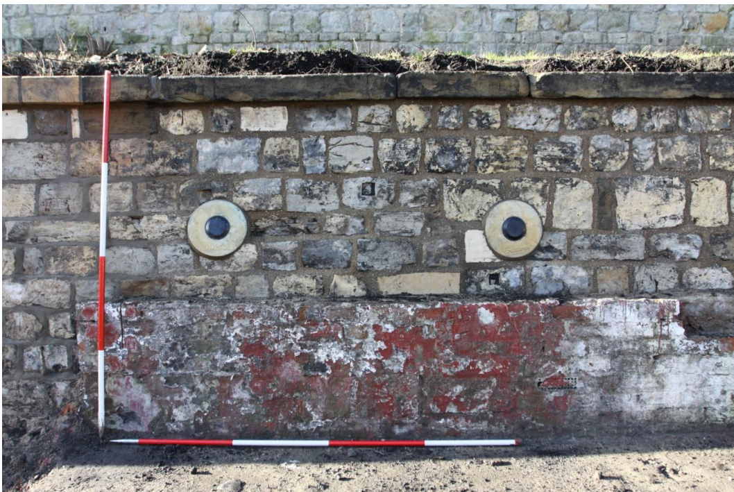
8. South-west facing view of the retaining wall. Scale units 0.5m
