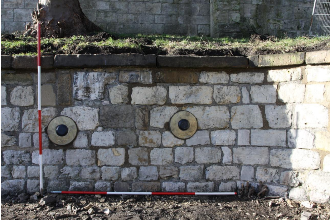
15. South-west facing view of the retaining wall. Scale units 0.5m
