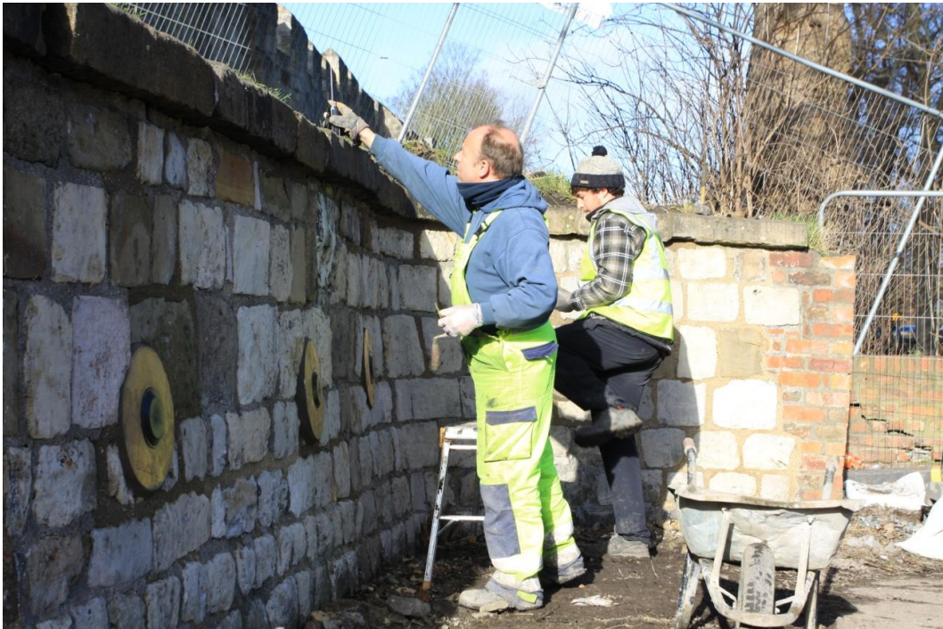
37. West facing view of the retaining wall during restoration
