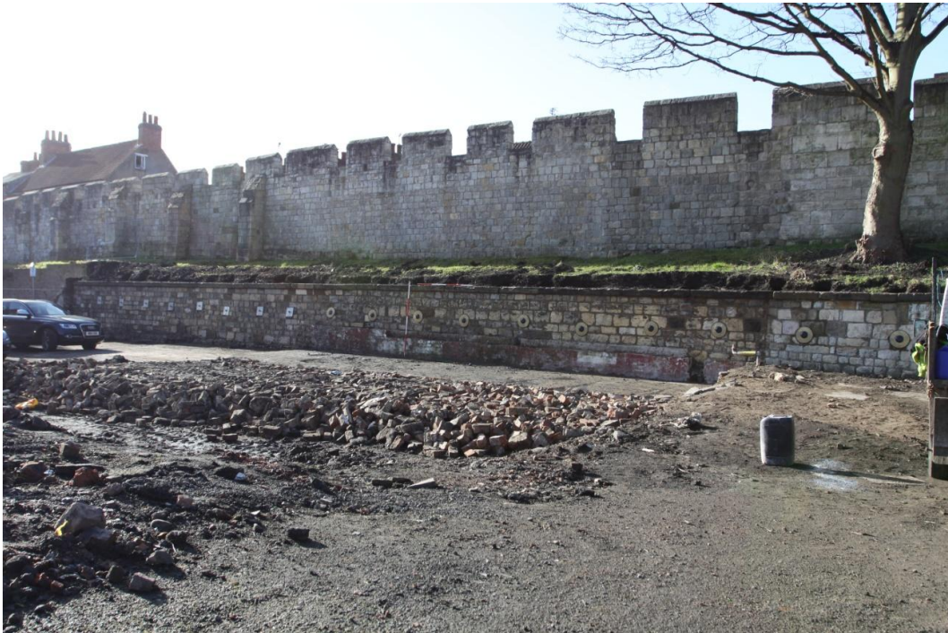
25. South facing view of the retaining wall. Scale units 0.5m
