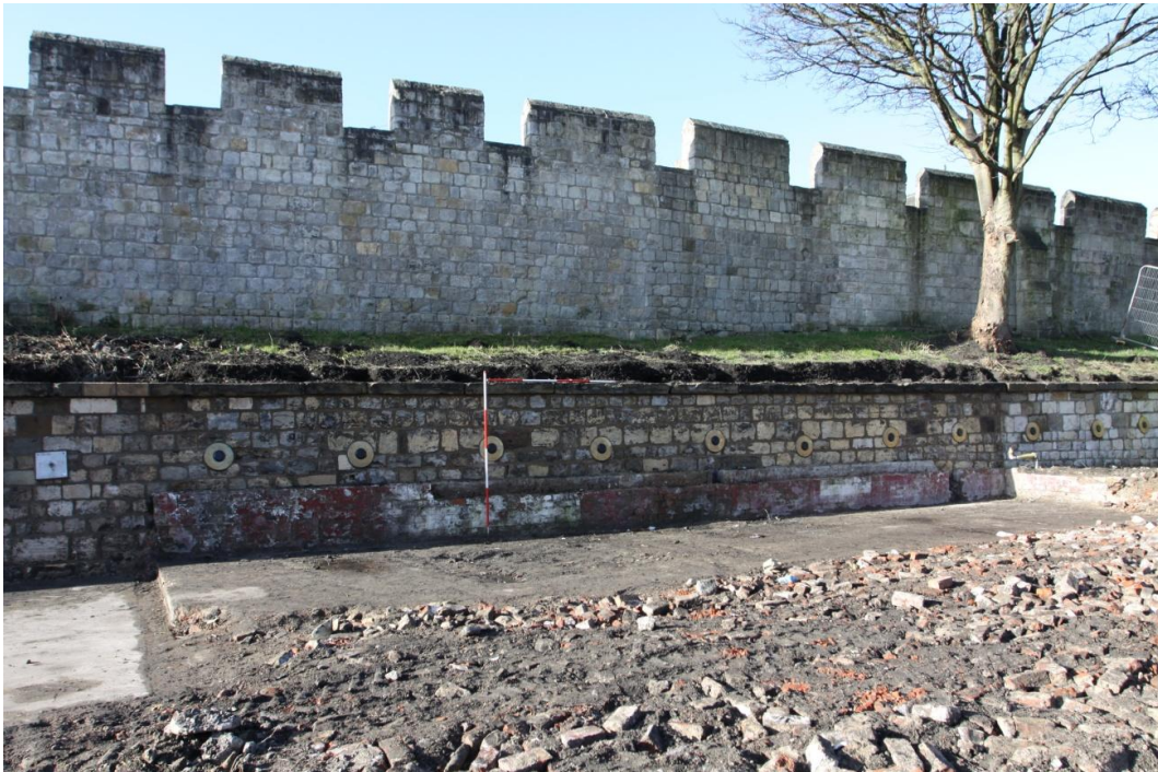
21. West facing view of the retaining wall. Scale units 0.5m
