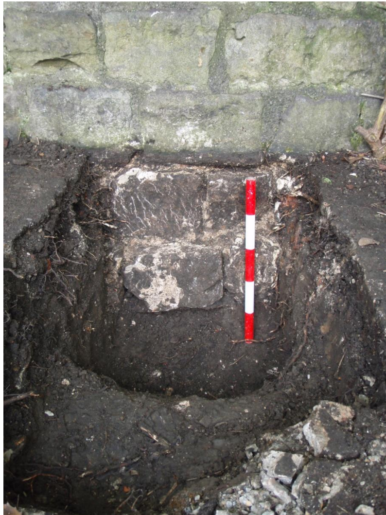
Plate 6. South-west facing view of Trial Pit 5 and the retaining wall footings. The clayey material beneath the stonework relates to the ramparts. Scale units 0.10m
