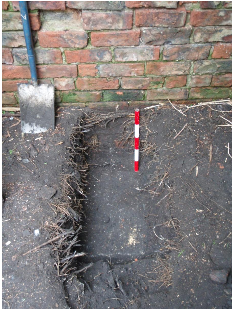
Plate 1. North-east facing view of Trial Pit 1. Scale units 0.10m
