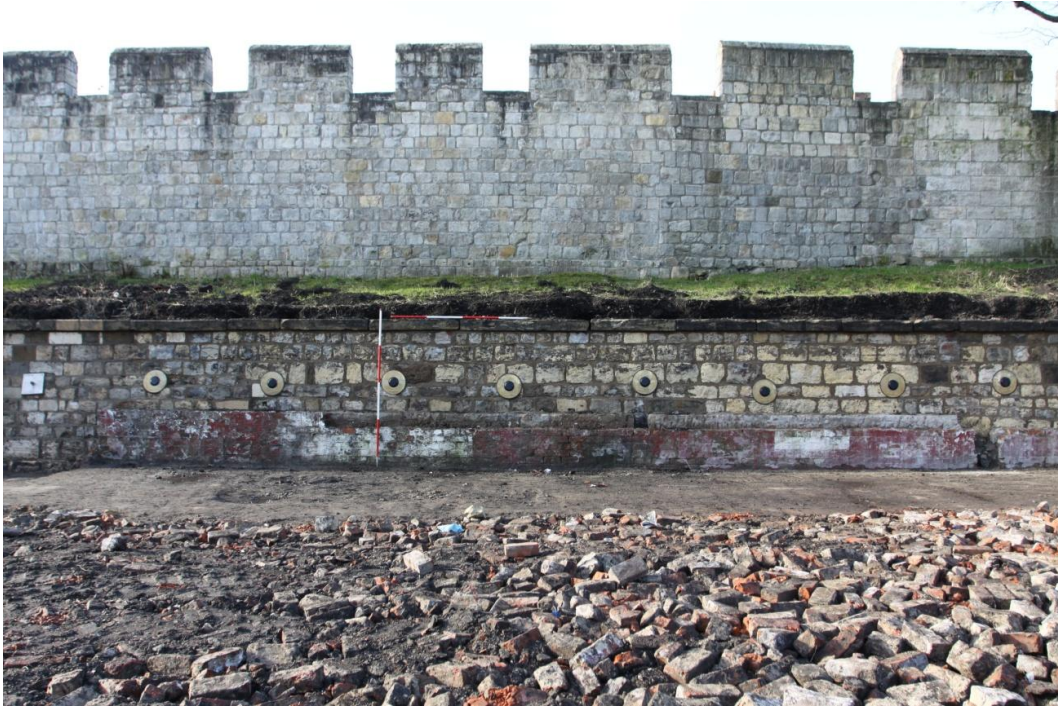
27. South-west facing view of the retaining wall. Scale units 0.5m
