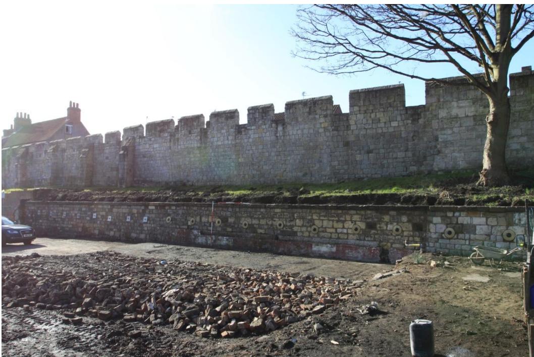
32. South facing view of the retaining wall. Scale units 0.5m
