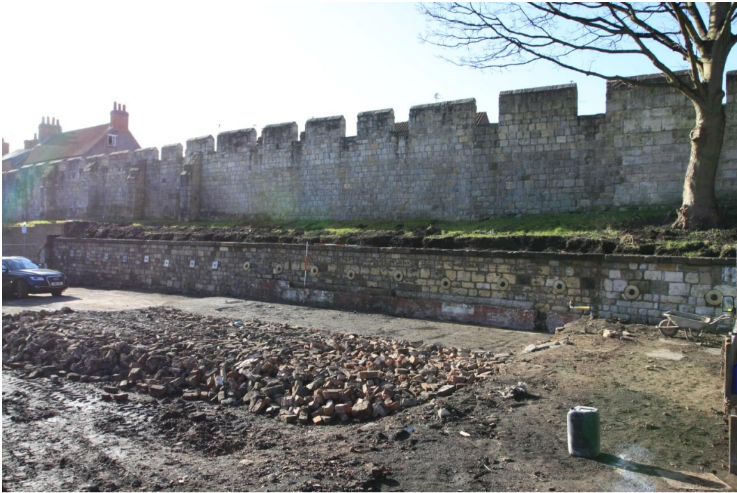
33. South facing view of the retaining wall. Scale units 0.5m
