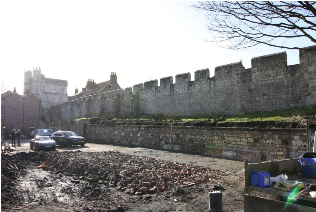
23. South facing view of the retaining wall. Scale units 0.5m
