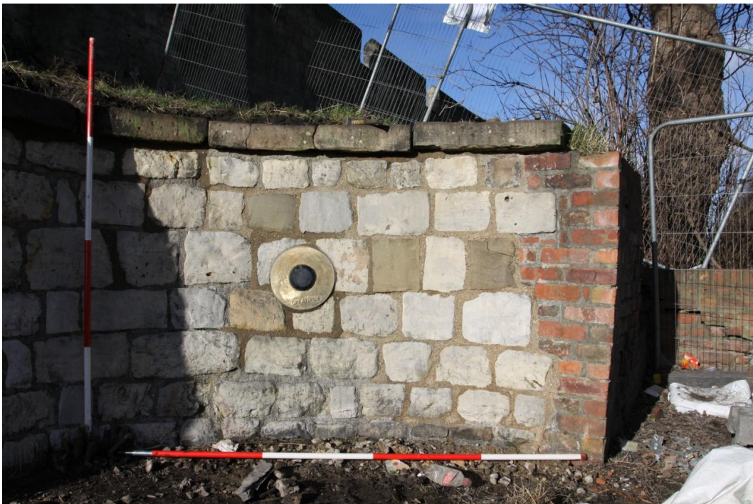
16. West facing view of the retaining wall. Scale units 0.5m
