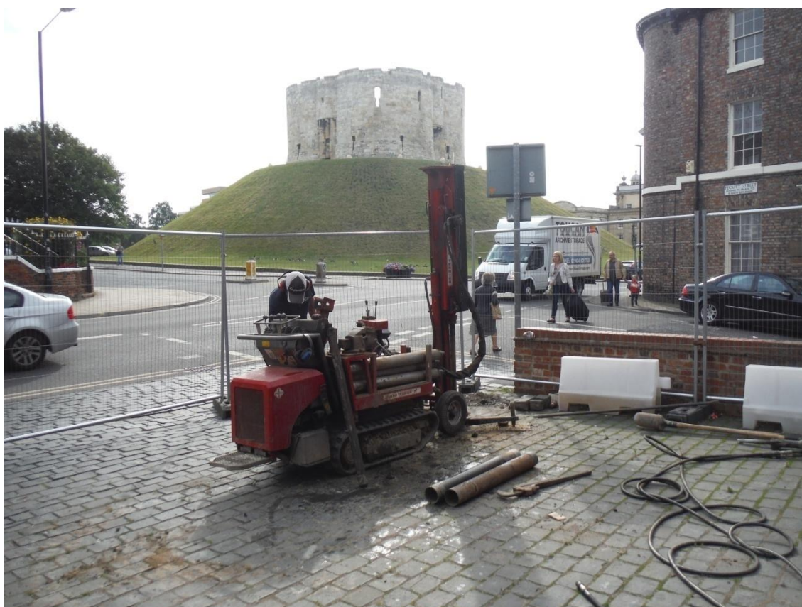
Plate 10 Borehole 1 during drilling
