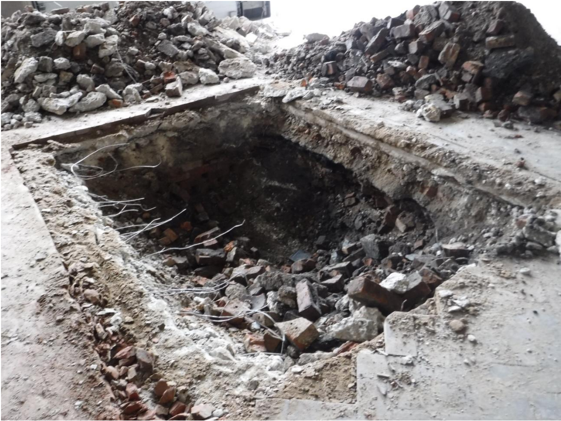
Plate 3 Trench 2 general view, looking east
