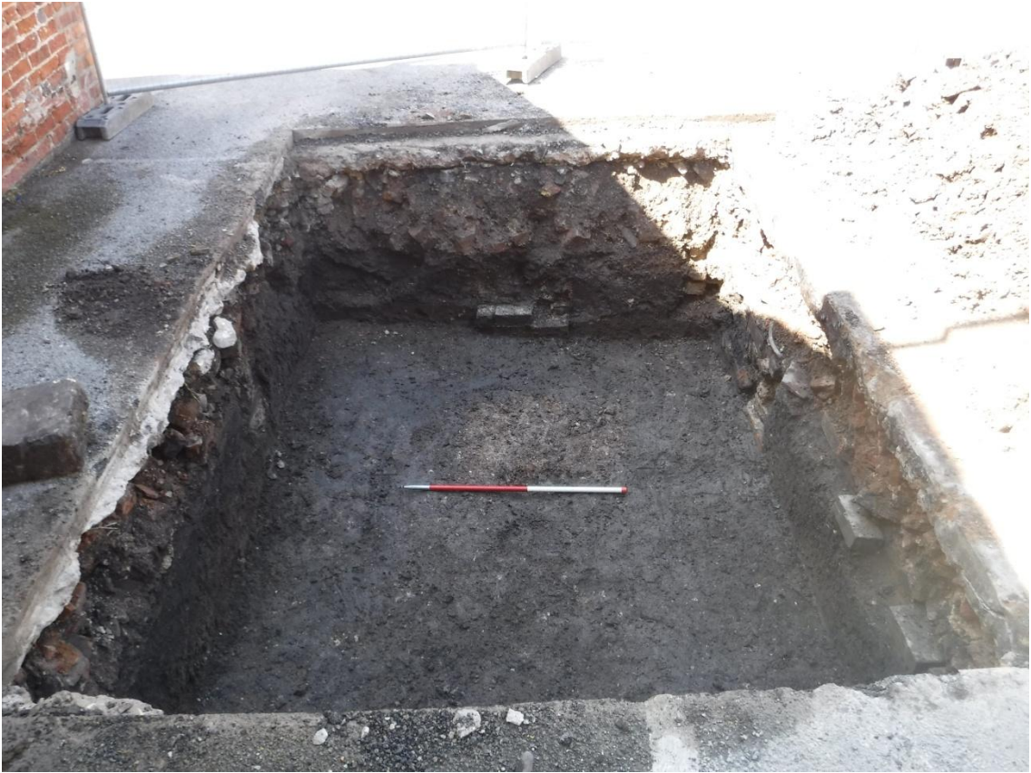
Plate 5 Trench 3 general view looking SW
