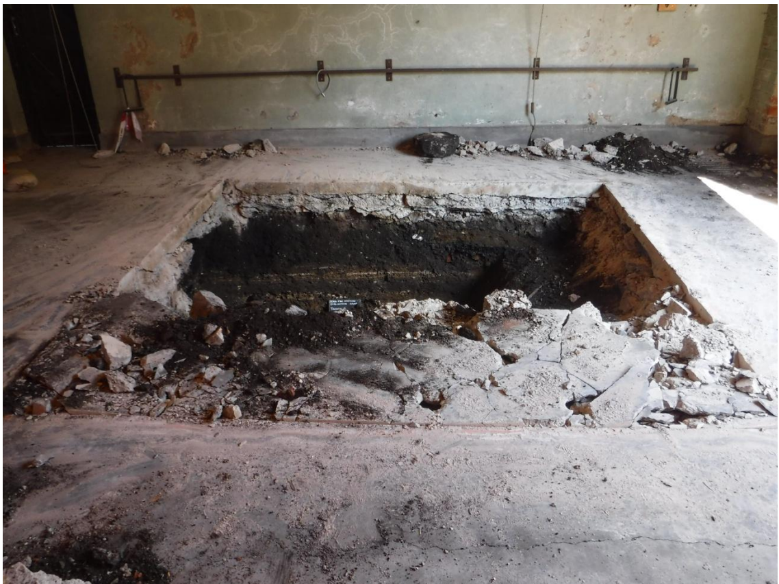
Plate 8 Trench 4 general view looking NE
