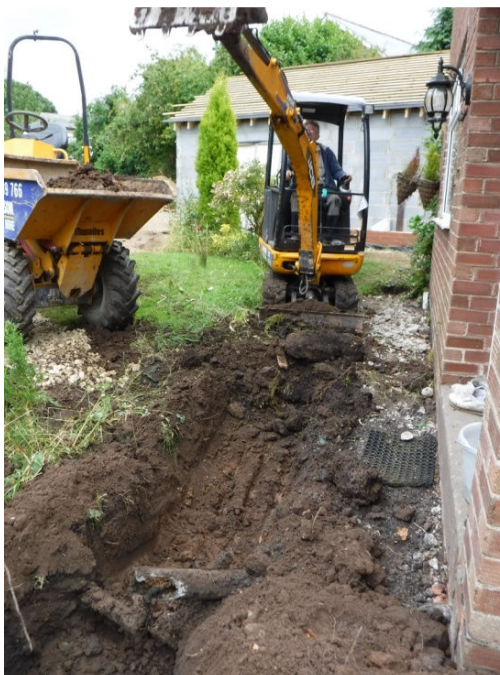
Plate 9 Excavation of Trench D facing north-east.
