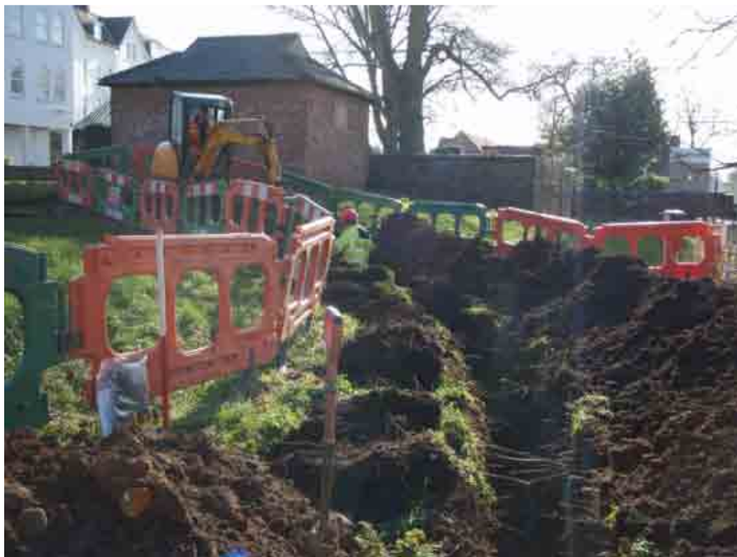
Plate 8 Trench 5 on approach to electric substation, Looking S
