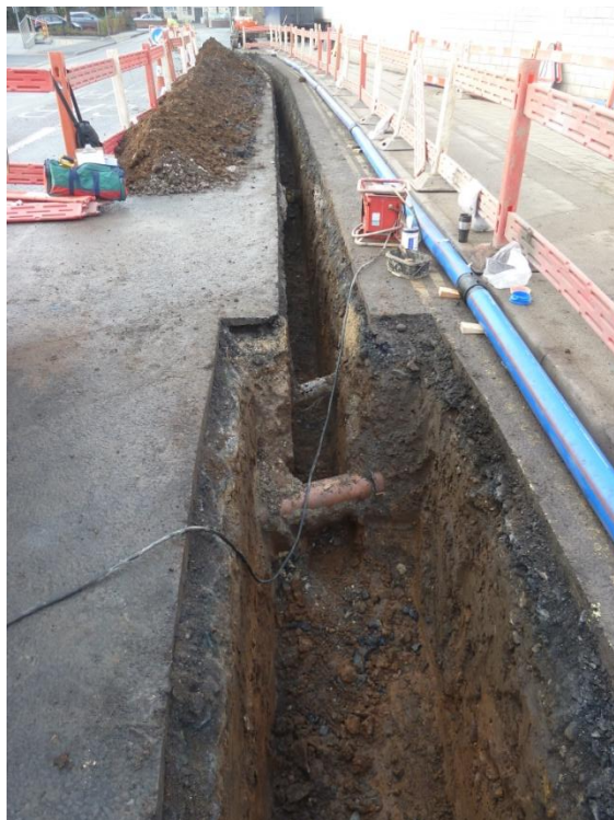
Plate 4. Utility trench looking W
