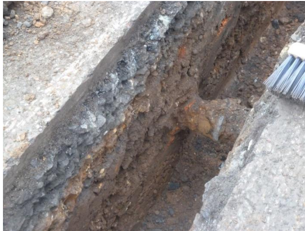
Plate 3. Iron pipework exposed in utility trench
