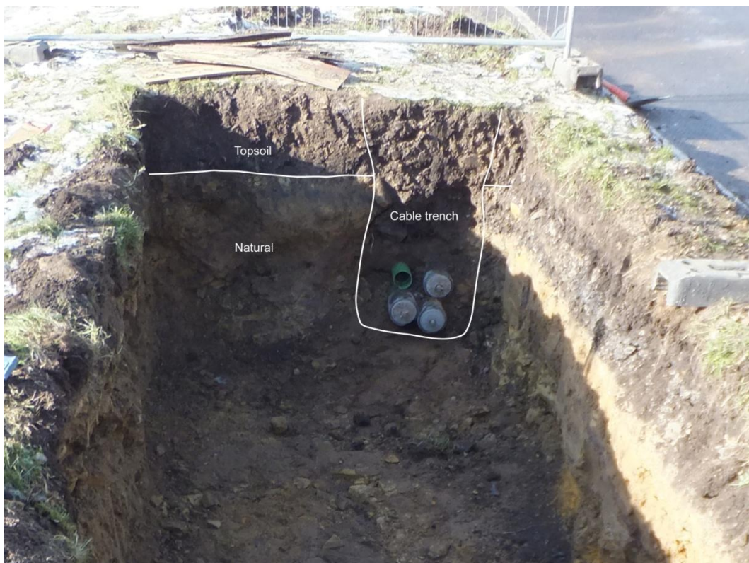
Plate 6 Joint bay 15, facing west.
