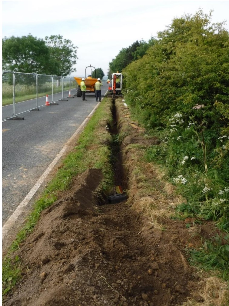
Plate 2 General view of trench at SAM 1021100, East Toft Dyke, facing south.
