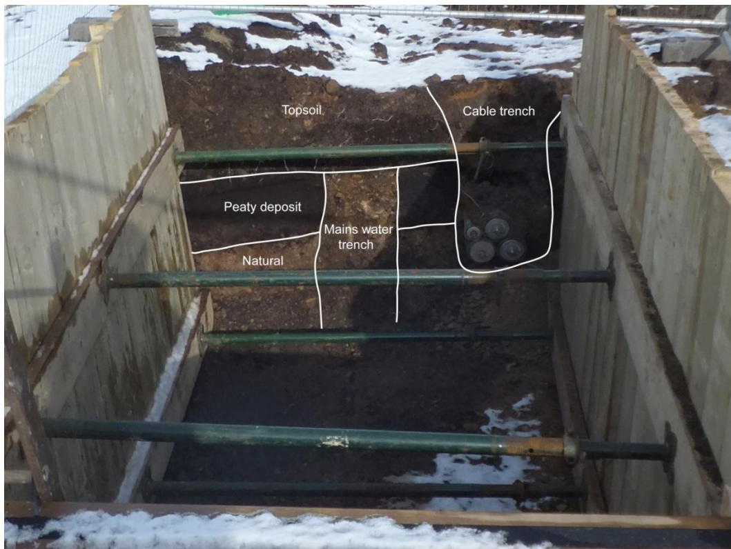
Plate 5 Joint bay 14, facing north.
