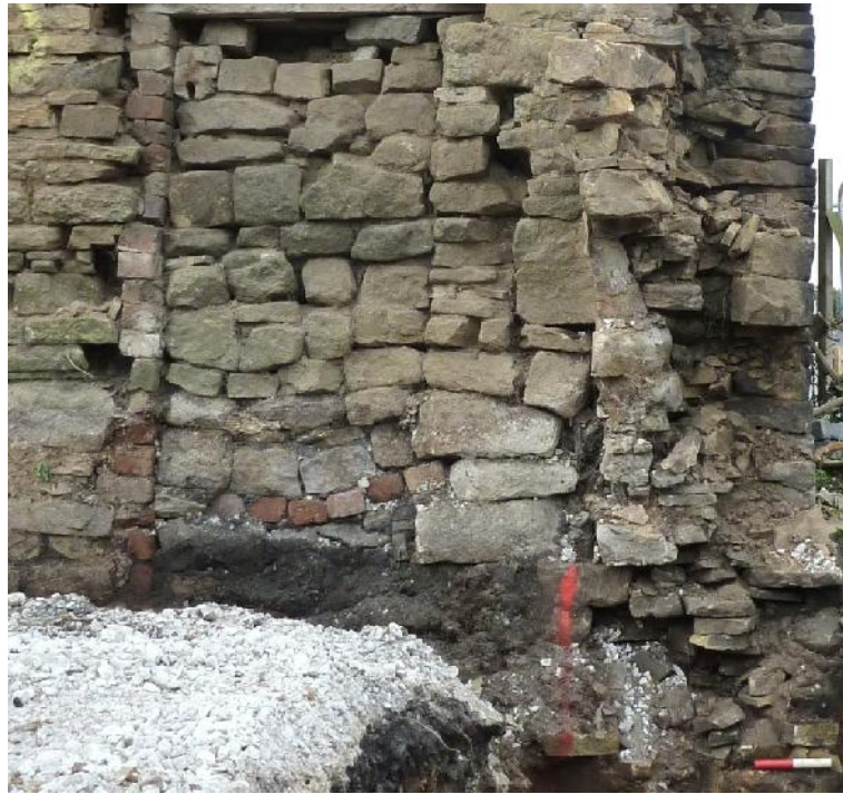
Plate 6 Elevation showing remains of western wall of Building 6/7 at north-west corner of Building 7 (far right). 0.10m scale divisions.
