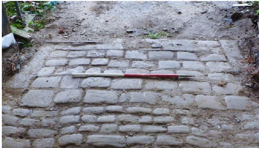
Plate 3 Detail showing larger setts and stone surround at southern entrance.
