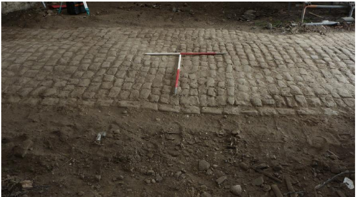
Plate 5 Record shot showing kerbstones along western edge (foreground) and buckled, rutted surface away from southern entrance. Looks east-south-east. 0.5m scale divisions.
