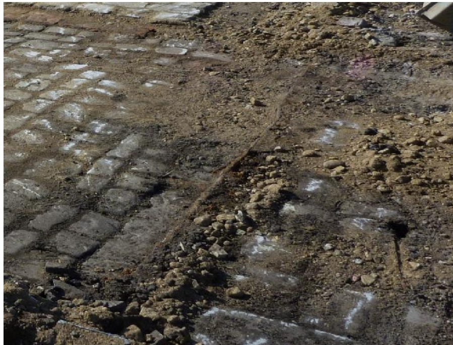
Plate 11 Building 6, record shot of iron door runner (bottom left – top right) after blocking removed. Looks south-east.
