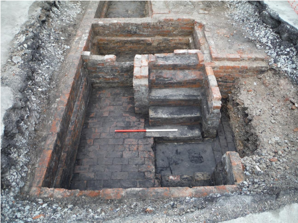
Plate 10. North-west facing view of the Leeds Arms coal cellar (set 213, 1.00m scale)
