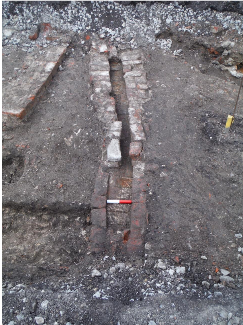
Plate 6. North-west facing view of brick culvert Set 107 (0.20m scale)
