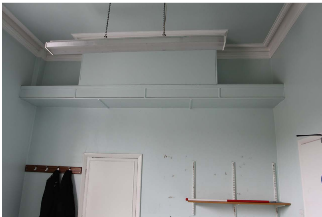
Plate 11: Room 10 former chimneystack north wall
