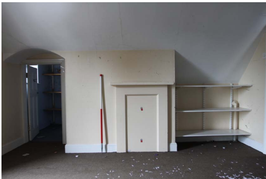
Plate 12: Room 16, south wall
