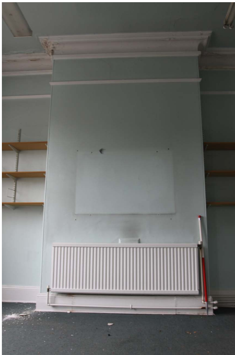
Plate 10: Room 8, chimneystack, cornice and picture rail to north wall
