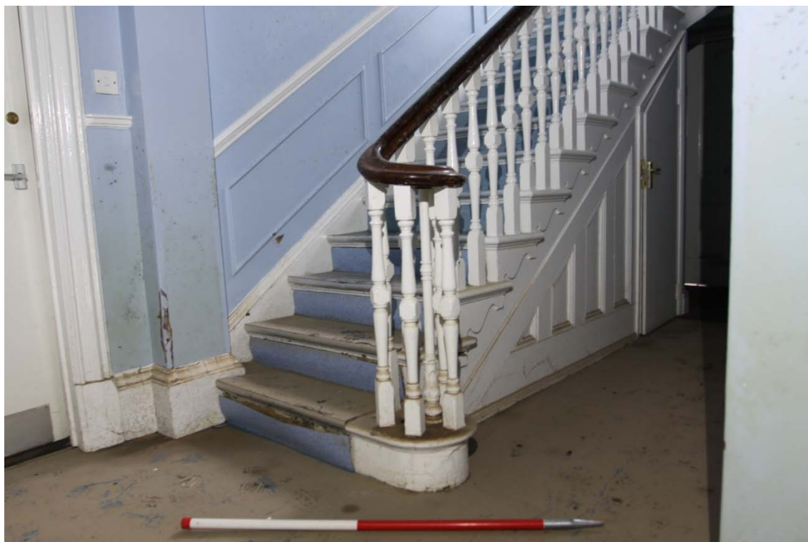
Plate 5: Room 5, staircase and hallway
