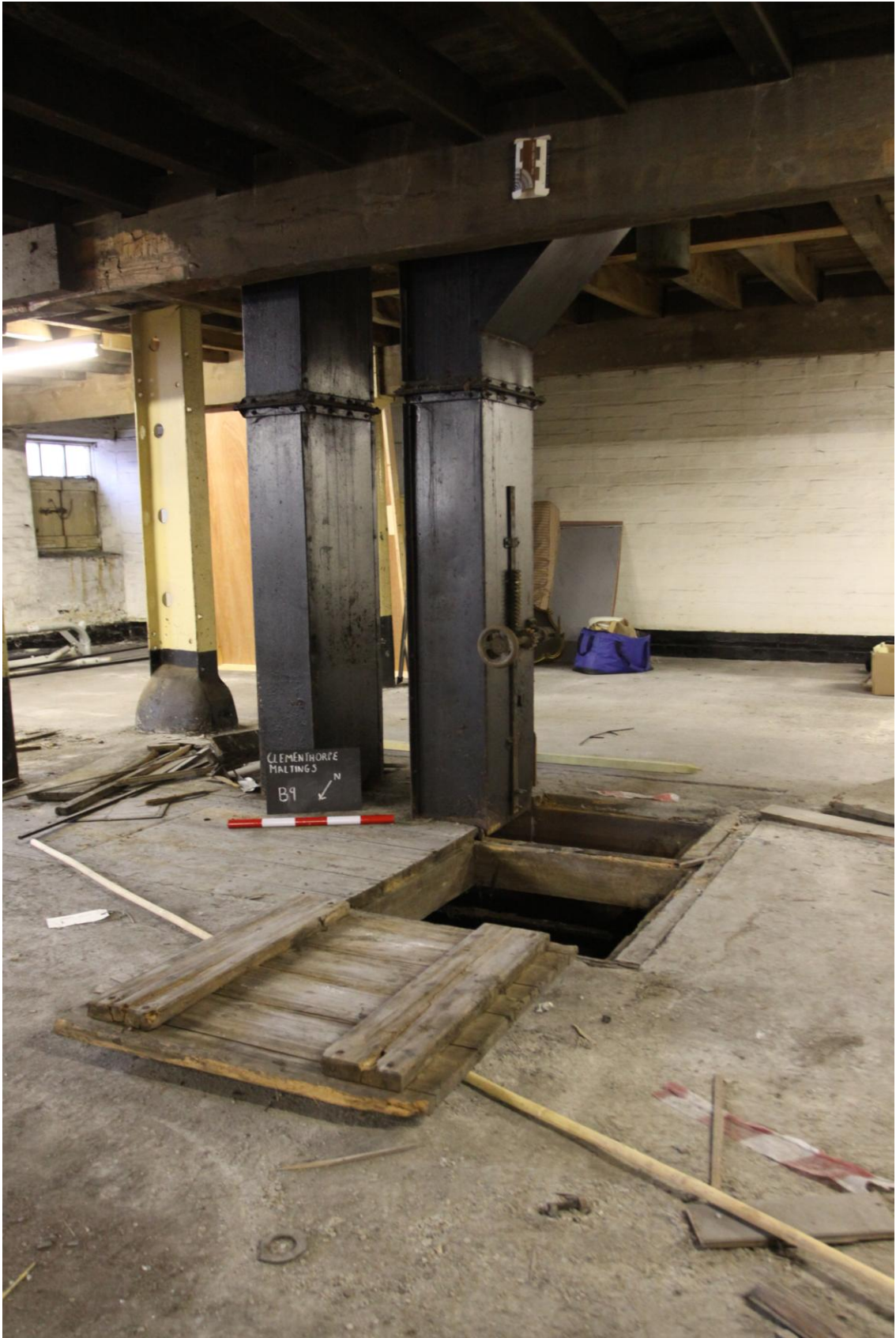
Plate 33: Double Bucket Elevator, Ground Floor Level (Photograph 81).
