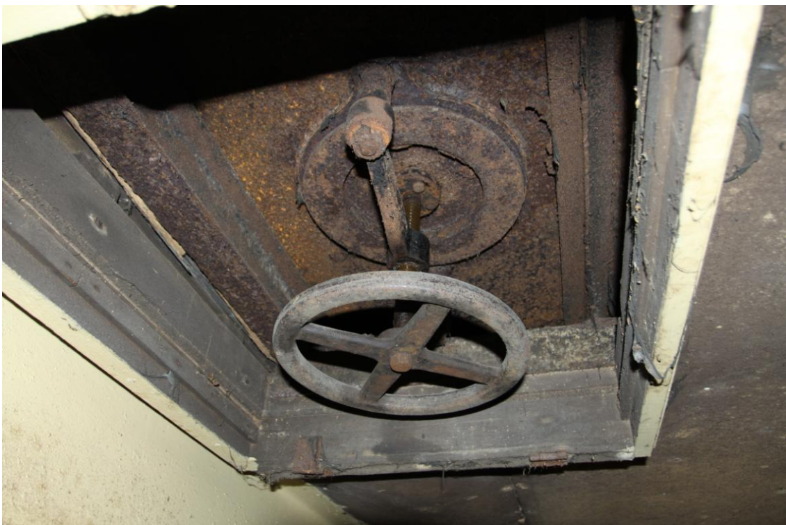
Plate 32: Hatches to Underside of Steeping Cistern (Photograph 66).
