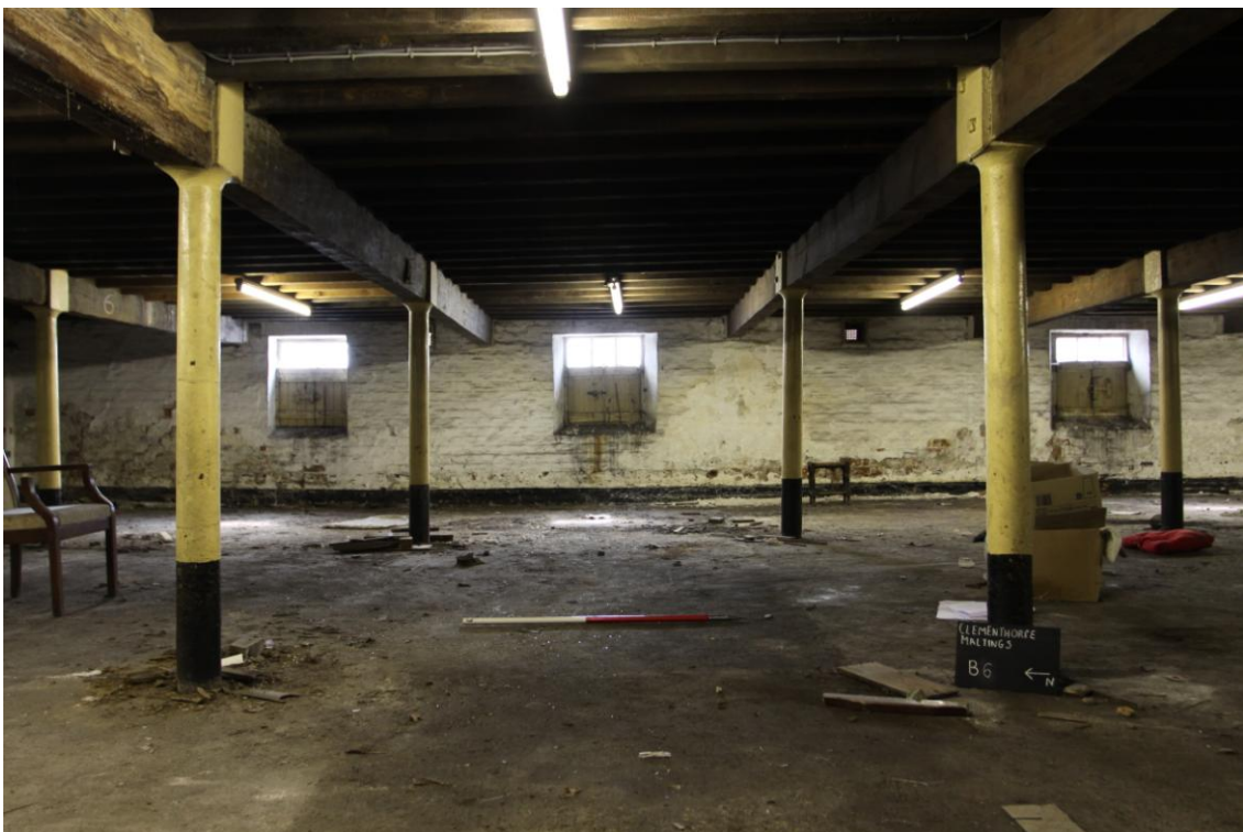
Plate 22: Windows to East Wall, Ground Floor Level (Photograph 21).
