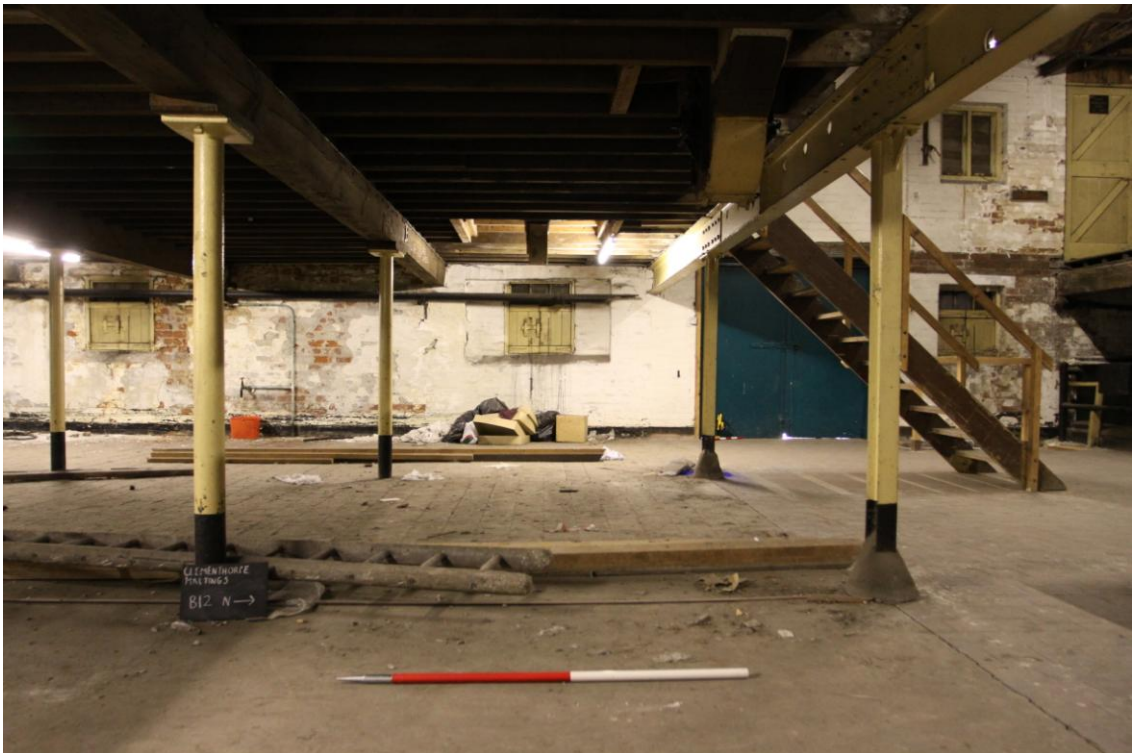
Plate 28: Continuation of Water Inlet Pipe along West Elevation, 1 st Floor Level (Photograph 127).
