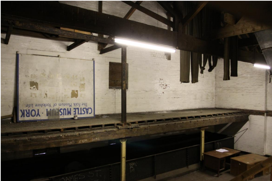
Plate 31: 3 rd Floor Level showing grain holes above Steeping Cistern (Photograph 167).
