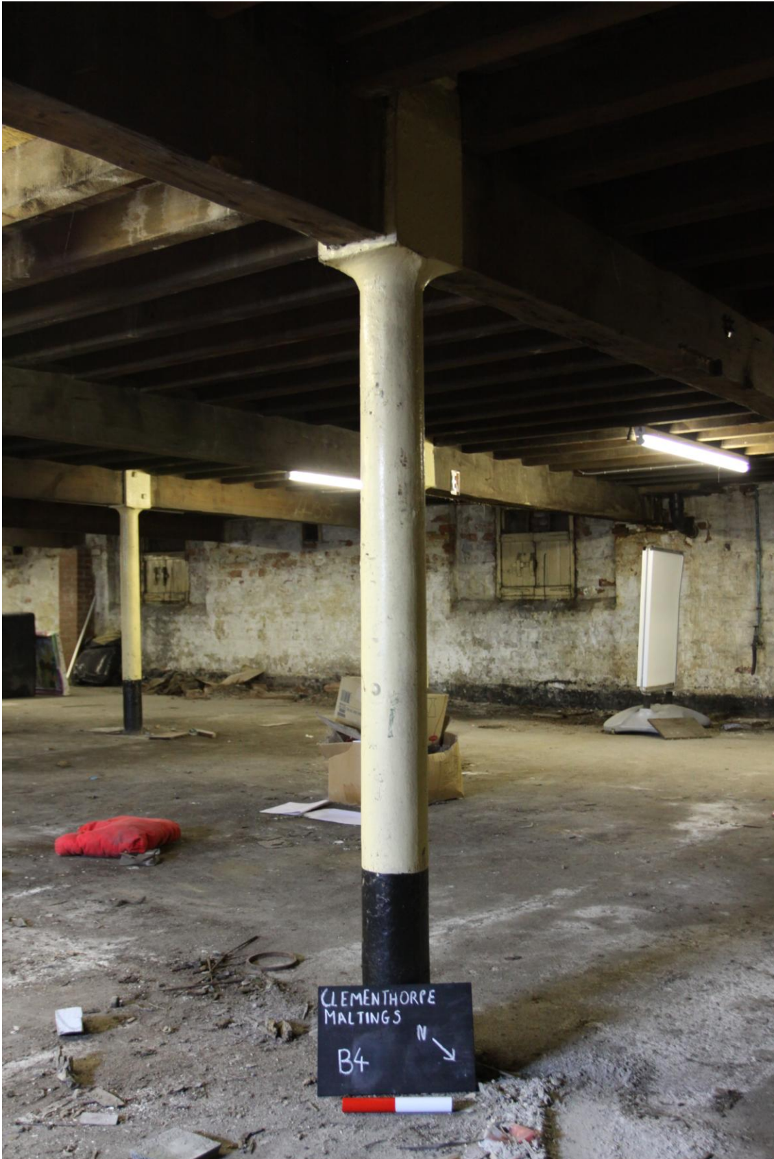
Plate 19: Cast Iron Column, Ground Floor Level (Photograph 72).
