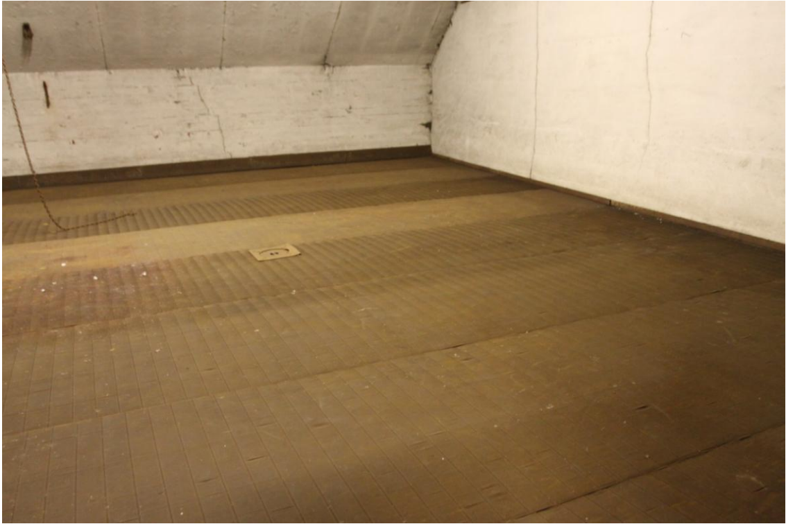
Plate 10: 3 rd Floor Level Kiln Drying Floor (Photograph 217).
