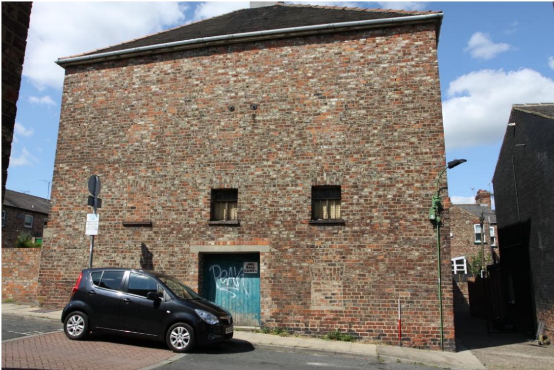
Plate 1: South elevation of Kiln (Photograph 234).
