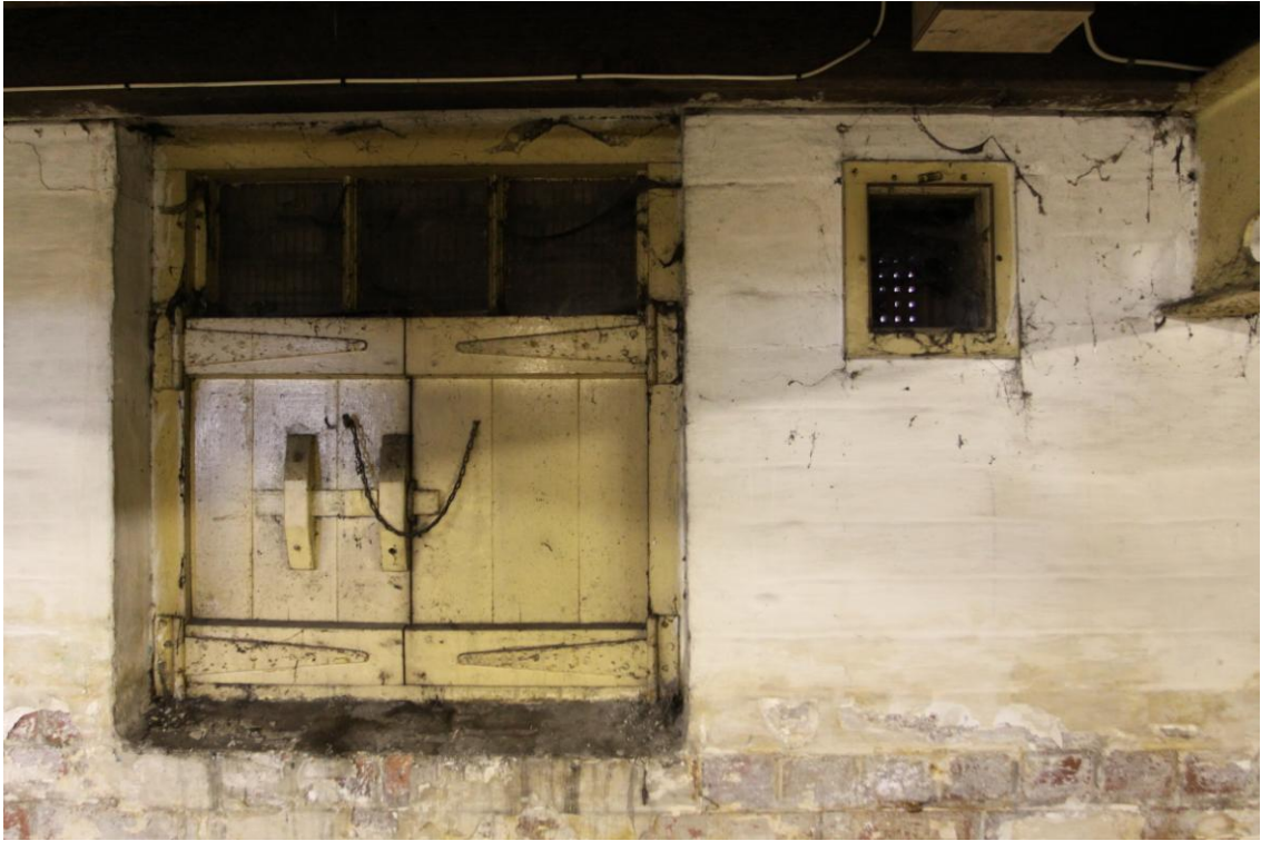
Plate 23: Window and Ventilation Hole Detail Ground Floor Level (Photograph 77)
