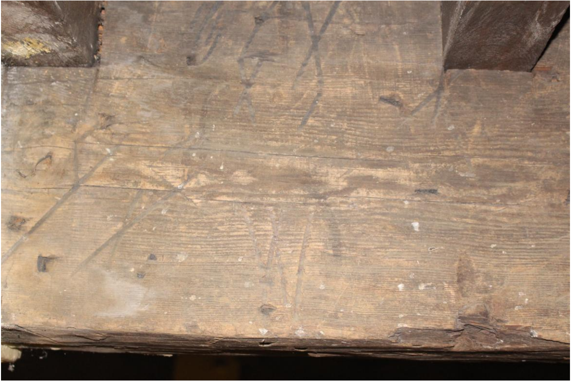
Plate 44: Baltic Timber marks to left of "W.F.No2H" (© Mark Sissons).
