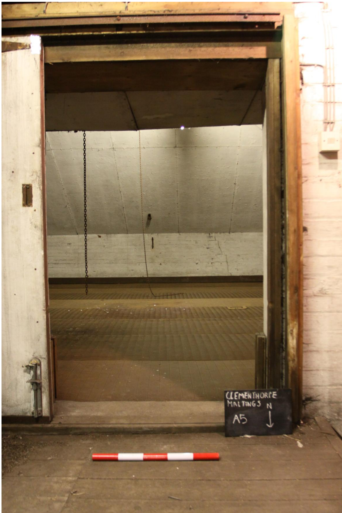
Plate 12: 3 rd Floor Level Doorway into Kiln (Photograph 214).
