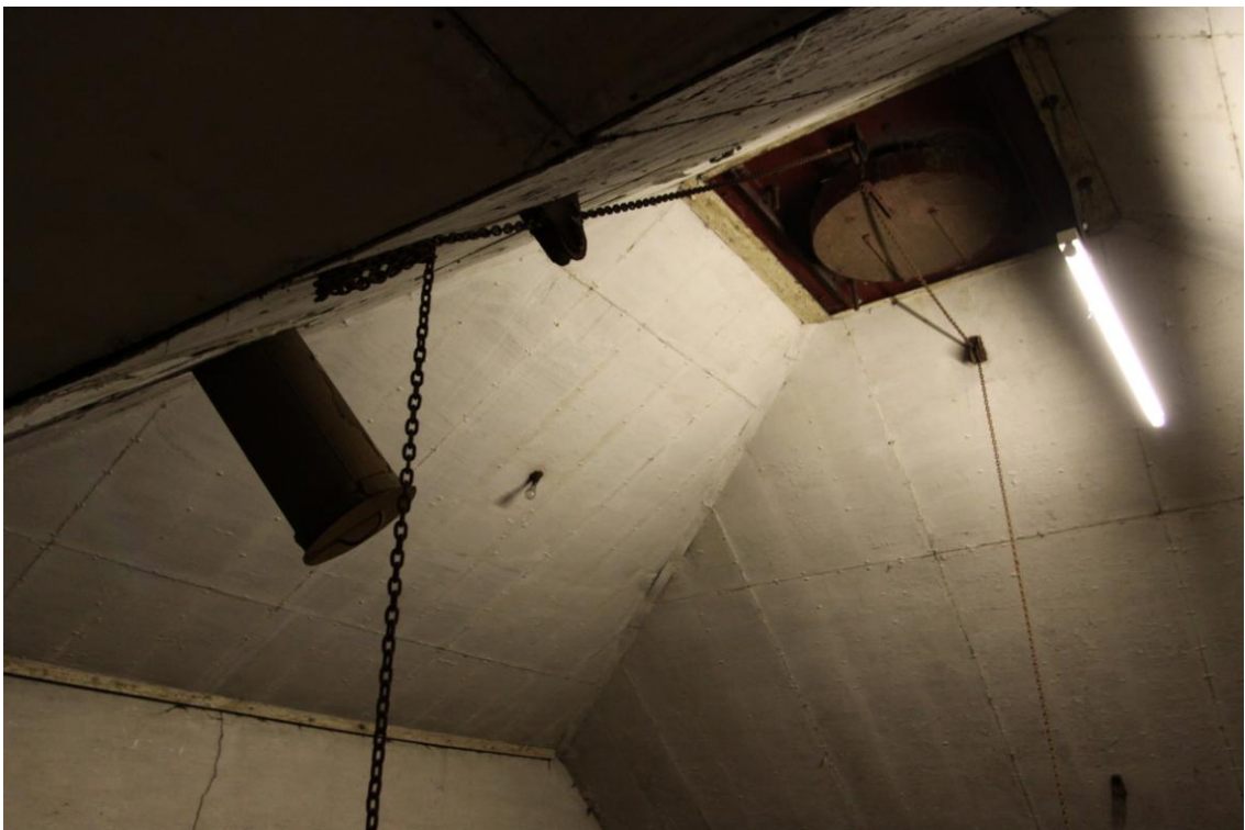
Plate 11: 3 rd Floor Level Kiln Roof (Photograph 216).
