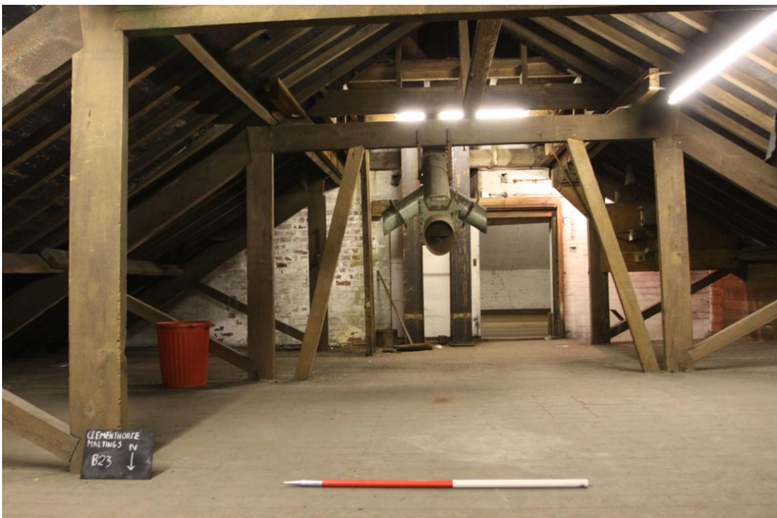
Plate 35: 3 rd Floor level showing pipes attached to Double Bucket Elevator (Photograph 207).
