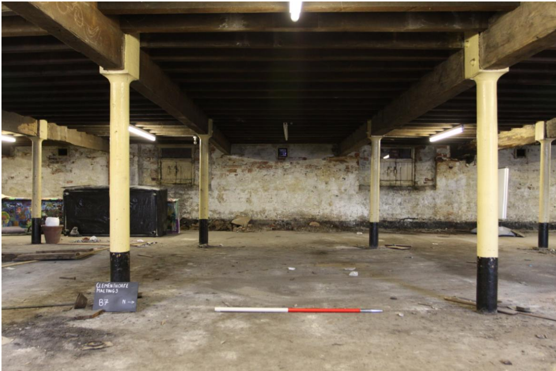
Plate 21: Windows to West Wall, Ground Floor Level (Photograph 43).
