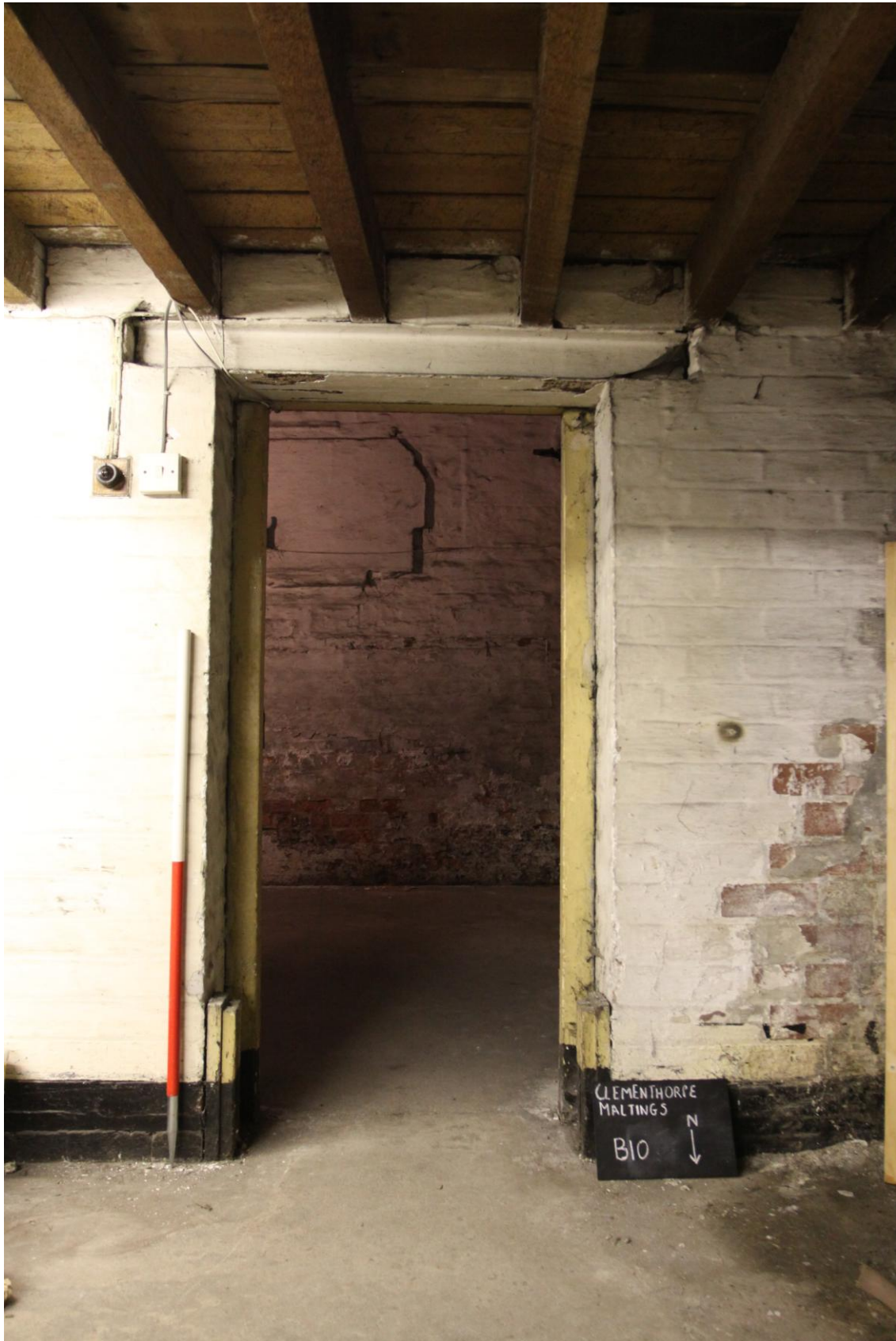
Plate 7: Doorway between Kiln and Malthouse (Photograph 89).
