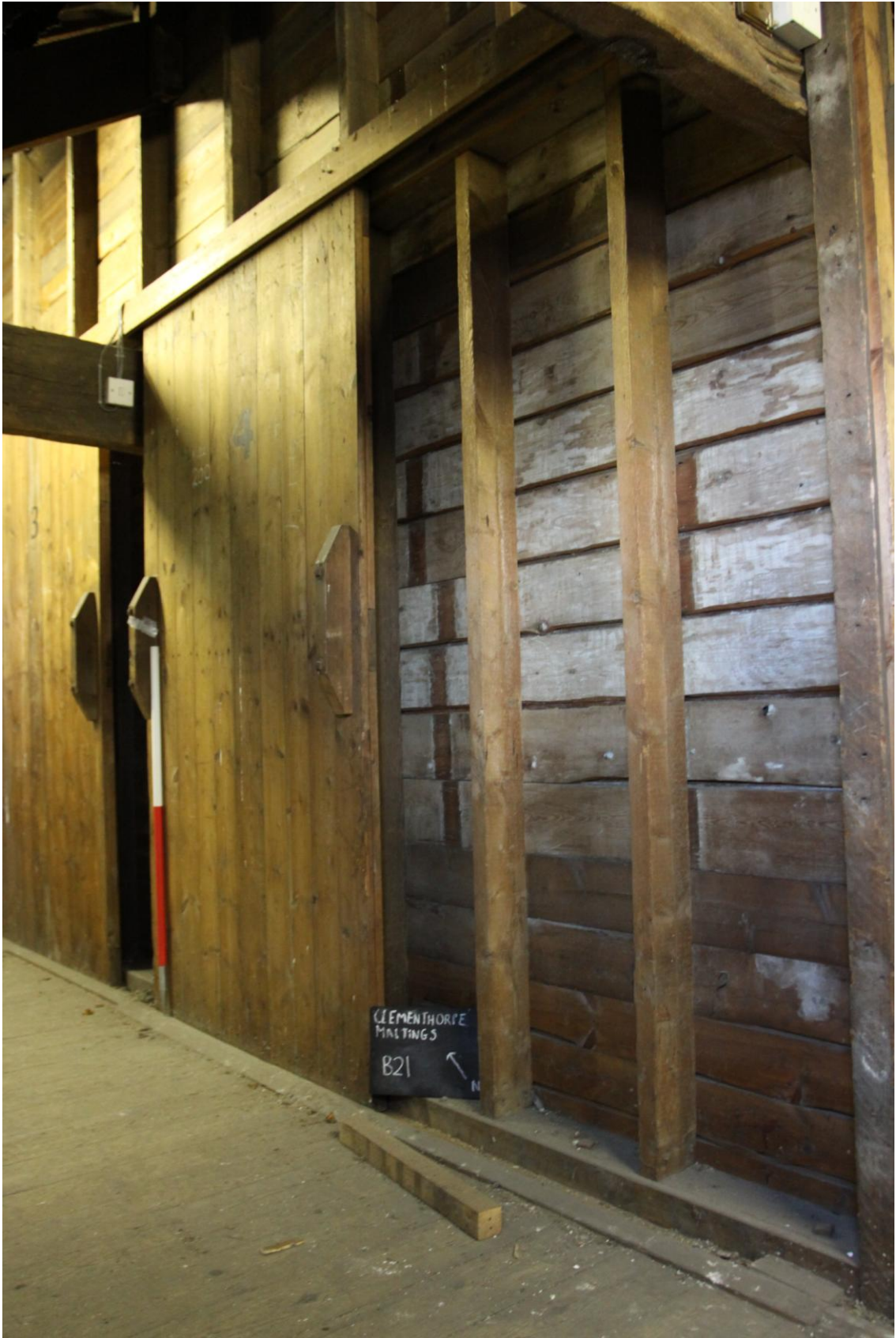
Plate 41: Storage Bins 2 nd Floor Level (Photograph 192).
