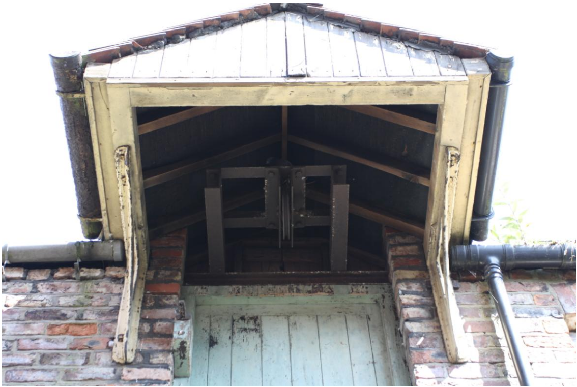
Plate 16: Hoist Door, Detail of Hoist Mechanism (Photograph 229).
