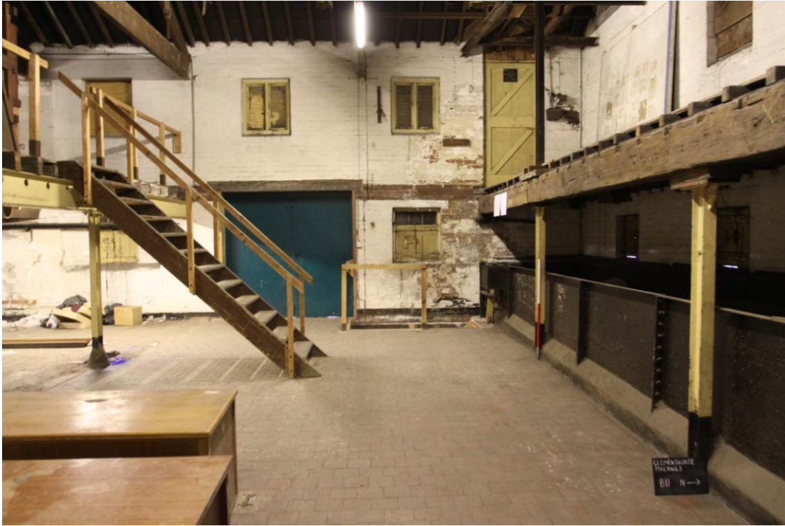
Plate 25: Removed Section of Floor at 2 rd Floor Level (Photograph 125).
