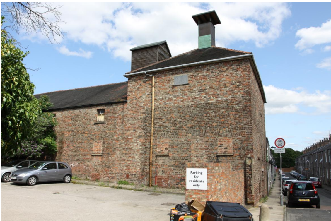
Plate 2: West Elevation of Kiln (Photograph 245).
