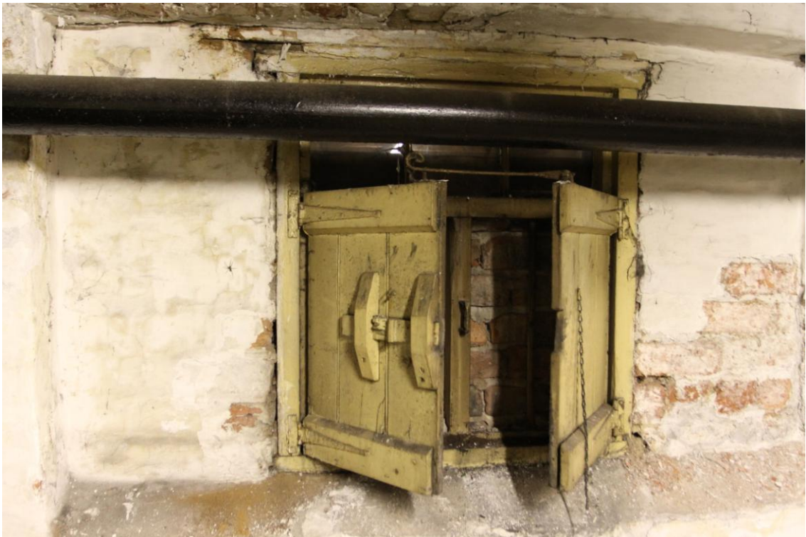
Plate 24: Window Detail 1 st Floor Level (Photograph 145).
