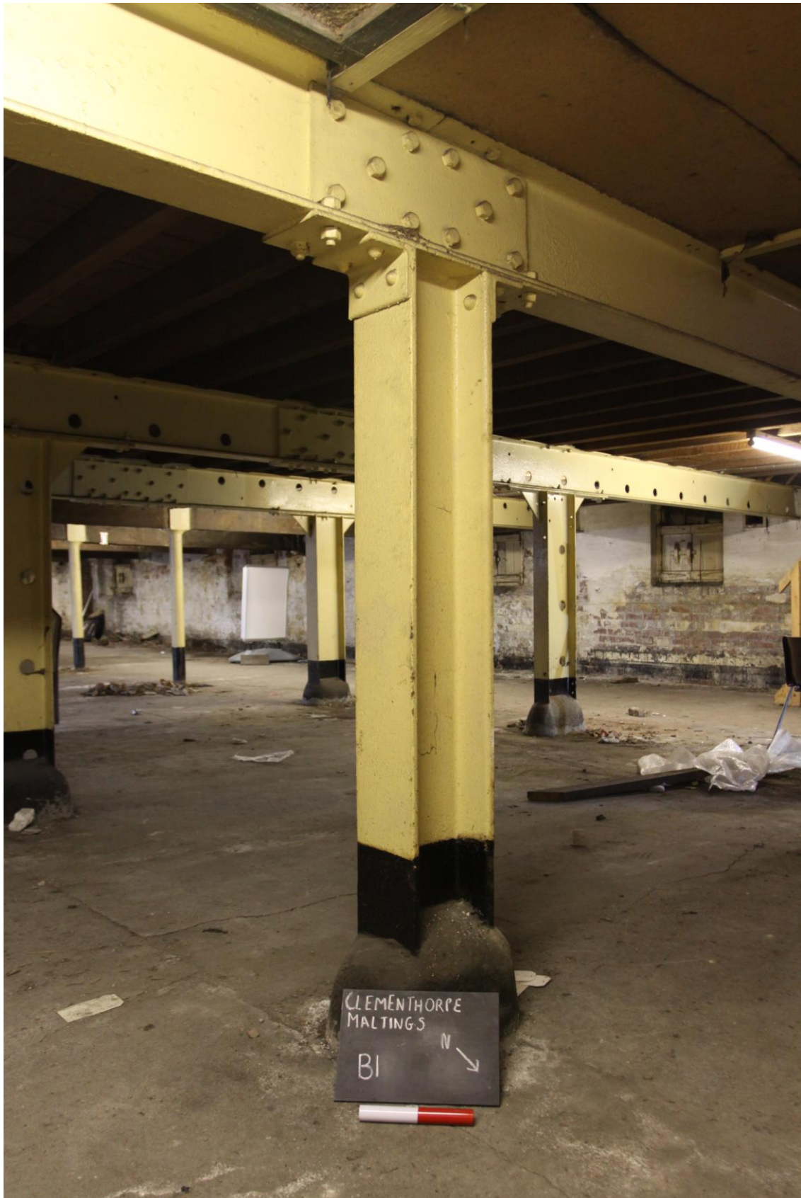
Plate 20: H-shaped Girder, Ground Floor Level (Photograph 68).
