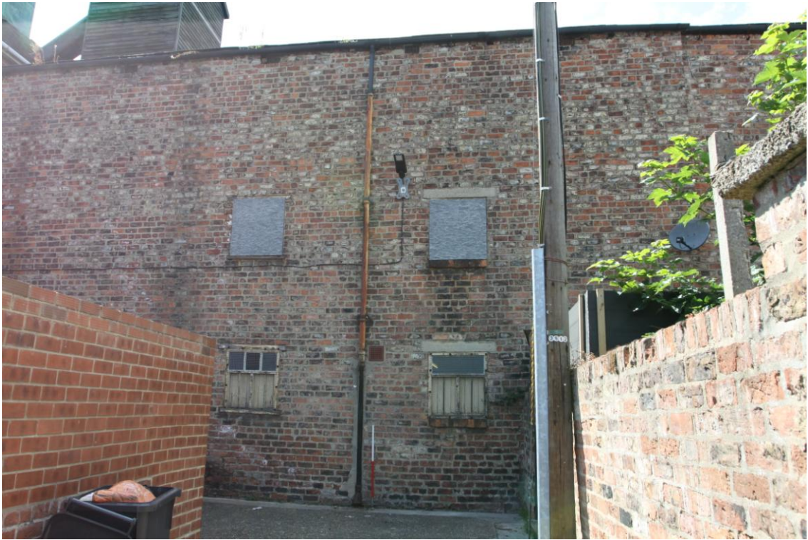
Plate 14: East Elevation malthouse, Window Details (Photograph 240).
