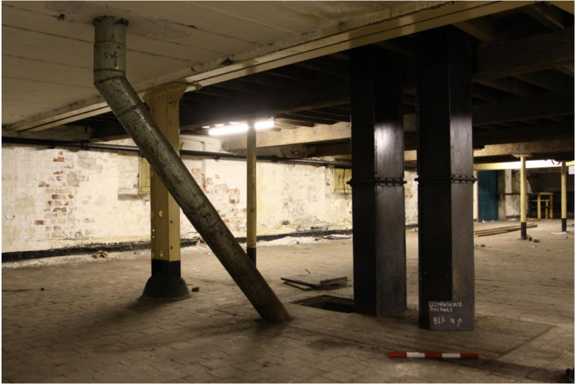
Plate 36: Pipework to the south end of the Malthouse (Photograph 139).
