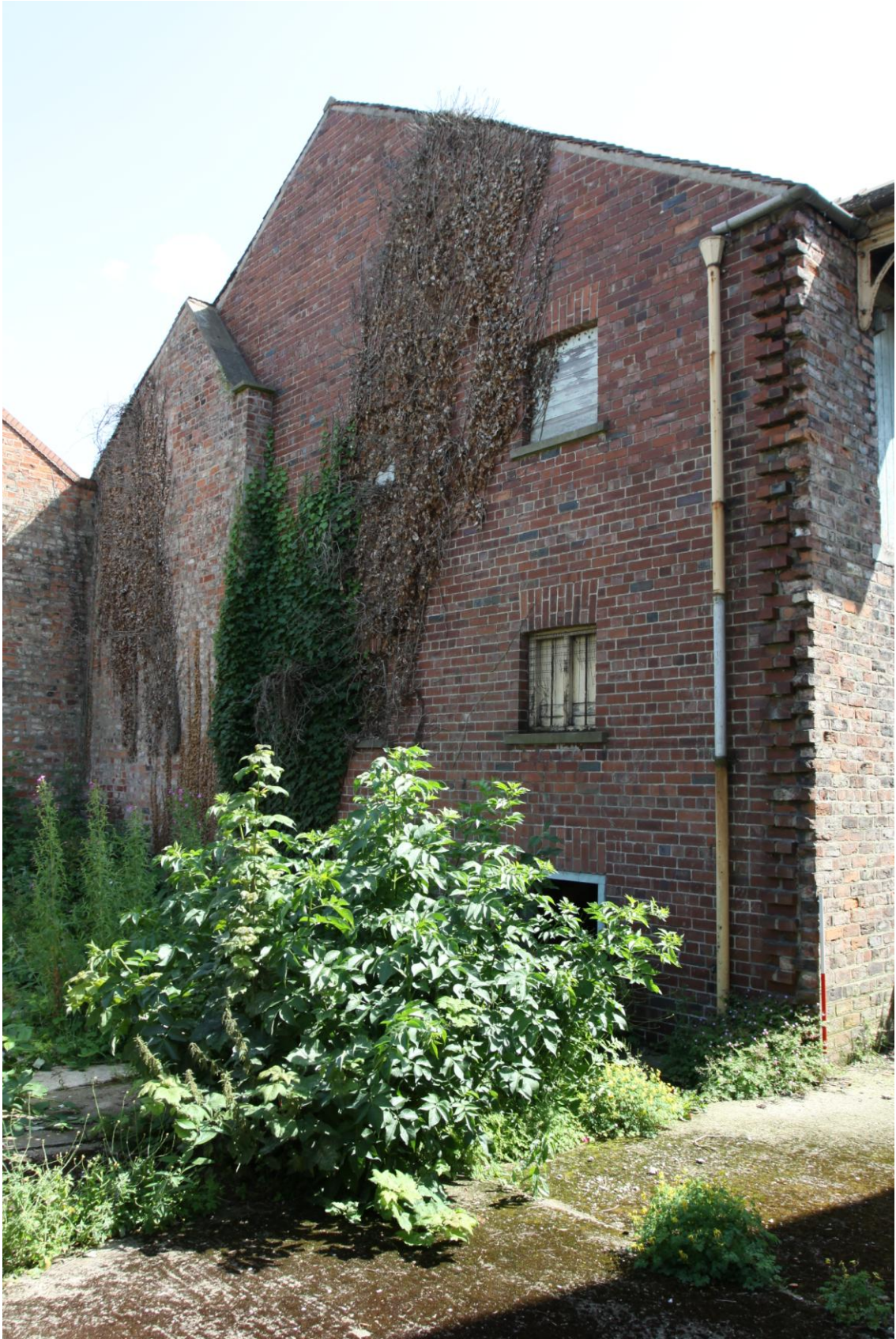
Plate 17: North Elevation of Malthouse (Photograph 220).
