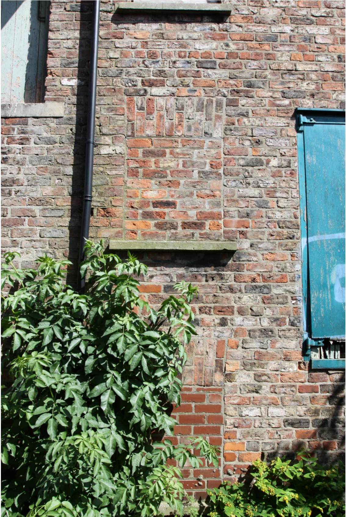
Plate 13: West Elevation Malthouse, Window Details (Photograph 230).
