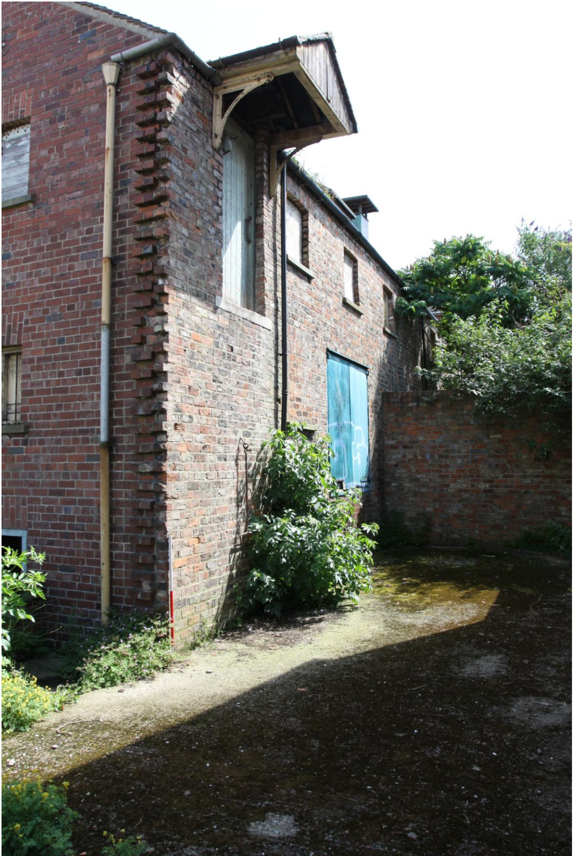
Plate 15: West Elevation Malthouse, Hoist Door (Photograph 227).
