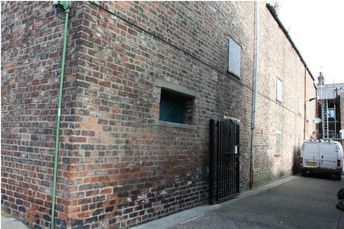
Plate 3: East Elevation of Kiln (Photograph 4).
