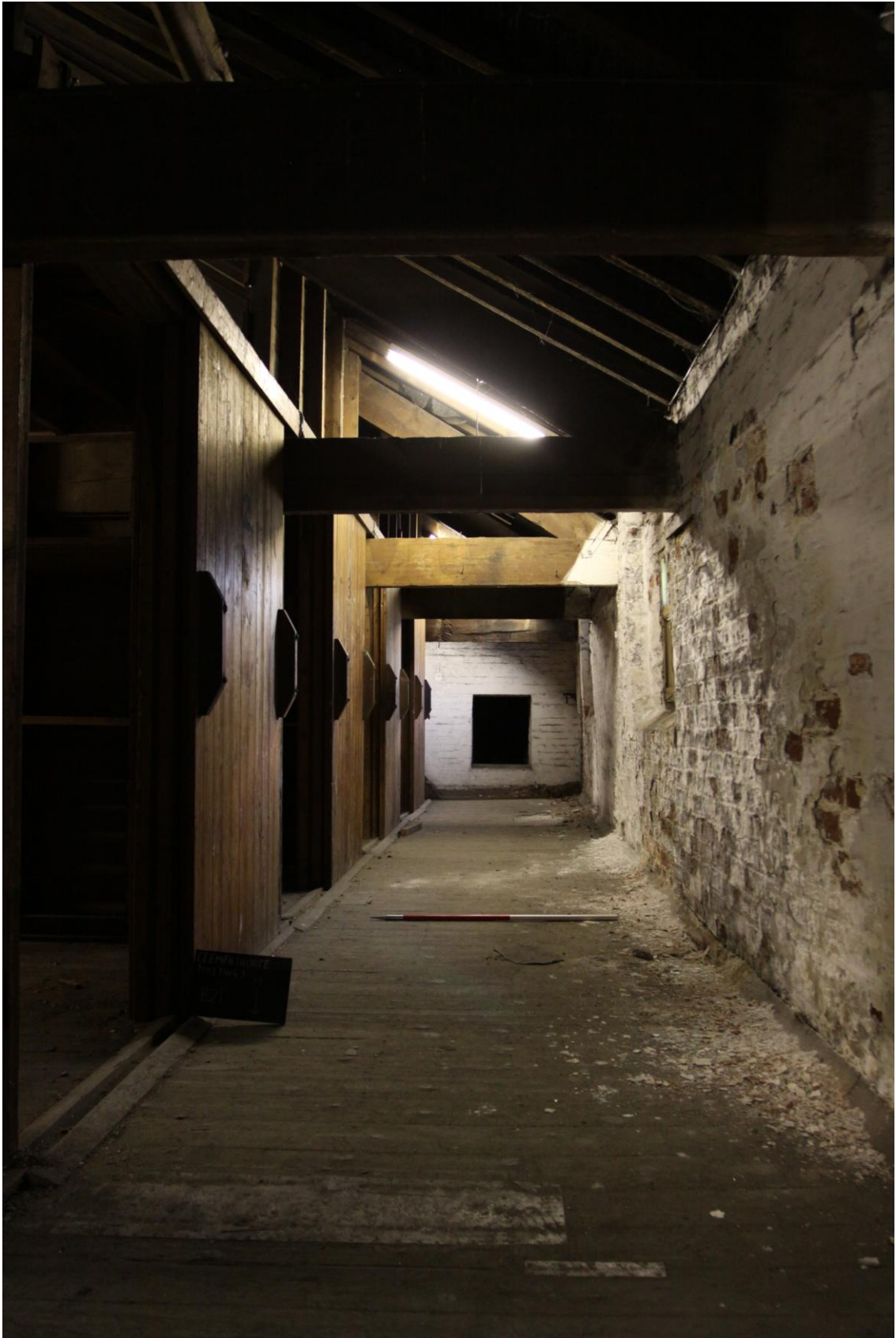
Plate 40: 2 nd Floor Level, Corridor and Storage Bins (Photograph 187).
