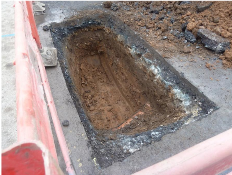
Plate 1: Hydrant pit looking SE.
