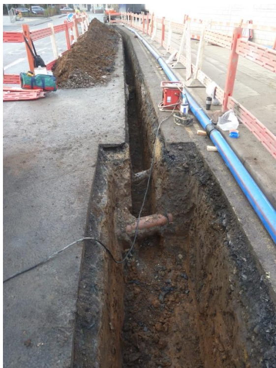
Plate 4. Utility trench looking W
