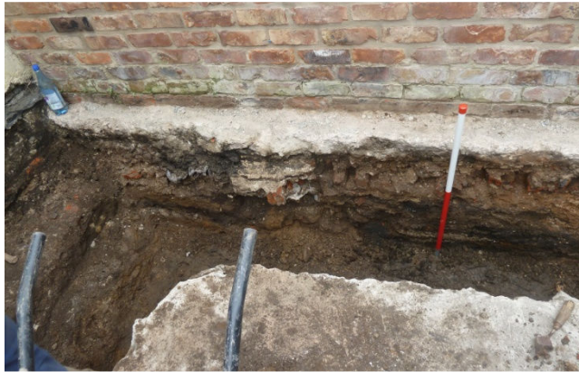
Plate 9. North footing trench, South facing section. West end. Scale 1m
