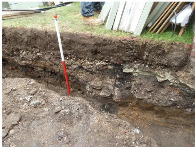
Plate 4. South footing trench, North facing section- middle of section. Scale 1m
