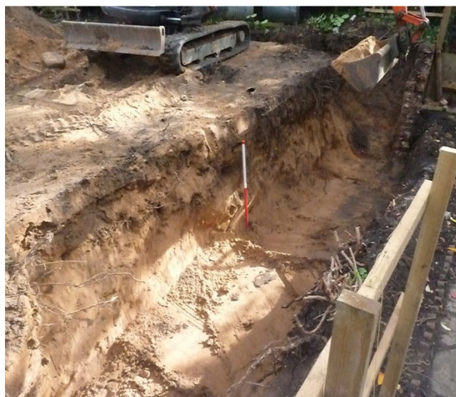
Plate 3. West footing trench under excavation looking SE. Scale 1m
