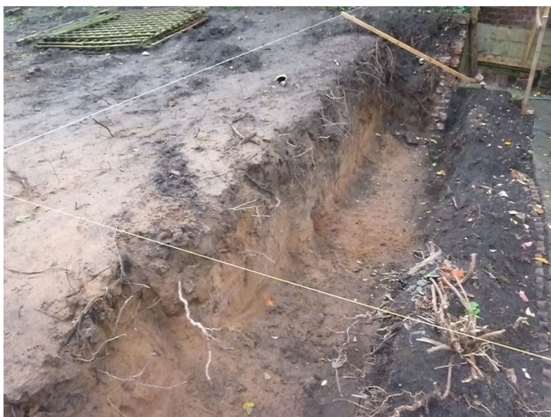
Plate 1: West footing trench as seen on arrival, looking SSE
