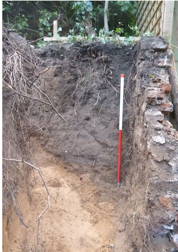
Plate 4. Intersection of South and West footing trenches looking S. Scale 1m
