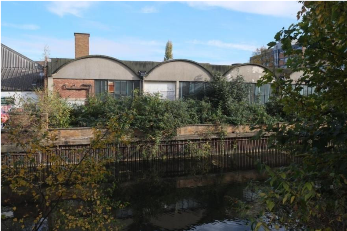
Plate 5 River Foss frontage showing river wall
