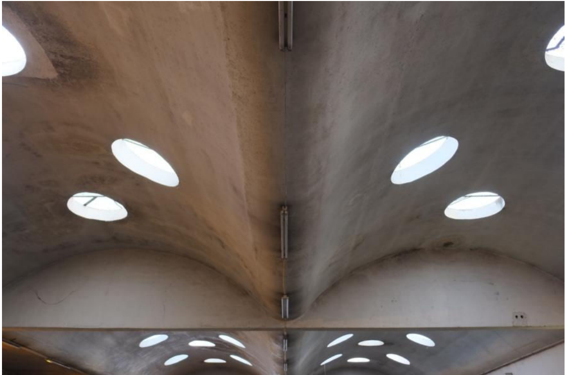
Plate 3 Roof structure with circular portal sky-lights
