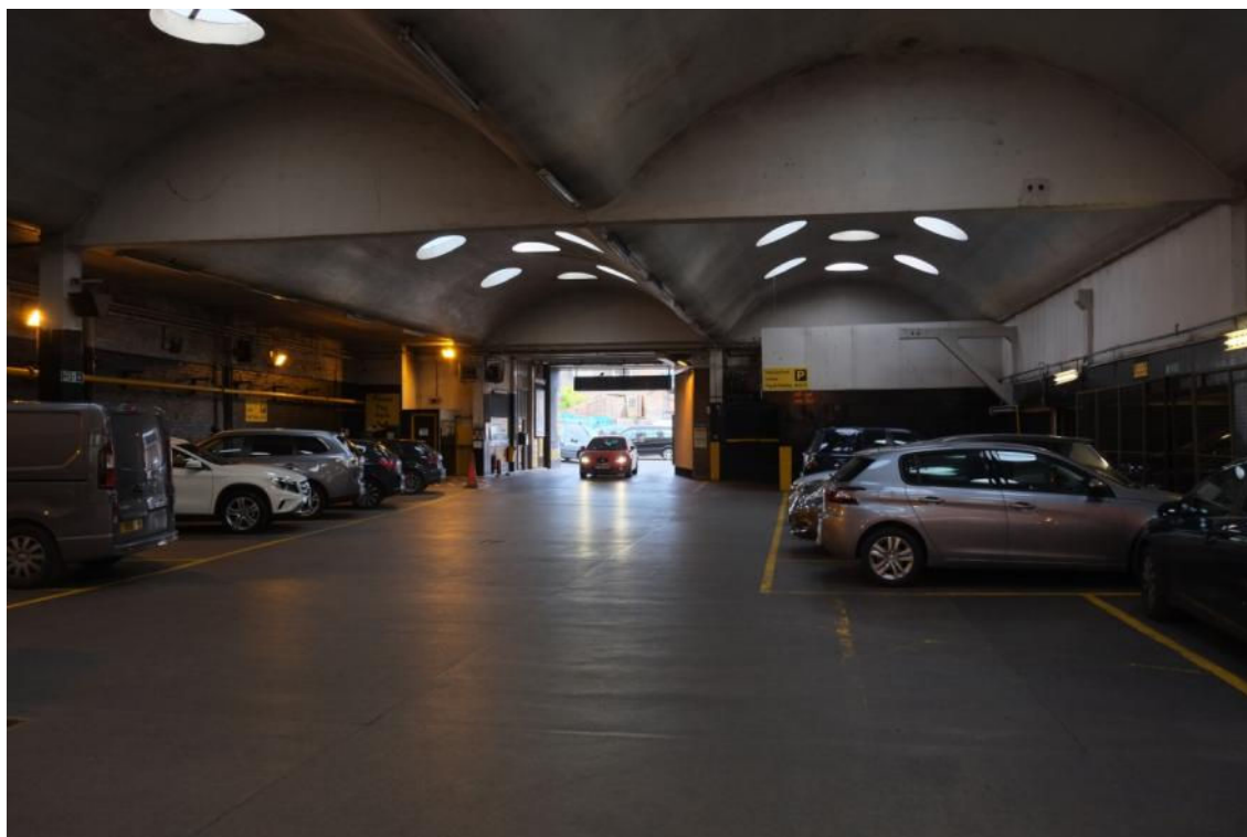
Plate 2 Entrance to Car Park
