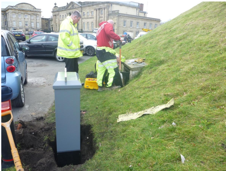
Plate 1 New feeder pillar in foreground, also showing excavation underway around existing feeder pillar
