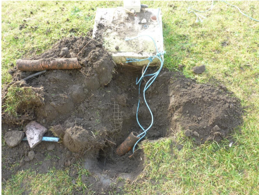
Plate 5 Plinth 12, showing excavation to expose and access the existing duct, note the nylon mesh also found next to the majority of other plinths.
