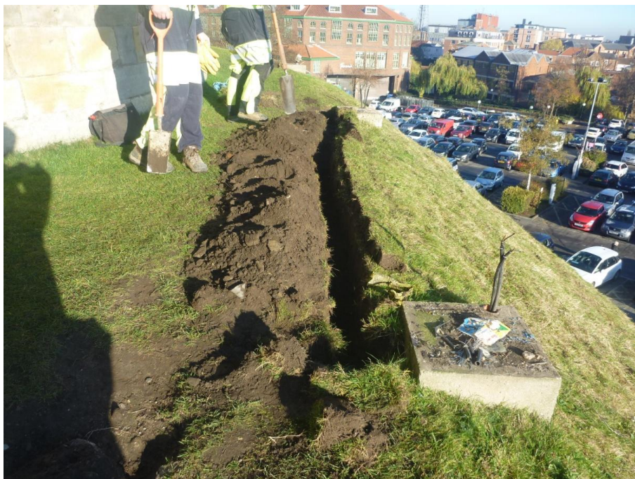
Plate 2 First section of cable trench running north-east from light plinth 1
