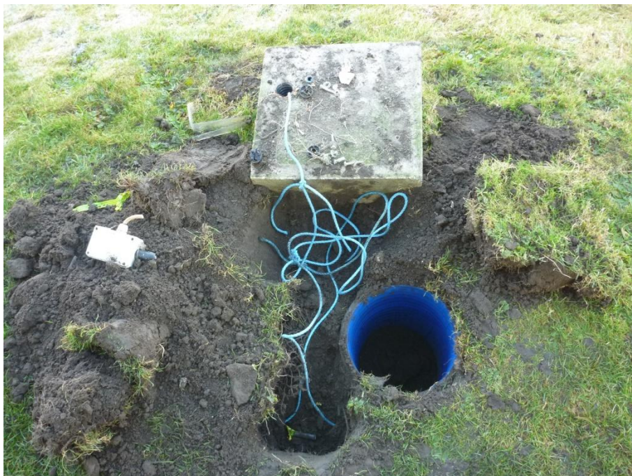
Plate 6 Plinth 4 and blue plastic sleeve in geotechnical inspection pit
