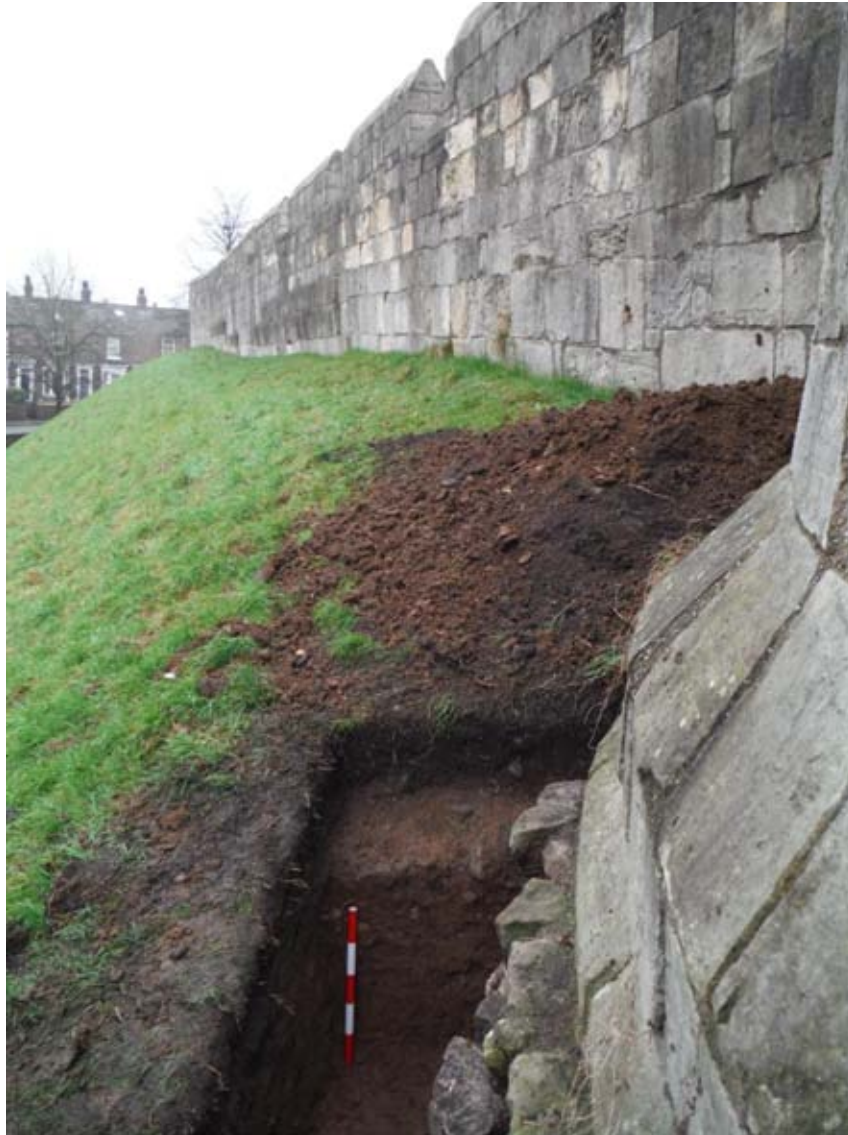
Plate 19. West facing view of Trial Pit 7 (0.50m scale).
