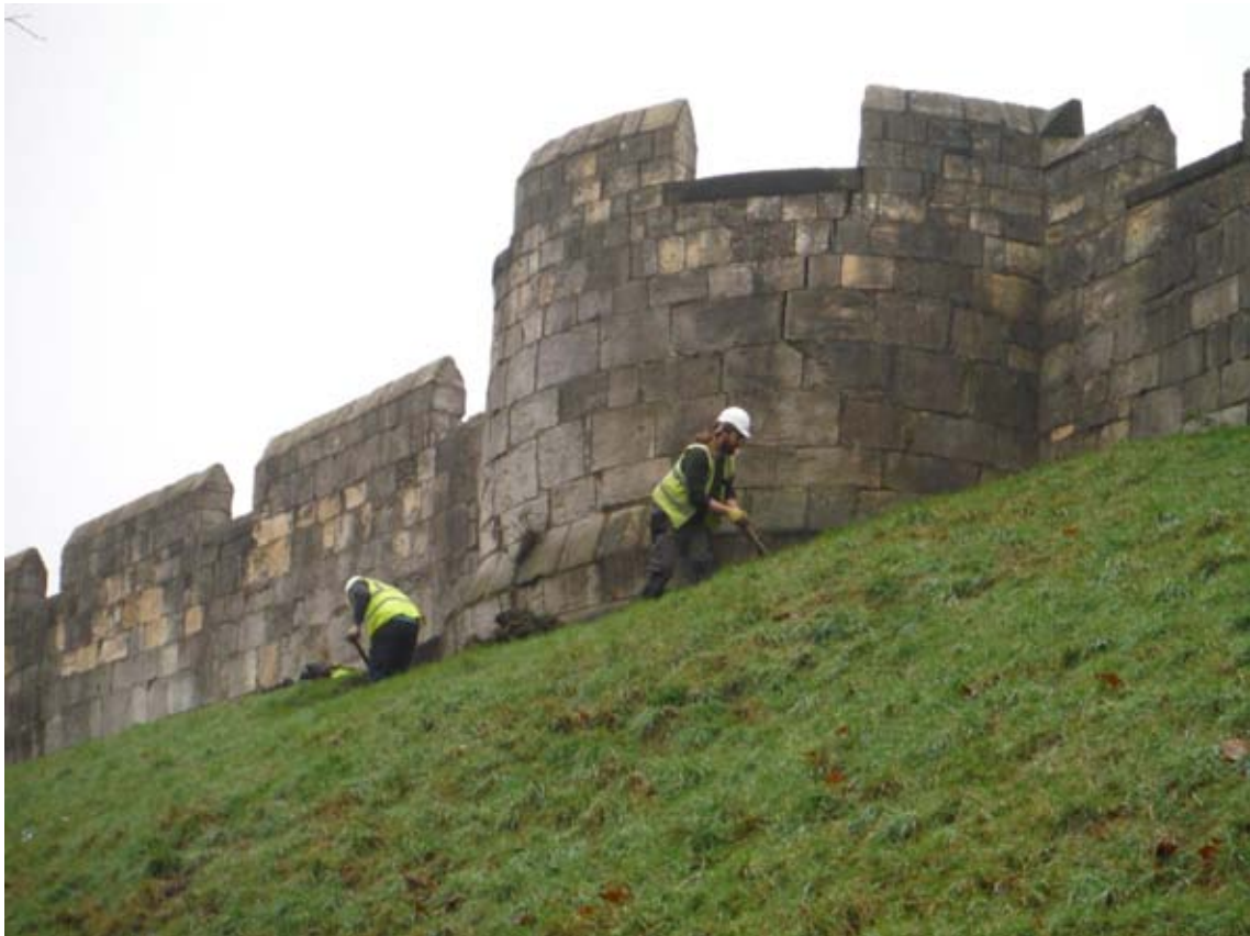
Plate 1. Excavation underway at Tower 2 (facing north-west).
