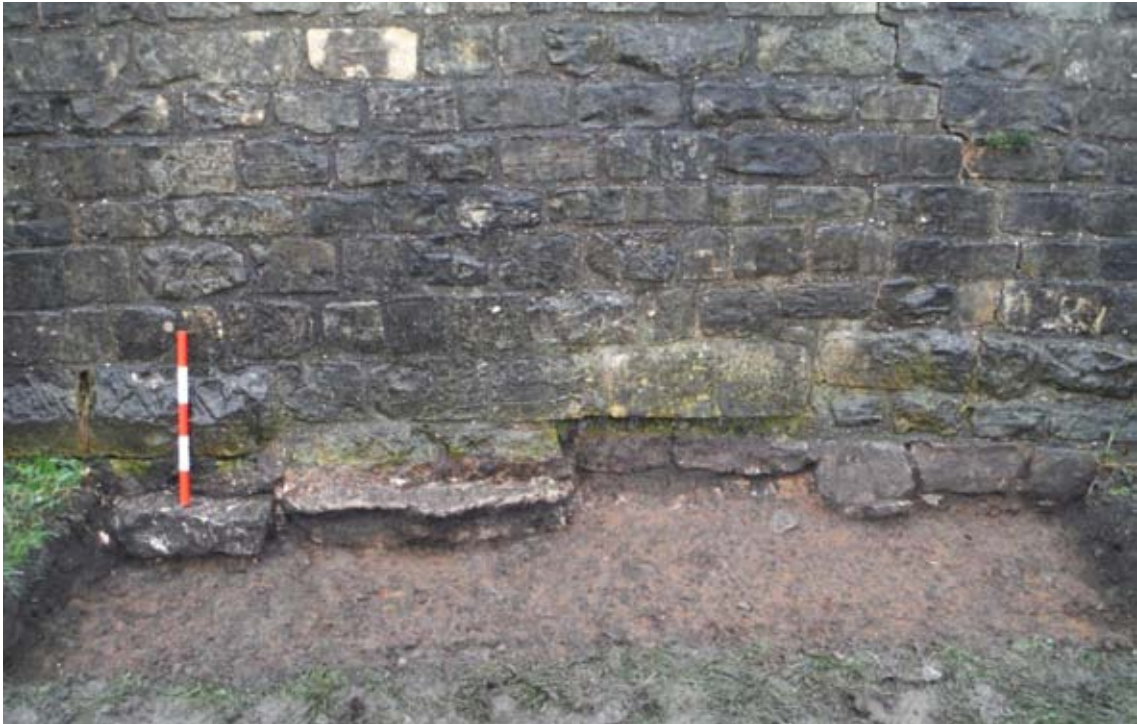
Plate 16. South-east facing view of Section 11, Trial Pit 5 (0.50m scale).
