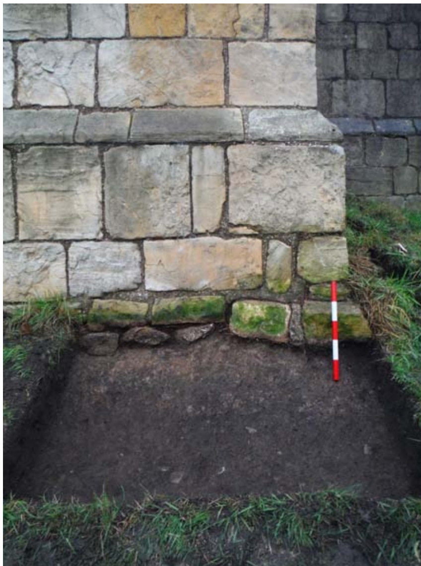
Plate 23. North-west facing view of Section 14, Trial Pit 9 (0.50m scale).
