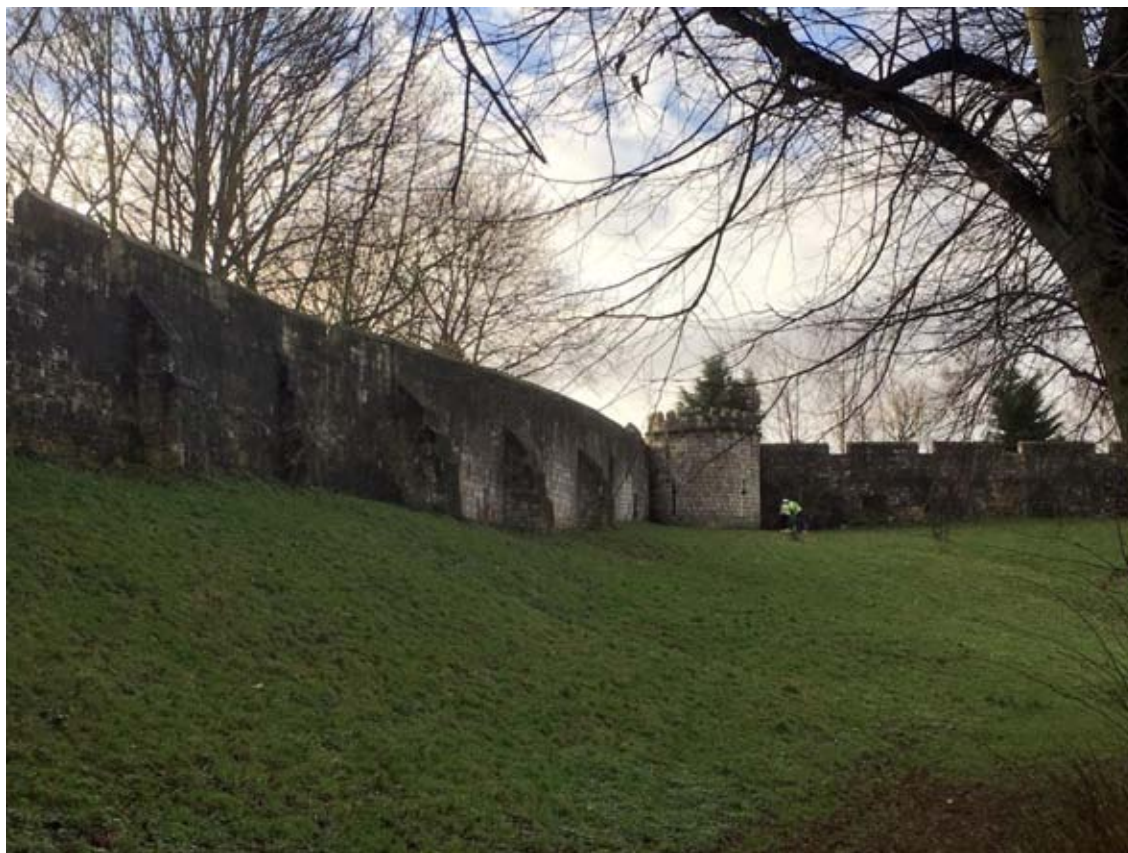
Plate 3. South-west facing view of Tower 32.
