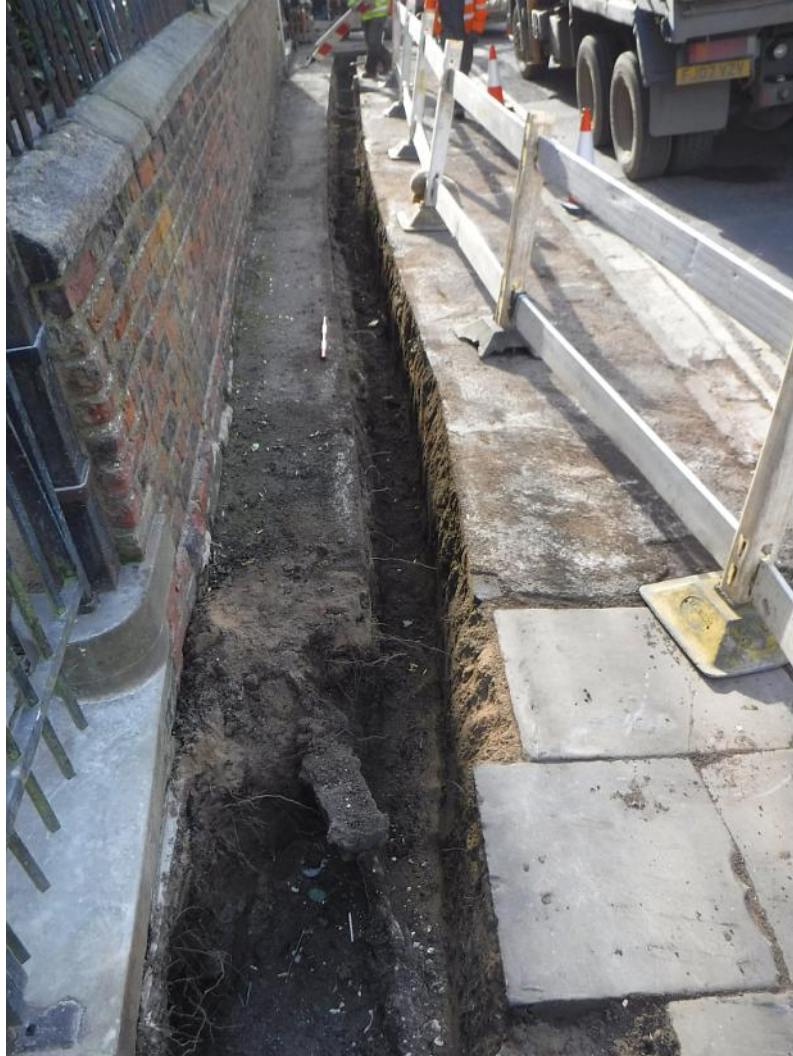
Plate 1 Drain cut along the footpath, facing southwest, scale unit 100mm
