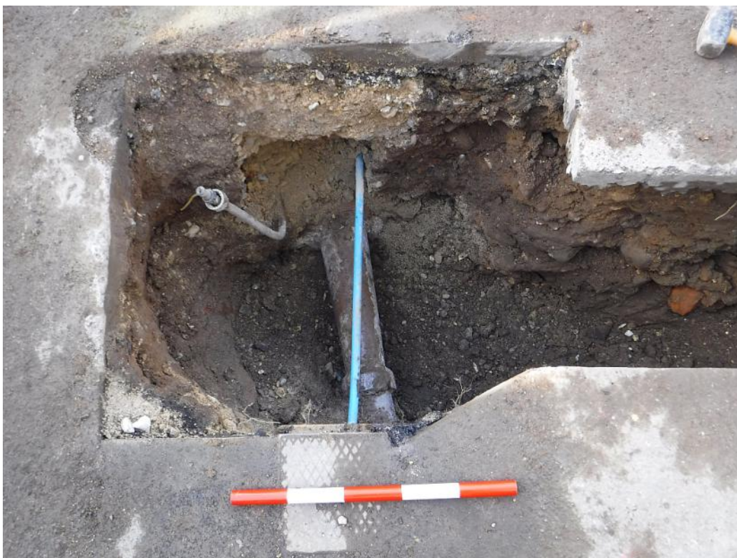
Plate 2 South-western end of drain cut, facing northwest, scale unit 100mm
