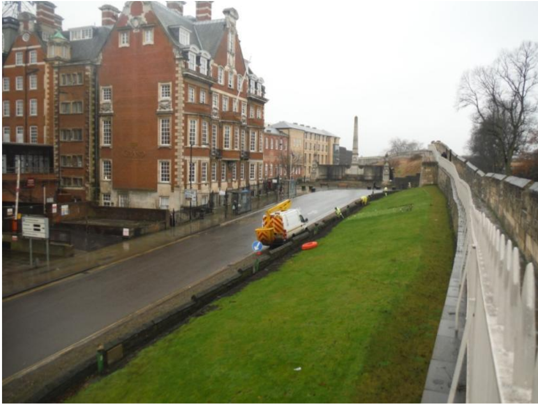
Plate 3. Fuse boxes and lighting plinths visible on the inner wall, facing south-east.
