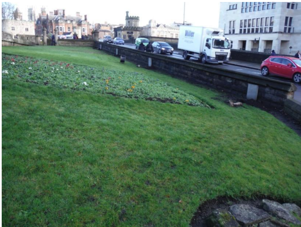
Plate 1. Lighting fuse boxes visible on the wall with the slots excavated in front, facing north-east.
