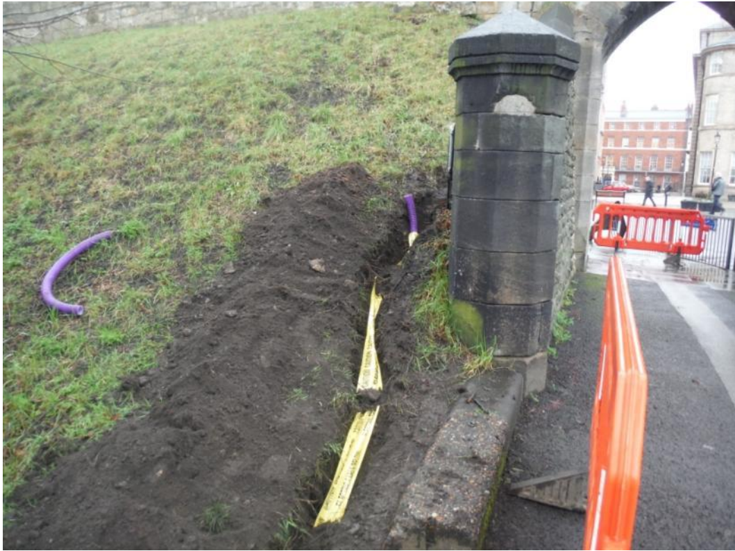
Plate 5. Replacement of ducting and electrical cable. facing east.
