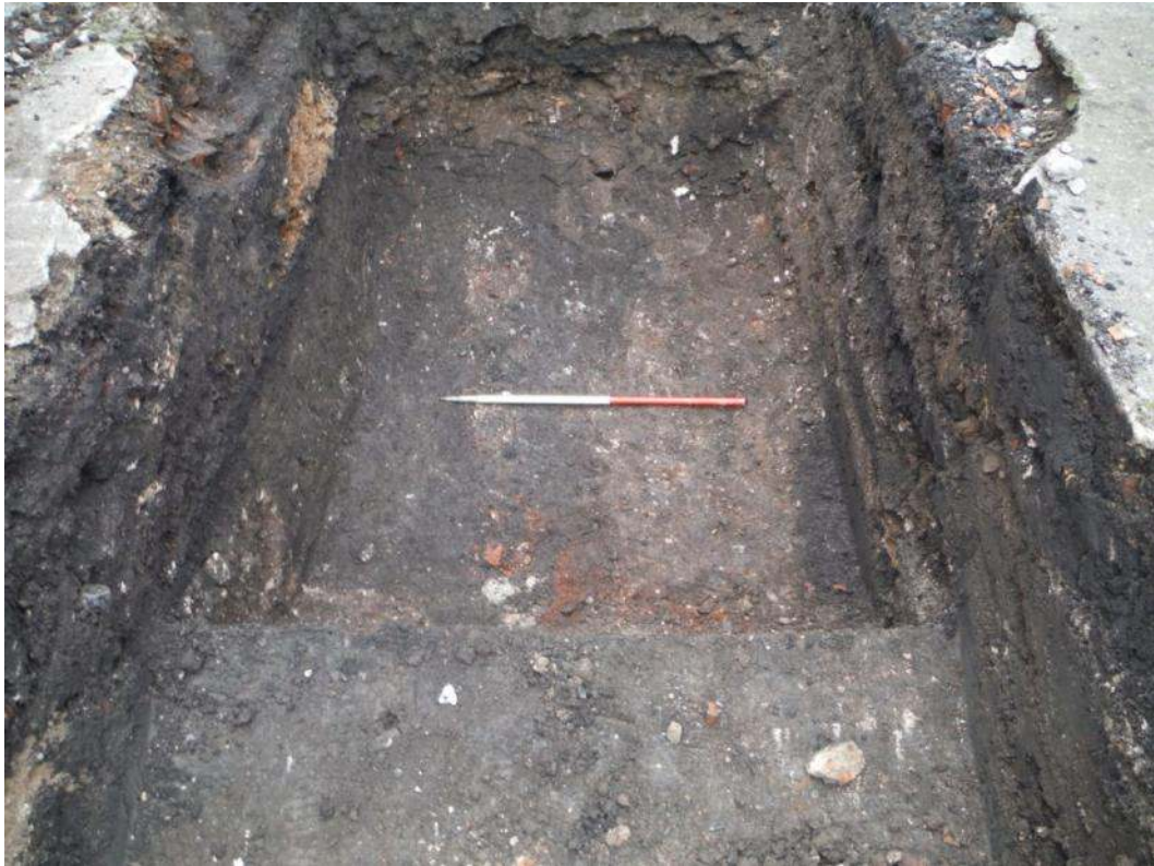
Plate 11: Trench 2, viewed from the north west
