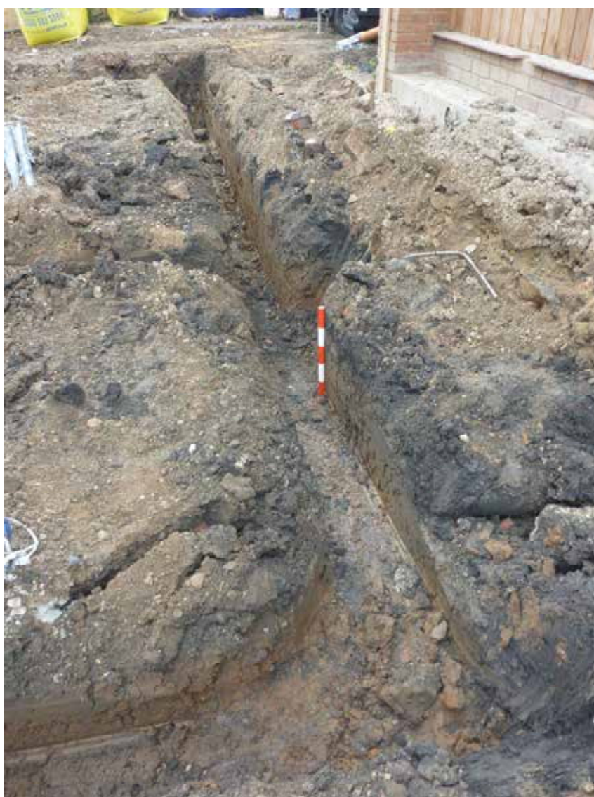
Plate 3: Service trenches viewed from the north-east
