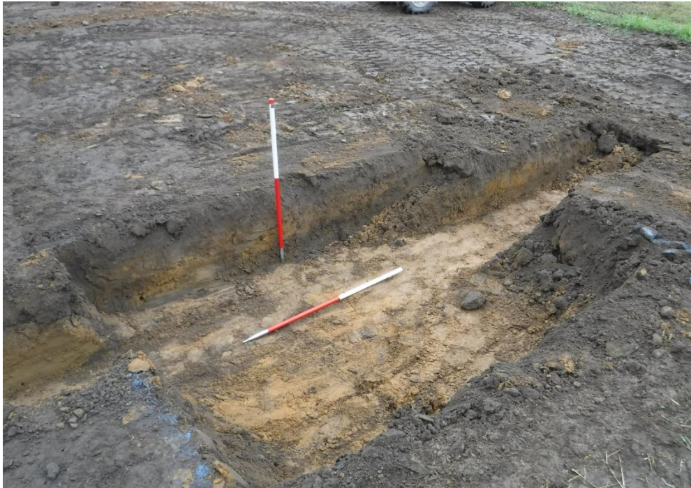
Plate 3. North wall footings for chimney stack looking south-west. Scales: 1m
