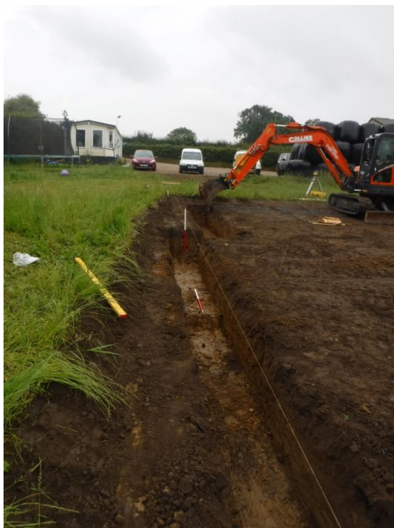
Plate 2. East footing trench, fully excavated, looking south. Scales 1m.
