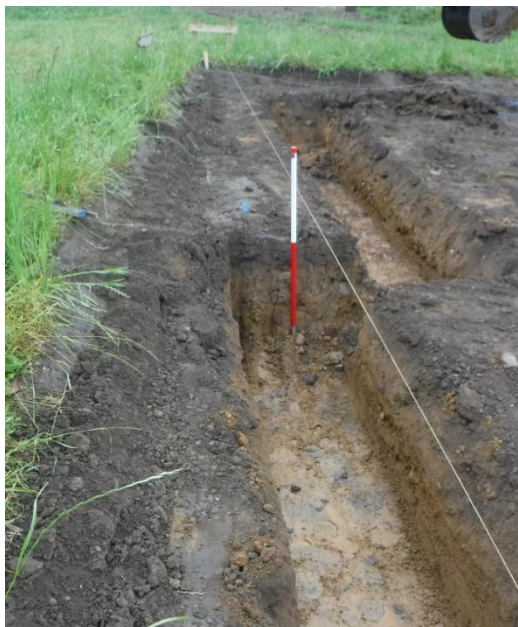
Plate 4. Detail of sequence exposed in east footing trench, looking south. Scale: 1m
