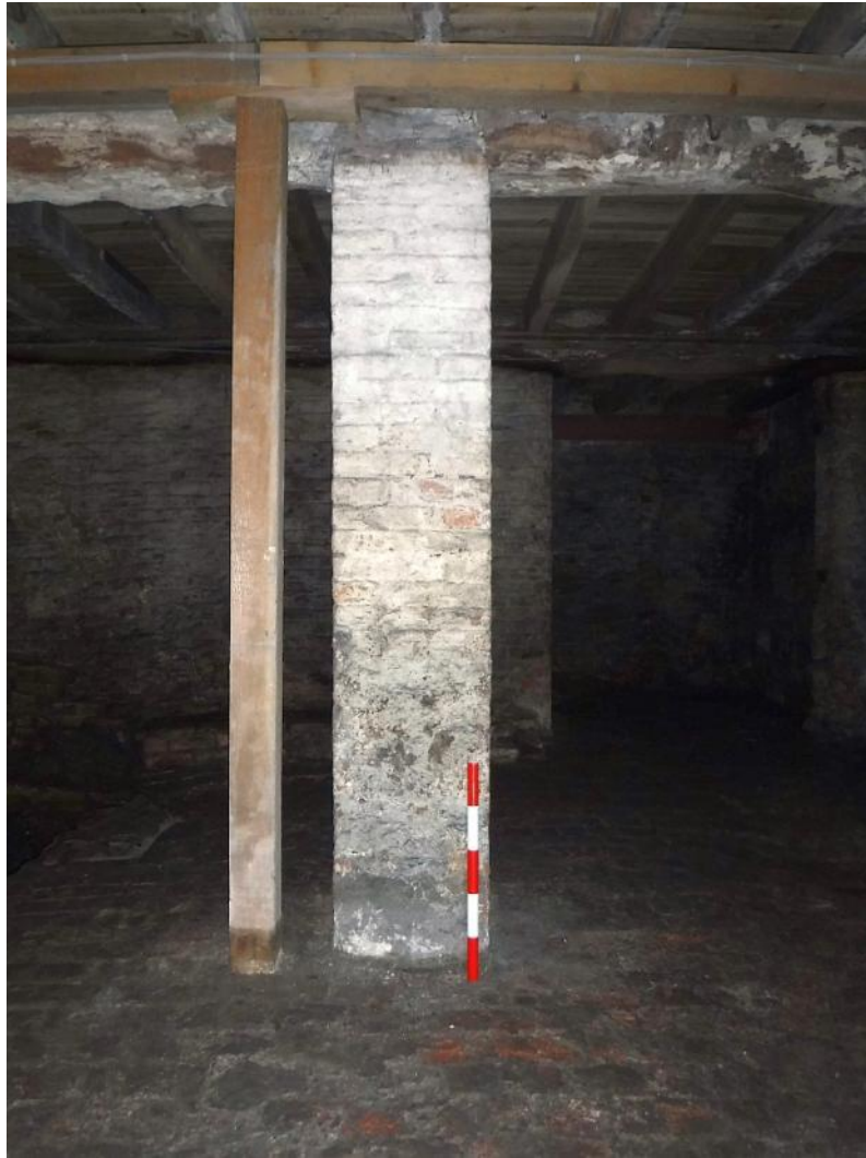
Plate 5 Support column, facing north-east, scale unit 100mm
