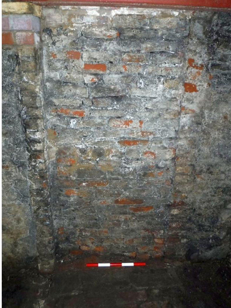
Plate 3 Blocked doorway, facing north-west, scale unit 100mm
