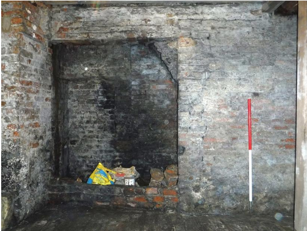
Plate 4 Chimney opening, facing north-west, scale unit 500mm
