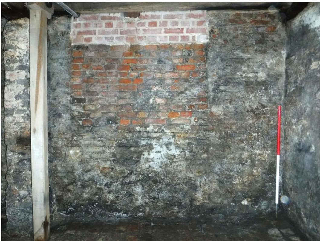
Plate 2 Bay wall and blocked lightwell, facing north-east, scale unit 500mm
