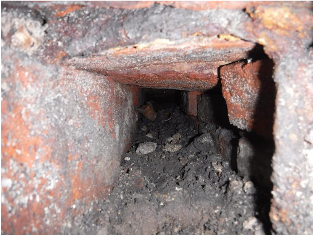
Plate 16 Test pit 3 culvert (internal), facing north-east, scale unit 100mm
