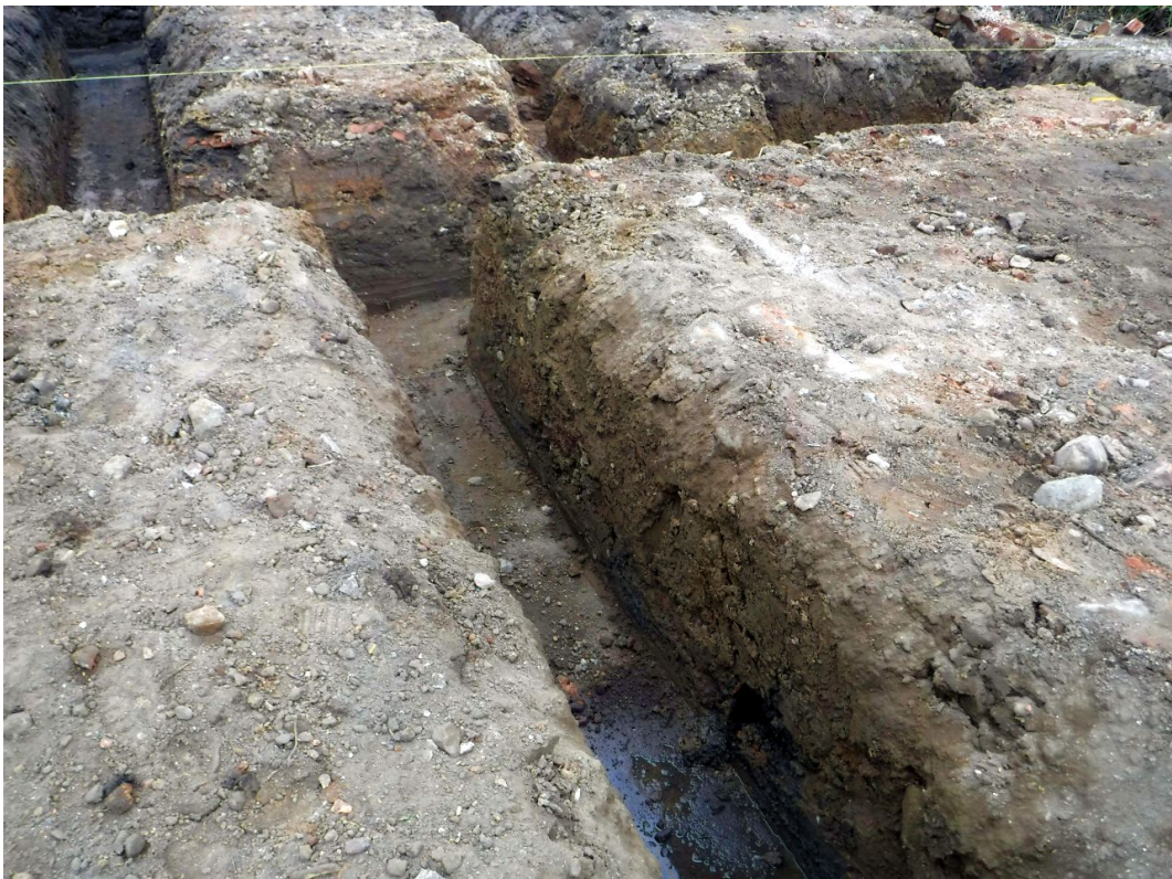
Plate 5 Strip foundations Plot 1, looking north.
