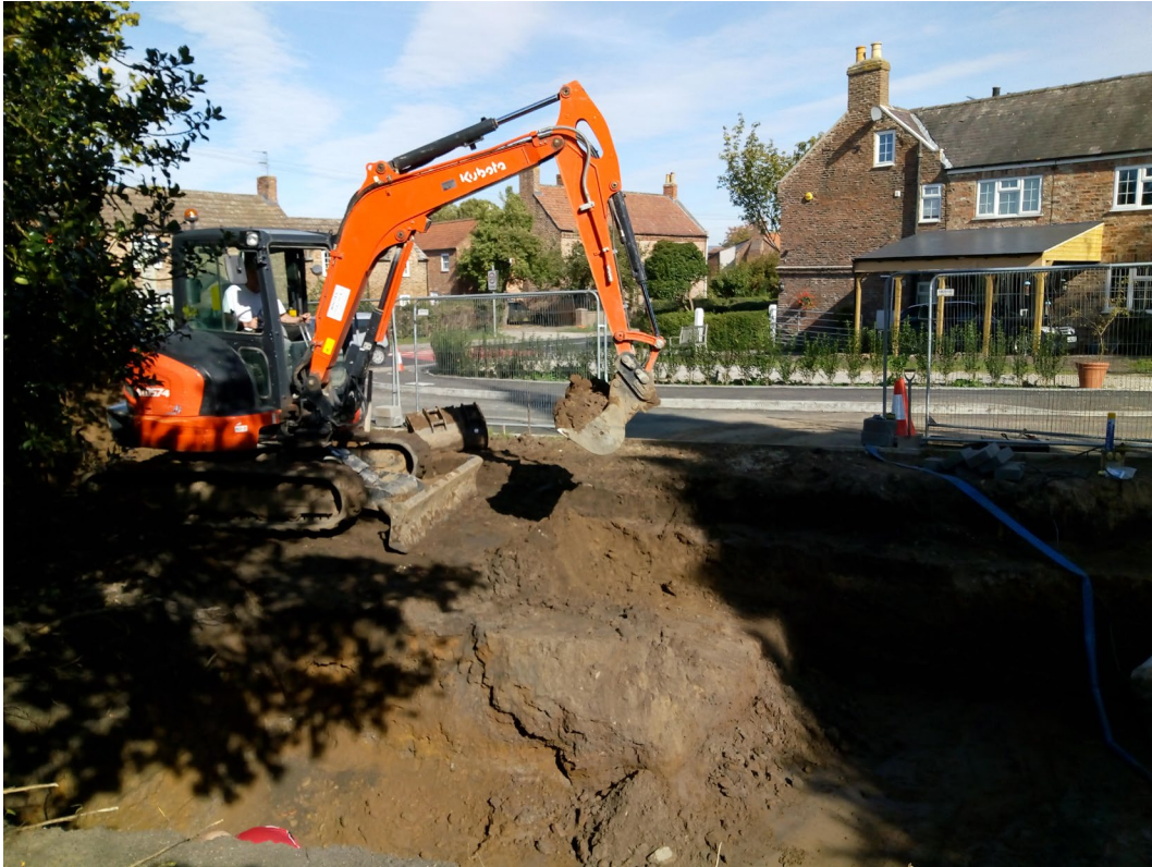
Plate 8 2018 monitoring, looking north-east.
