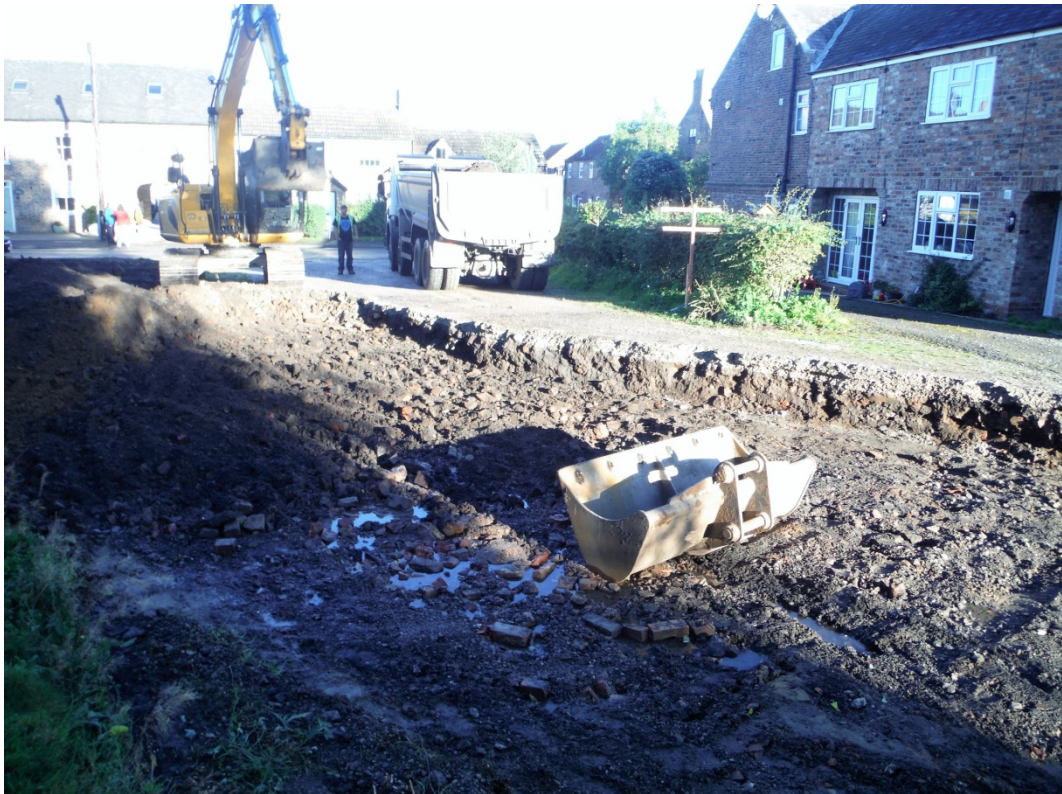
Plate 6 Road strip, looking north-east.
