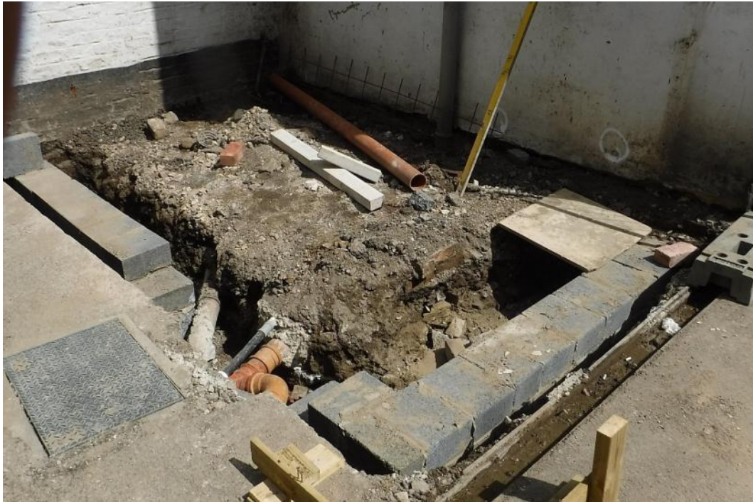
Plate 1 Foundations, facing north
