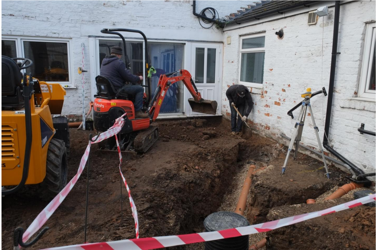
Plate 3 Stripping commences across the footprint of the new building
